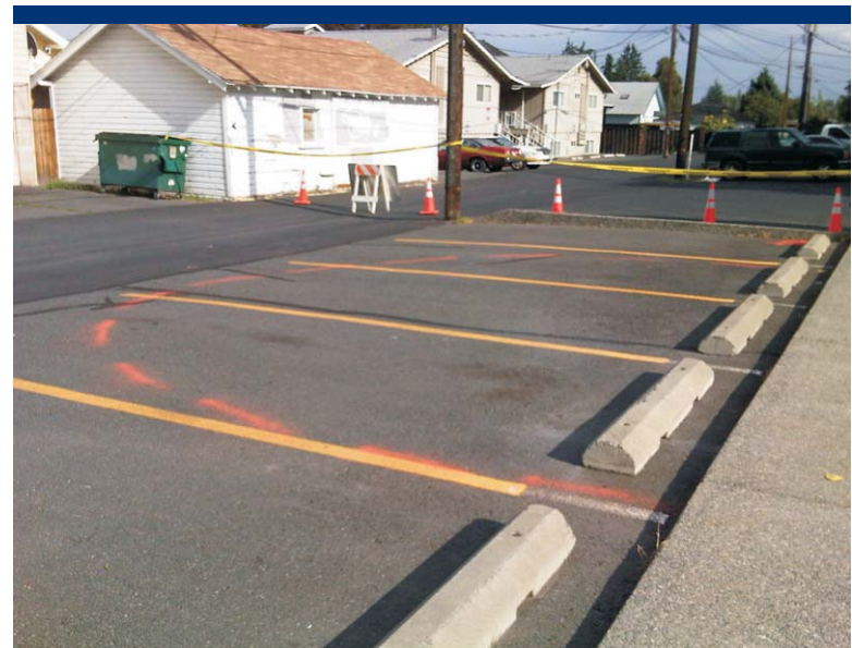
Photo 3 Paint showing area of visible mercury beads in the parking lot.
