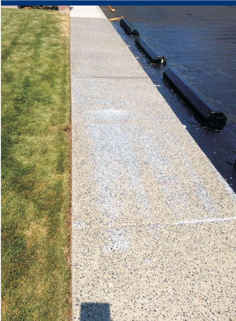
Photo 14 View of the slurry sealant applied to the sidewalk section at the detonation point.
