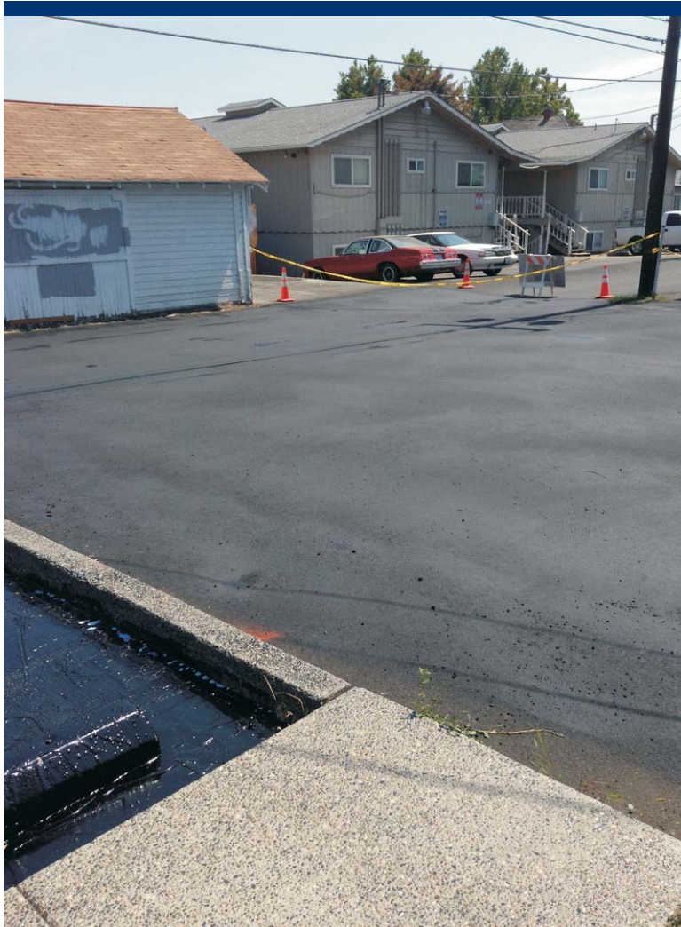
Photo 12 View of the applied cold asphalt sealant on the southern portion of the exclusion zone.
