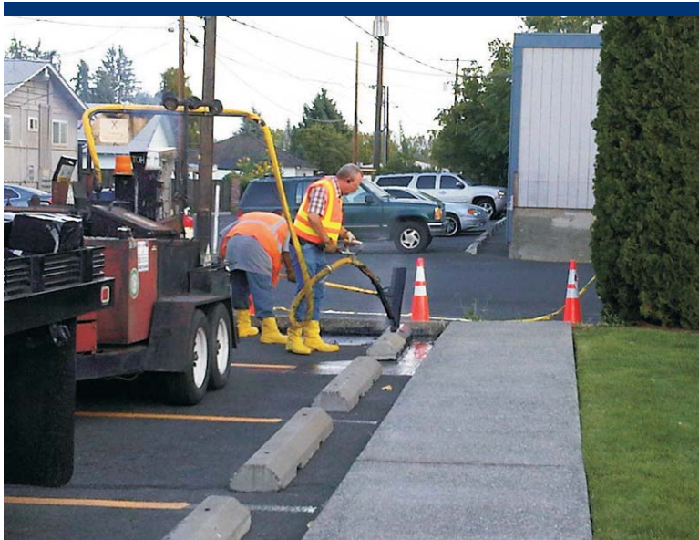
Photo 4 City of Yakima workers applying slurry sealant in parking lot.
