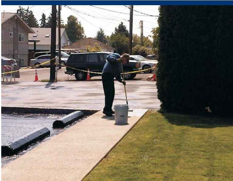
Photo 9 Application of sealant on sidewalk.
