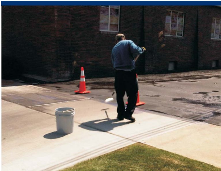
Photo 11 Application of concrete sealant on public sidewalk.
