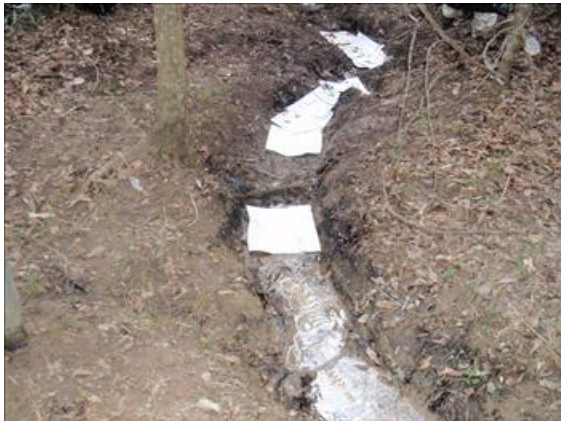
Photo 9: Absorbent Pads
