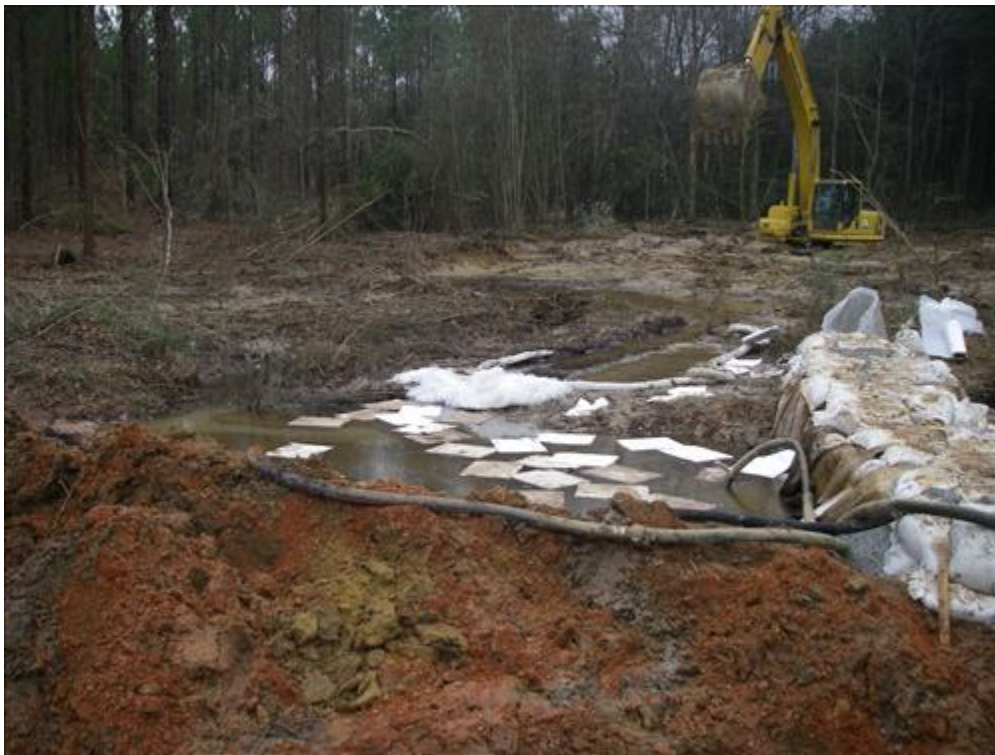
Photo 2: Temporary Underflow Dam
