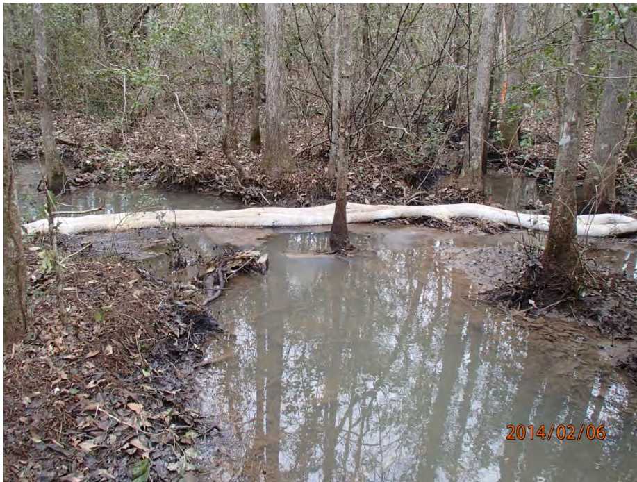
O&M Station D2 – Three sock booms and one snare line before replacement.
