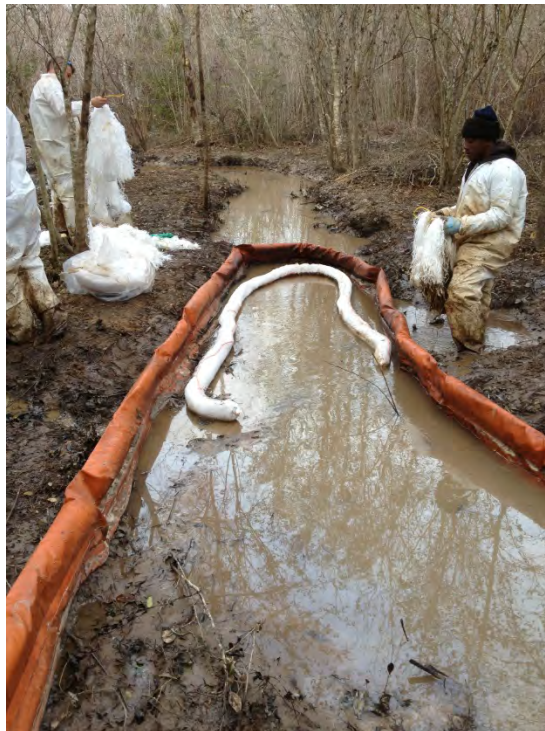
O&M Station C3 – After replacement of sock boom.
