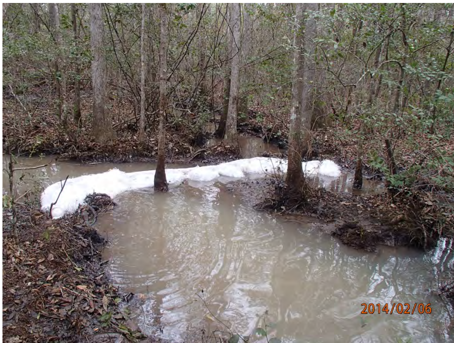
O&M Station D2 – One sock boom and one snare line after replacement.
