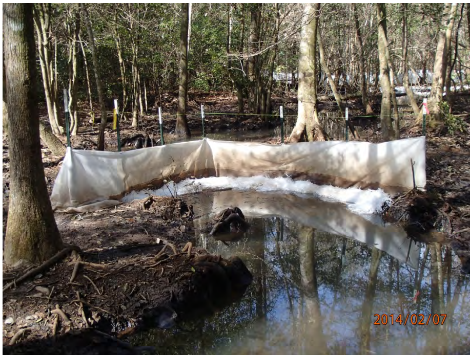
O&M Station E1 – After placement of snare and sock boom.
