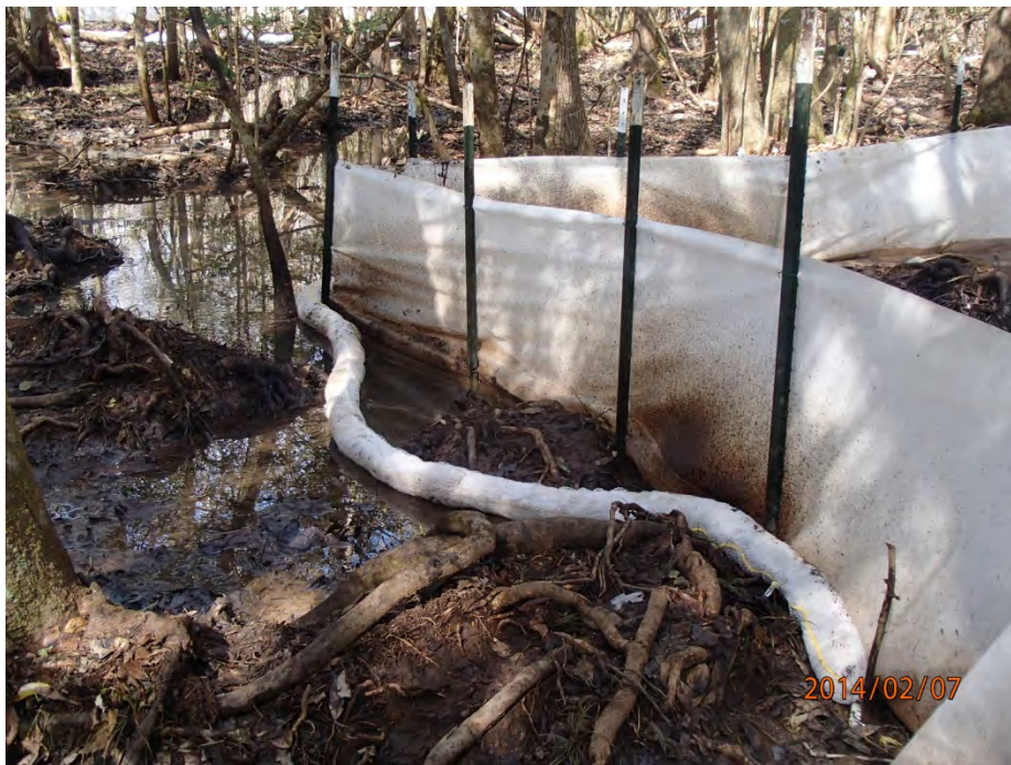
O&M Station E2 – After placement of sock boom.
