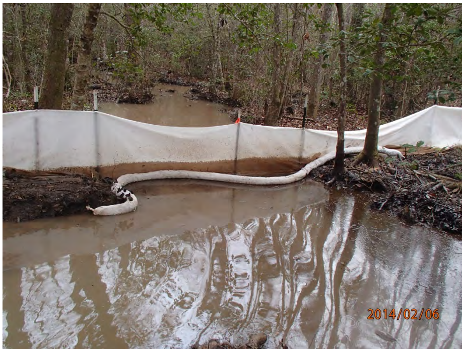
O&M Station D1 – After replacement of sock boom.
