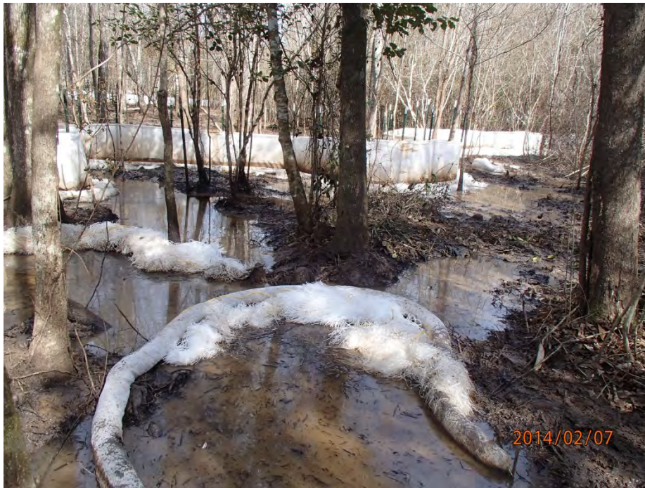
O&M Station B1 – with new sock boom and snare.
