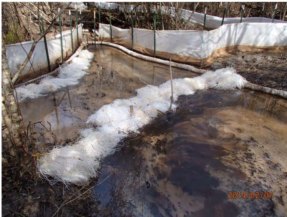
O&M Station B2 – with new sock boom and snare.
