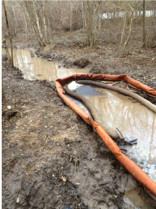
O&M Station C3 – Before replacement of sock boom.
