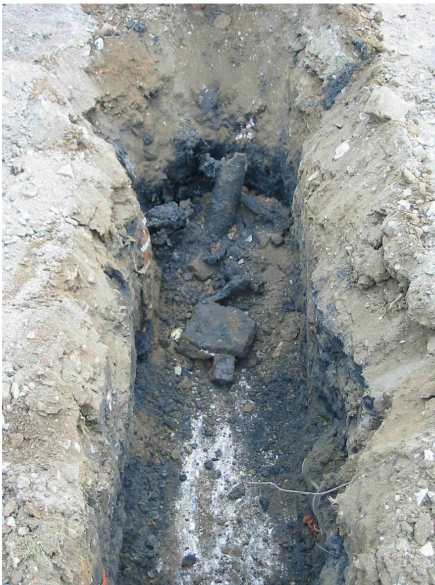
Photo Metro-Trainer.060: View to the northeast of a concrete slab encountered at 4 ft bgs in the Test Trench-02 excavation at the Trainer Industries, LLC/former Metro Container Corporation site. Most of the anthropogenic fill encountered in this trench was comprised of bricks, concrete block, terra-cotta pipe, and miscellaneous metallic debris.
