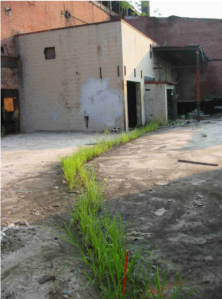
Photo Metro-Trainer.040: View to the northeast of the same area depicted in Photo Metro-Trainer.009, the location of the “open top” drum reclaiming operations, within the confines of the former drum reclaiming building at the Trainer Industries, LLC/former Metro Container Corporation site. The presence of vegetation in the waste conveyance channels makes the trend of this former drainage system very evident. The orange stake in the foreground marks the location of the 05-MET-68 soil boring location.
