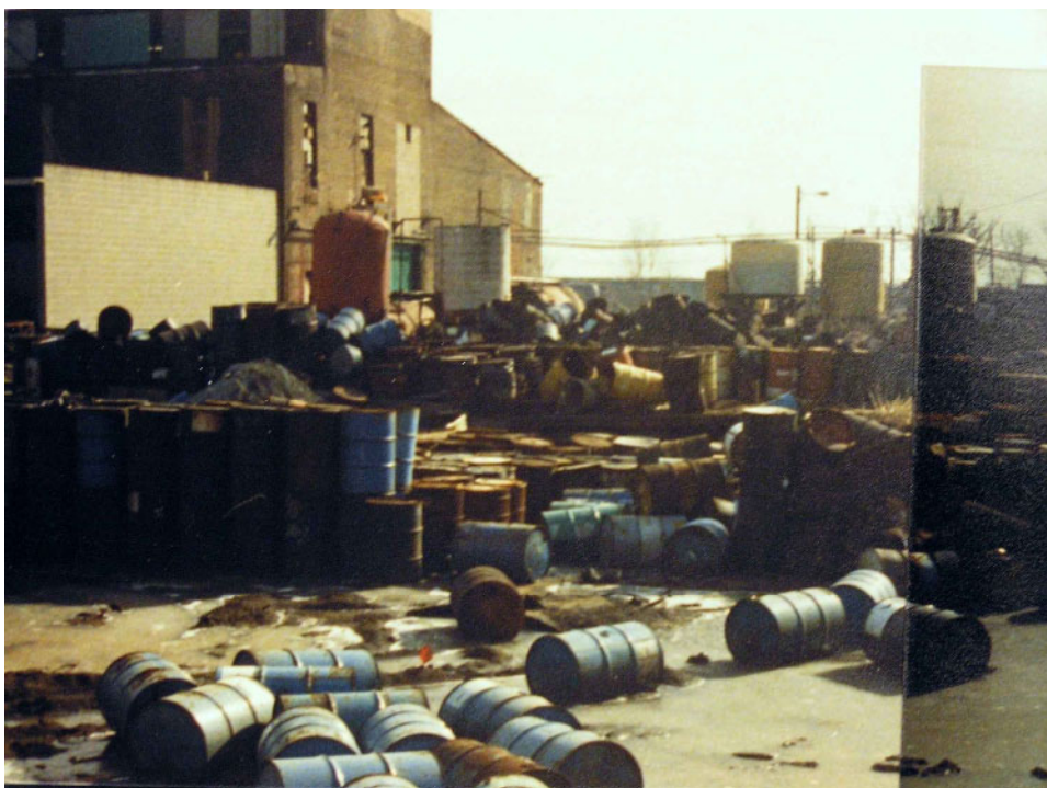
Photo Metro-Trainer.89-13: View to the southeast of the drum reclaiming building (left), formerly the Oven Building under Stauffer Chemical Company, Inc. ownership (1920-1959). Note the hundreds of drums dumped haphazardly through this section of the property, the liquids surrounding the drums, and the Acid Tank Farm (right background), which was used as a de facto waste impoundment by Metro Container Corporation in the late 1980s.
