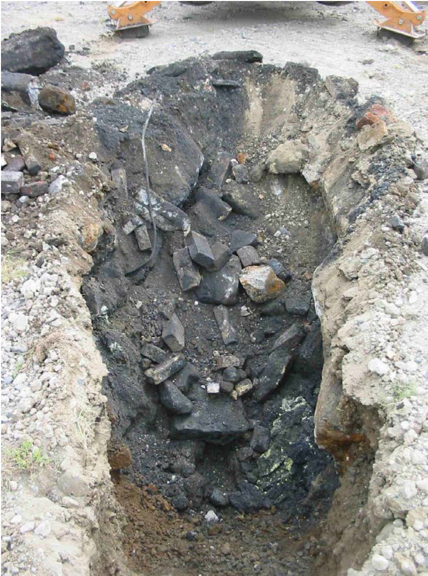
Photo Metro-Trainer.067: View to the southeast of the Test Trench-04 excavation at the Trainer Industries, LLC/former Metro Container Corporation site, in the area depicted at the center of Photo Metro-Trainer.002. This test trench encountered demolition debris, primarily brick and rebar-reinforced concrete, probable remnants of the aboveground storage tank demolition that took place after Stauffer Chemical Company, Inc. ownership when the site was cleared of most of its original tankage.
