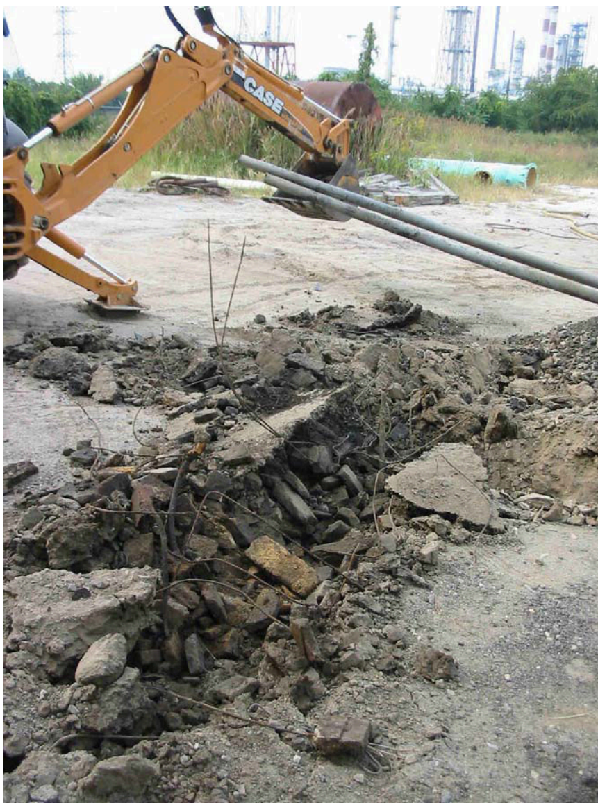
Photo Metro-Trainer.064: View to the west of the Test Trench-03 excavation at the Trainer Industries, LLC/former Metro Container Corporation site. In addition to the aforementioned plastic piping, a significant amount of metallic debris (e.g., wire, conduit), bricks, and cast concrete block was encountered in the excavation.
