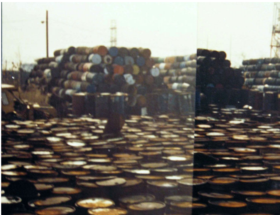
Photo Metro-Trainer.89-18: Close-up view to the south of Photo Metro-Trainer.89-17. Note again the unsecured drum lids that caused sludge to spill out of the drums during precipitation events.
