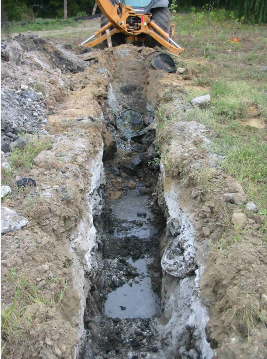
Photo Metro-Trainer.056: View to the northwest of the Test Trench-01 excavation at the Trainer Industries, LLC/former Metro Container Corporation site. This trench was being advanced to the northwest towards the 05-MET-129 Geoprobe ® location from the 05-MET-01 Geoprobe ® location. Hydrocarbon sheens were noted on the water table, due primarily to the severe soil impacts present beneath the water table in this vicinity.
