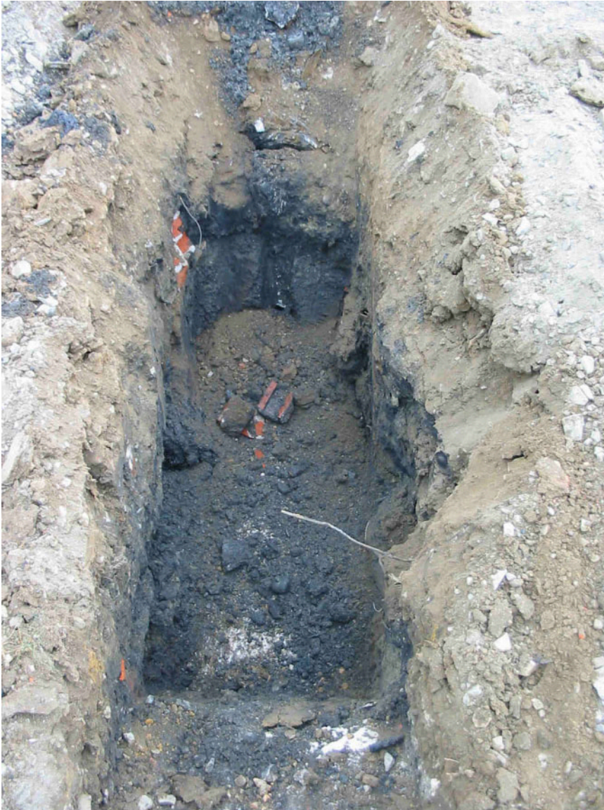
Photo Metro-Trainer.059: View to the northeast of the commencement of the Test Trench-02 excavation at the Trainer Industries, LLC/former Metro Container Corporation site. This trench, which encountered construction debris and a concrete slab, was advanced between the 05-MET-86 and 05-MET-139 Geoprobe ® locations. Historical aerial photographs indicate that this location was the site of a Stauffer Chemical Company, Inc. structure.
