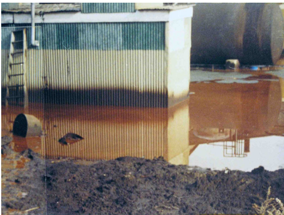
Photo Metro-Trainer.89-24: Close-up view to the northeast of Photo Metro-Trainer.89-22 of the wastewater treatment plant (center) and DAF sludge tank (far right). Some of the most significant impacts to the subsurface discovered in the 2005 Site Characterization were caused by the sludge waste in this unlined impoundment; note the heavy black staining indicating the high level mark on the primary wastewater treatment plant shed (center).
