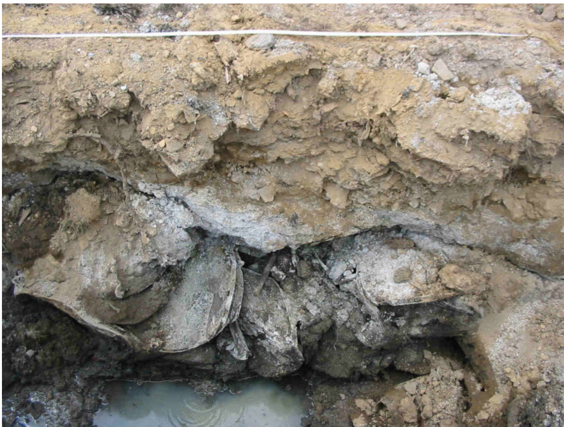
Photo Metro-Trainer.054: View to the southwest of the sidewall of the Test Trench-01 excavation at the Trainer Industries, LLC/former Metro Container Corporation site. Underlying a 2-foot thick layer of soil cover, a distinct light gray layer of flyash was encountered. Underlying this flyash layer was a tightly compacted deposit of crushed and apparently incinerated drums at a depth of 3 to 5 feet bgs.
