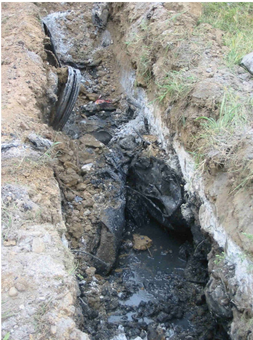
Photo Metro-Trainer.053: View to the northwest of the Test Trench-01 excavation at the Trainer Industries, LLC/former Metro Container Corporation site. This photograph shows the trench being excavated through the top of the water table; additional drum lids were encountered at this depth in addition to numerous crushed 55-gallon drums.
