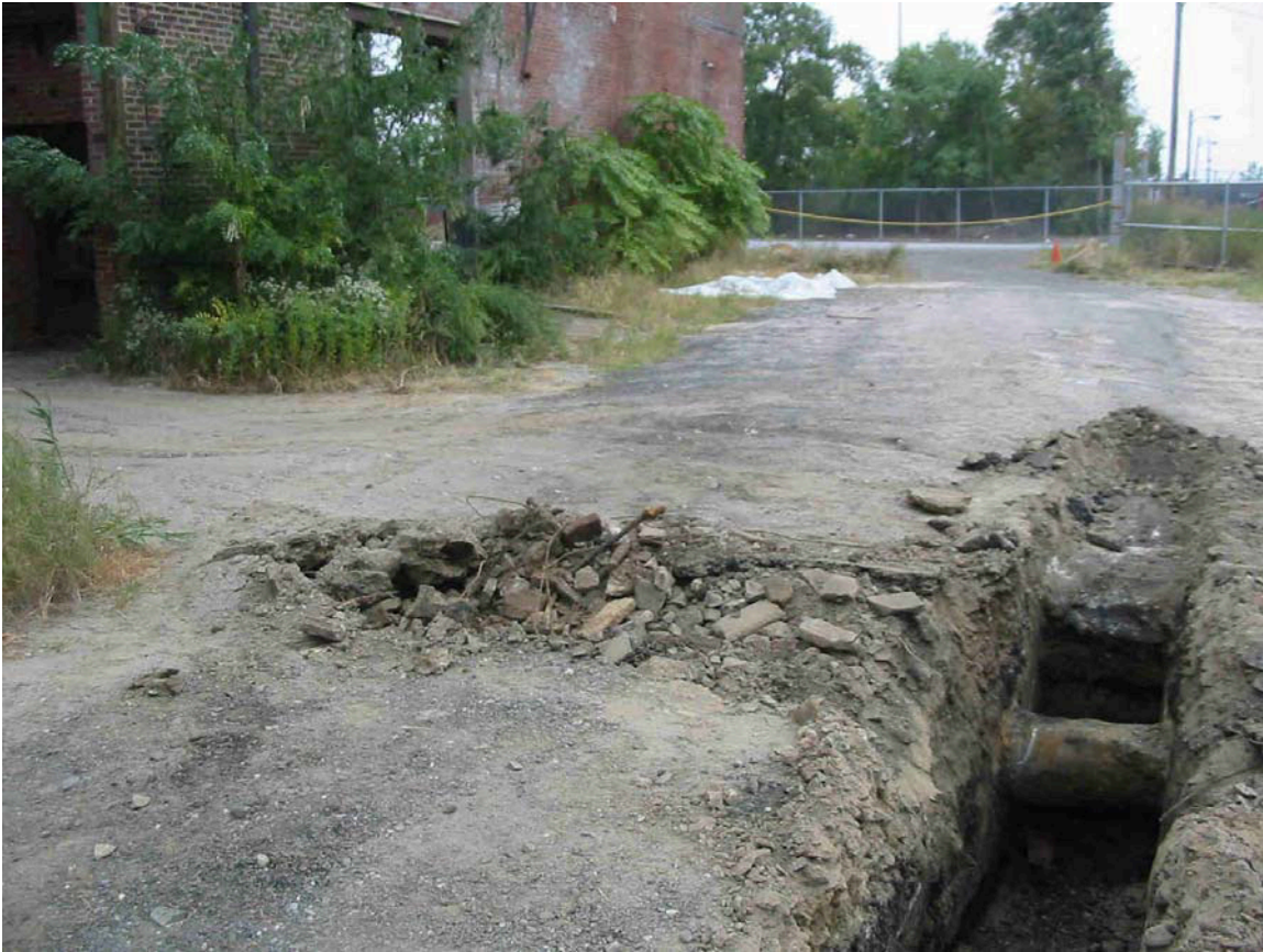
Photo Metro-Trainer.066: View to the southeast of the Test Trench-03 excavation at the Trainer Industries, LLC/former Metro Container Corporation site, showing the orientation of the 15-inch diameter steel pipeline, which may have been the discharge pipe to the former disposal lagoon. It is surmised that when this pipe became inoperable upon closure of the former disposal lagoon, the two plastic pipes seen in Photo Metro-Trainer.063 were installed as part of the primary wastewater treatment system that operated under the former Universal Container Corporation/Metro Container Corporation ownership after 1972.
