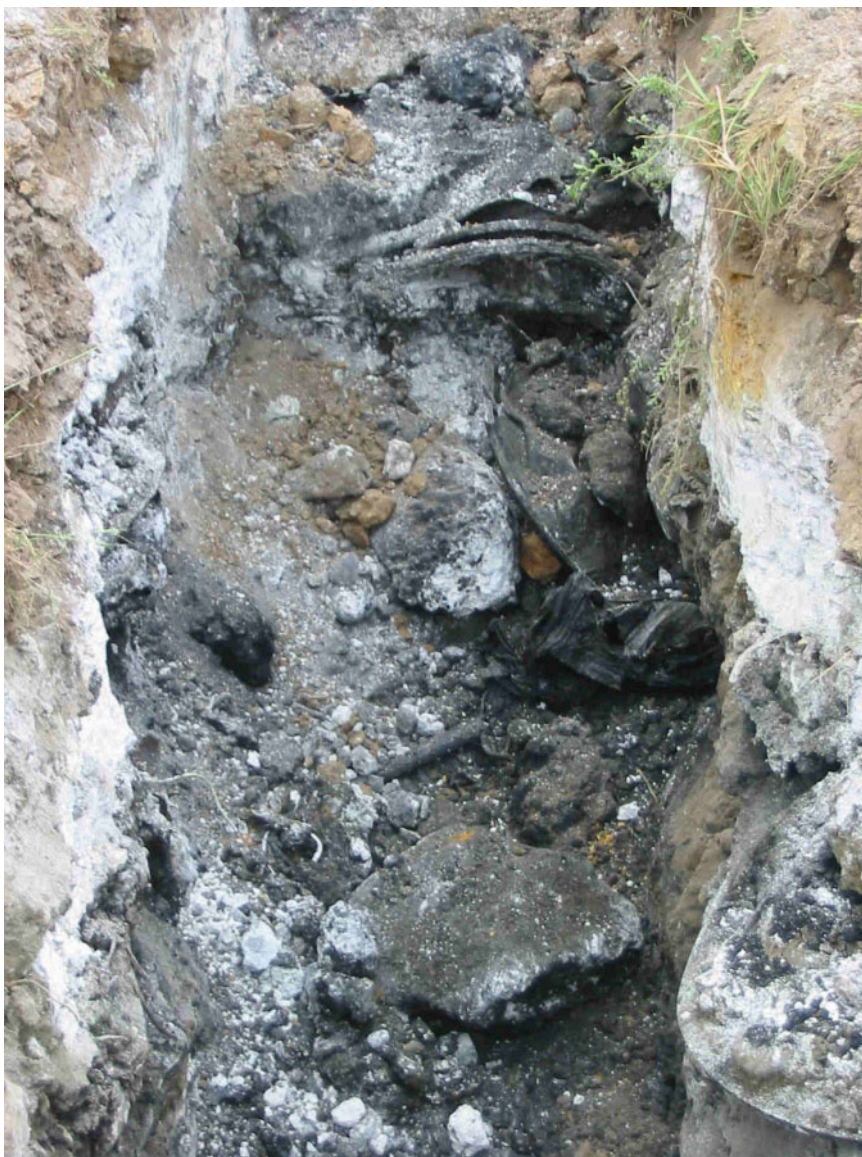
Photo Metro-Trainer.052: View to the northwest of the Test Trench-01 excavation at the Trainer Industries, LLC/former Metro Container Corporation site. This photograph shows the trench had been excavated to a depth just above the water table and that numerous drum lids were encountered at approximately 3 ft bgs.
