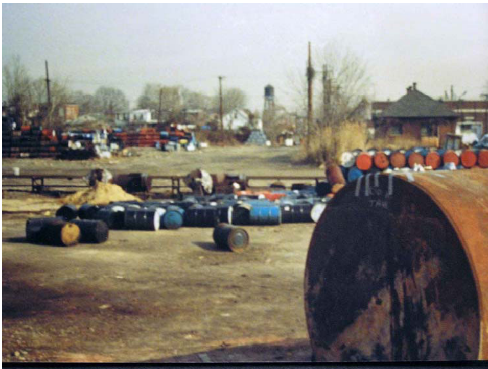
Photo Metro-Trainer.89-03: View to the northeast of the Metro Container Corporation locker room and office (far right background), stockpiled drums (far left background), a discarded tank (right foreground), and a portion of the conveyor system (center) that was used to carry the drums into the drum reconditioning building (far right, not pictured).
