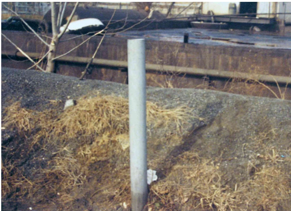
Photo Metro-Trainer.89-10: View to the northwest of the former MW-5 monitoring well (foreground) and the concrete holding tank and secondary containment (background). One of the concrete holding tank circular sumps and one of the tank pump houses are visible in the upper right-hand corner of the photograph.
