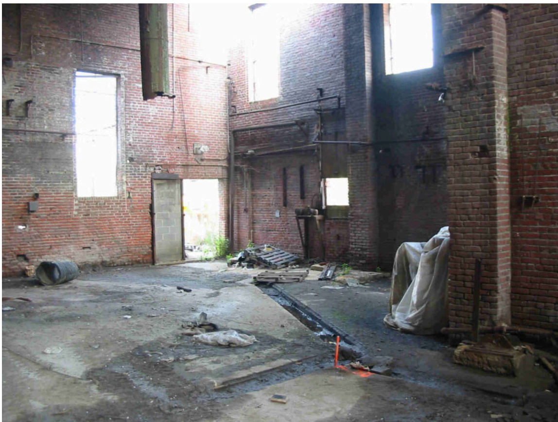
Photo Metro-Trainer.041: View to the west of the same former boiler room depicted in Photo Metro-Trainer.014 within the confines of the former drum reclaiming building at the Trainer Industries, LLC/former Metro Container Corporation site. The orange stake in the foreground marks the location of the 05-MET-58 soil boring location at the intersection of several floor channels that conveyed waste and other materials during the drum reclaiming operations conducted on the site between 1963-1988.
