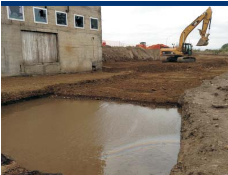
Photo 31 Clean backfill is delivered in two separate lifts that are each compacted.
