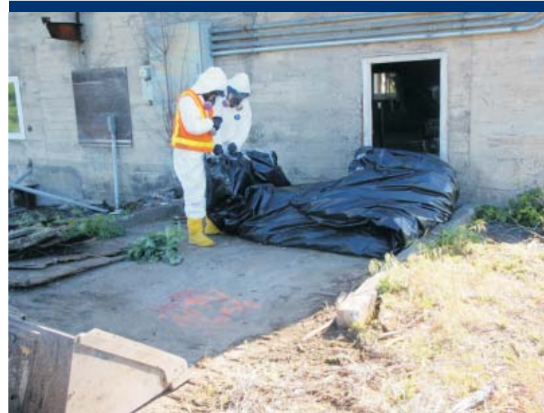
Photo 6 ERRS asbestos-trained workers double-wrapping CAB.
