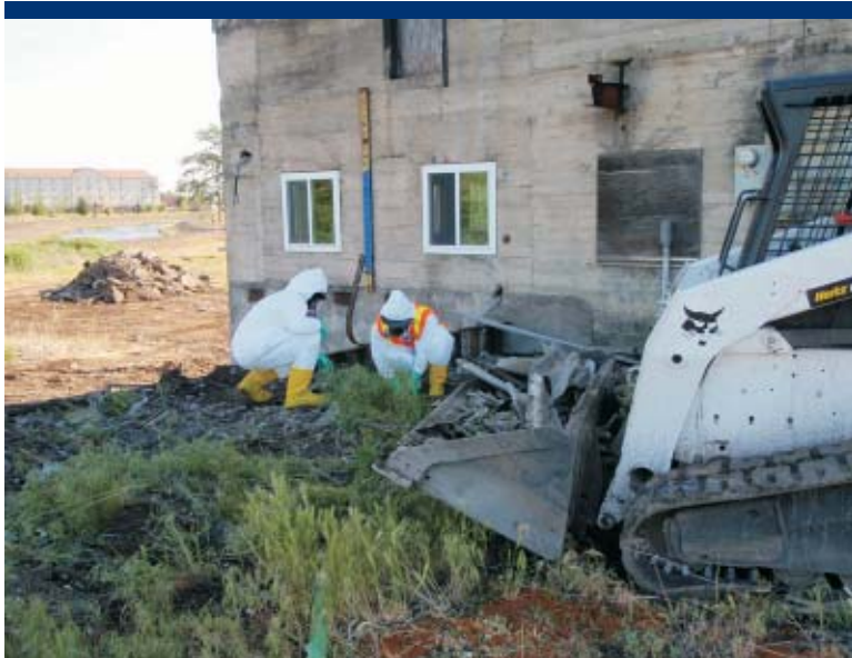
Photo 5 ERRS asbestos-trained workers placing CAB in plastic bags.
