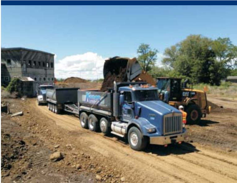
Photo 41 Loading a haul truck with excavated soil.
