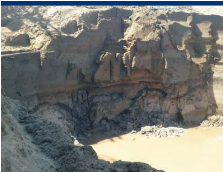
Photo 63 Exposed sidewall (approximately 14 feet high) with PCB contaminated soil located near the groundwater.
