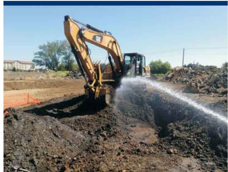
Photo 56 Dust suppression during excavation in the southeastern lobe.
