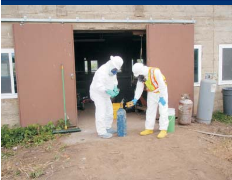
Photo 65 Venting the abandoned propane cylinders and air monitoring with a MultiRae photo-ionization detector.
