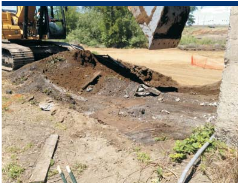
Photo 75 Excavating the southern lobe and discovering the lead-contaminated soil.
