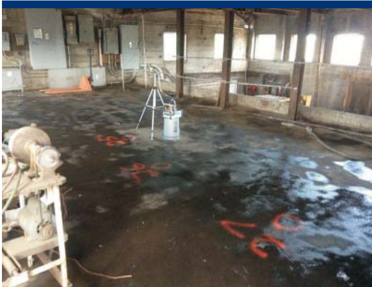
Photo 93 Treatment of main floor of shop building with Lead Safe binding agent after gross decontamination.
