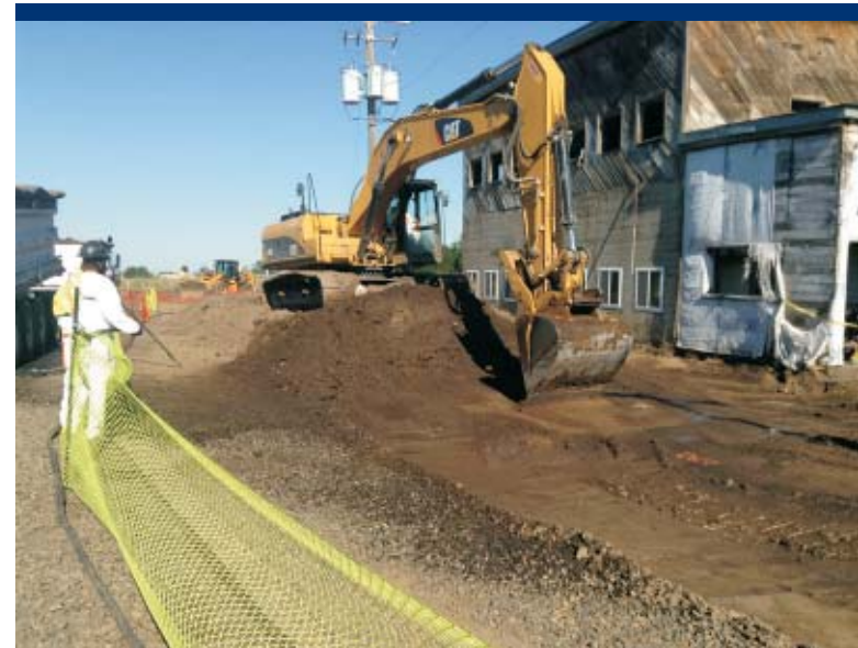
Photo 80 Excavating lead-contaminated soil from the Upland Area in OU1.
