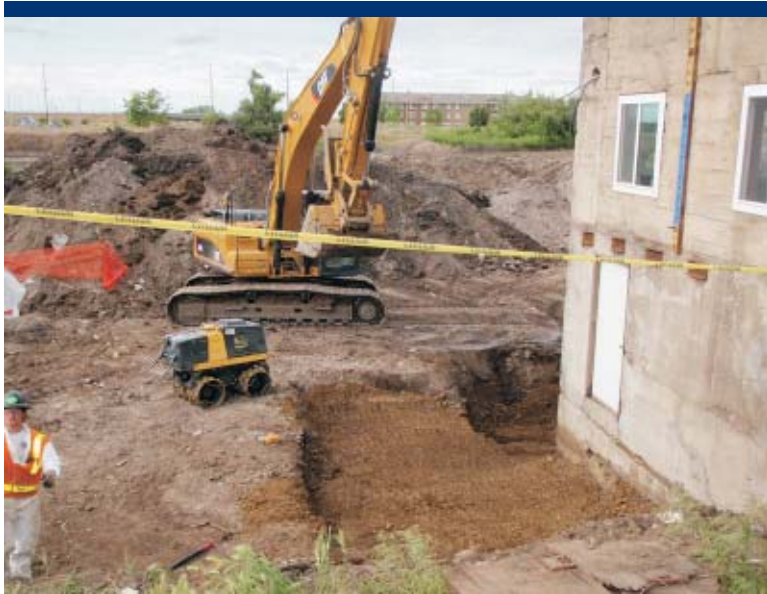
Photo 25 Compacted backfill along the shop building foundation.
