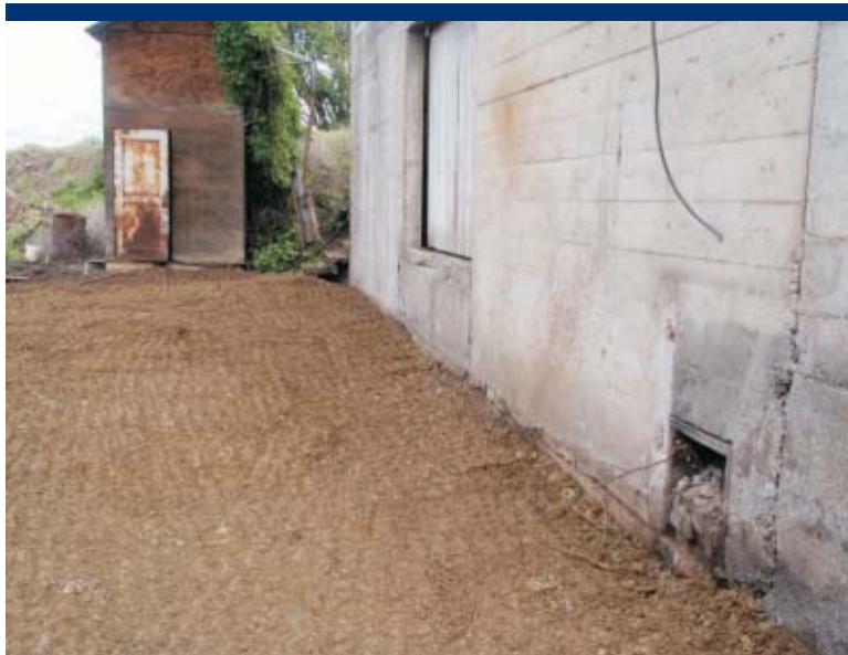
Photo 27 Compacted backfill along the north side of the shop building foundation.
