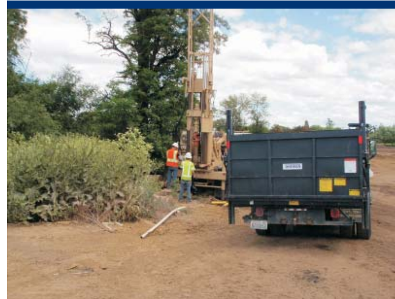
Photo 66 Abandoning MW2 near the swale.
