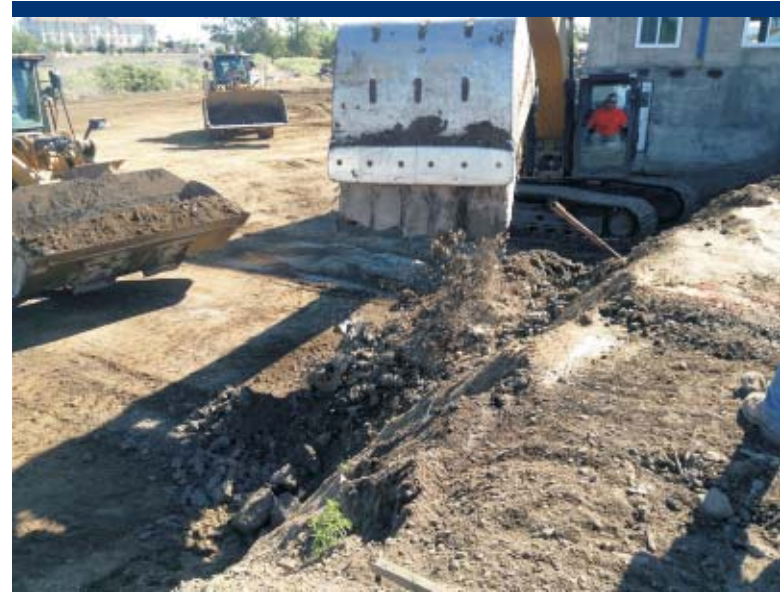
Photo 62 Excavating near former retaining wall to access PCB contaminated soil located near the groundwater.
