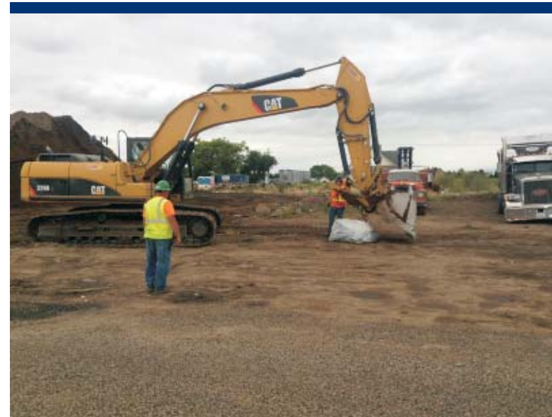
Photo 72 Preparing to load the double-wrapped CAB in a truck for transportation and off-site disposal.
