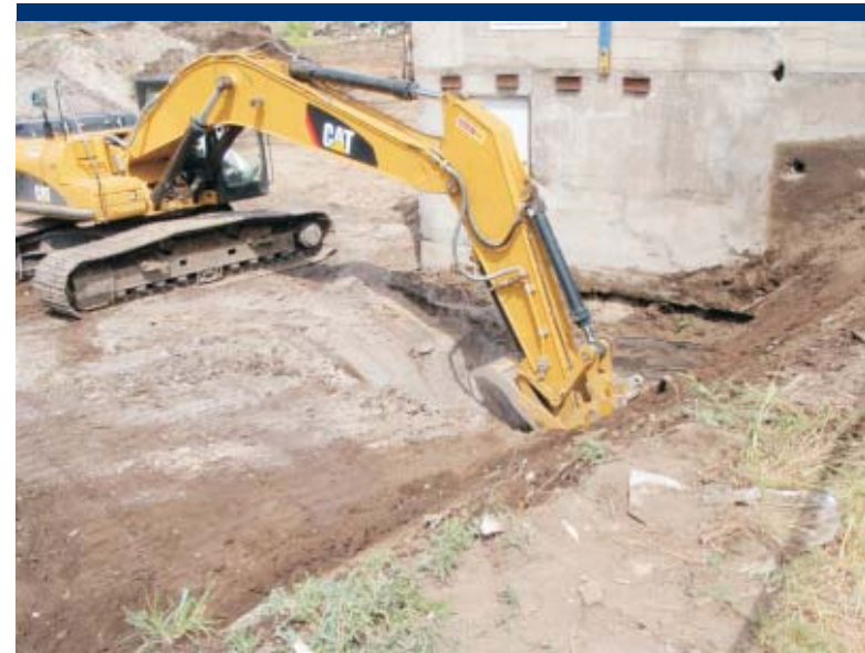
Photo 24 Excavating along the shop building foundation near the former location of the retaining wall.
