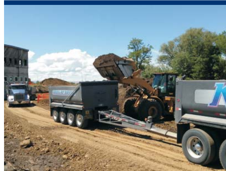
Photo 42 Loading a pup with excavated soil.
