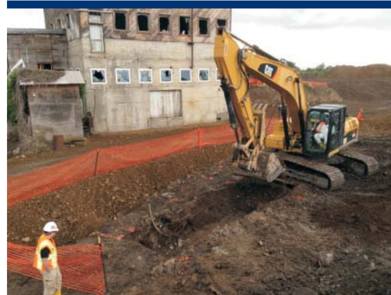
Photo 38 Excavating lead-contaminated soil from the Process Area.
