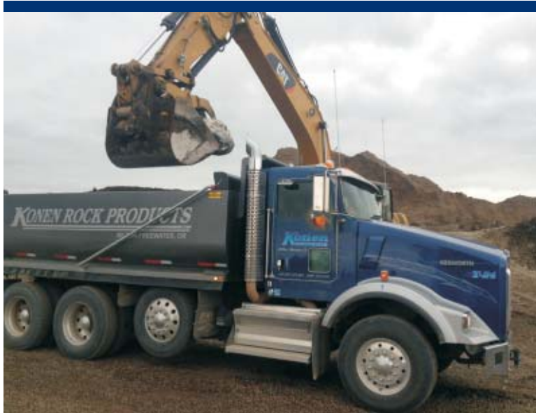
Photo 73 Loading the double-wrapped CAB in a truck for transportation and off-site disposal.
