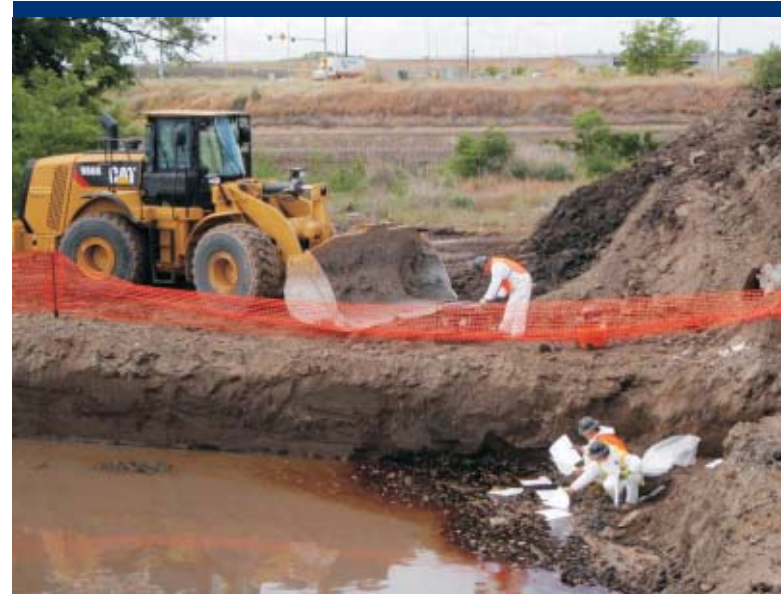
Photo 18 Deploying absorbent pads in the heavy oil.
