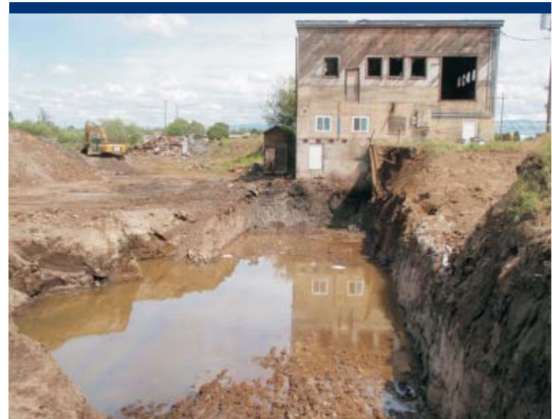
Photo 16 Excavated area near the southwest corner of the SPA with shallow seeping groundwater.
