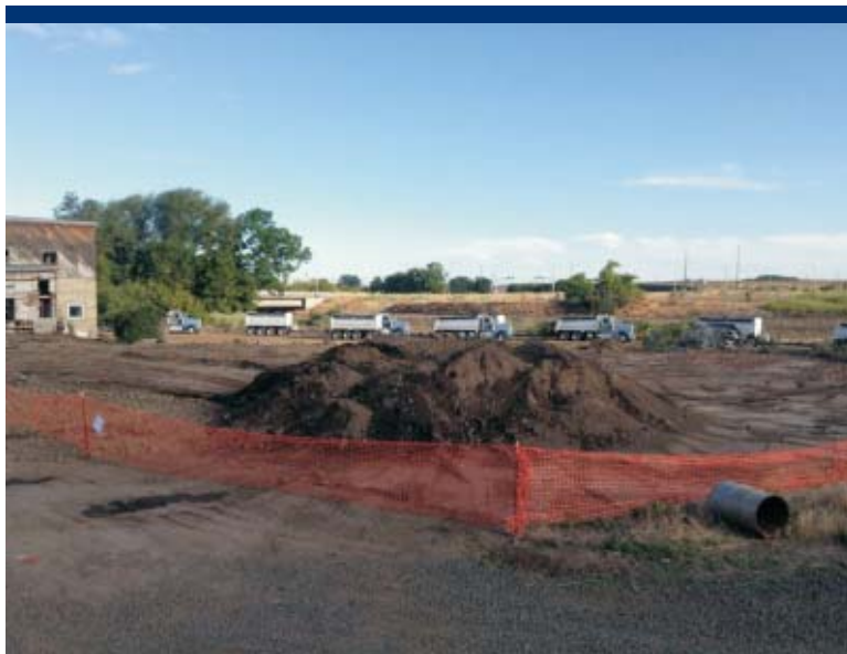
Photo 95 Stockpile of OU3 in foreground; convoy of trucks waiting to receive lead-contaminated soil in the background.
