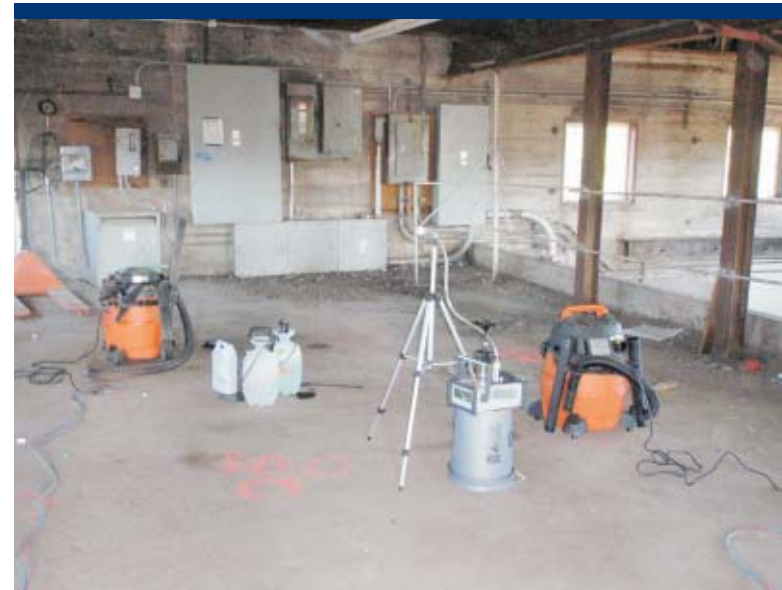
Photo 92 Air monitoring and sampling equipment deployed before gross decontamination of main floor.
