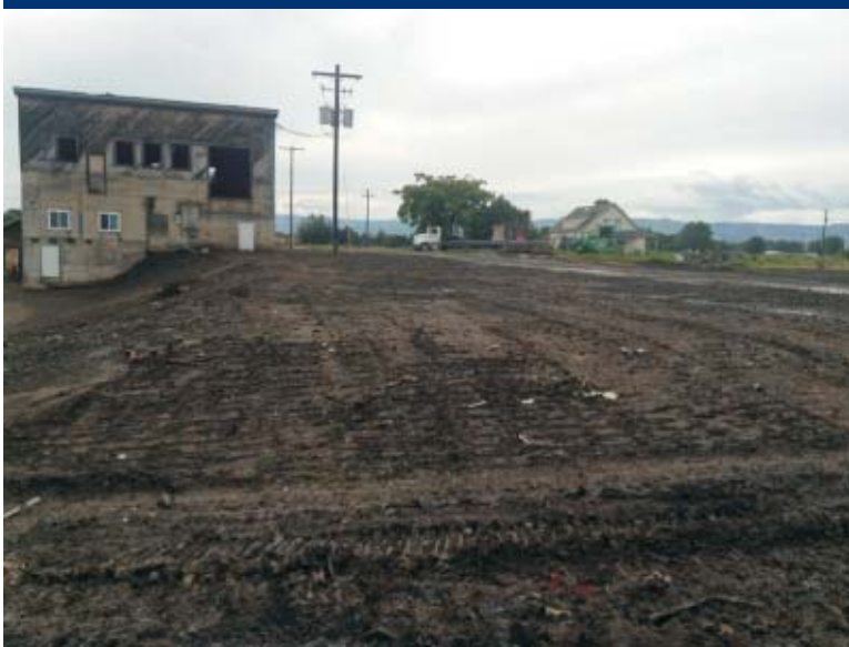
Photo 101 View of the western section of the Upland Area after compaction of backfill.
