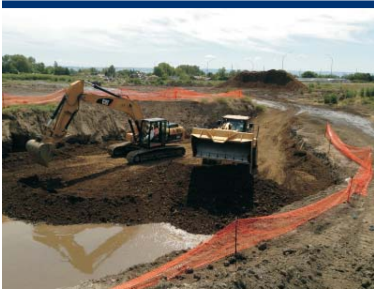
Photo 29 Placing clean backfill in the exposed excavation in the SPA.
