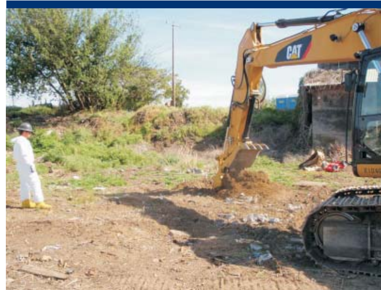
Photo 10 Installing eastern test pit (SP01) along the boundary of the SPA and NPA.
