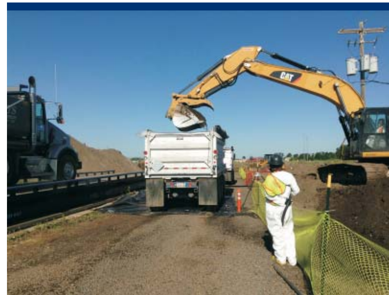
Photo 96 Excavator loading a pup with lead-contaminated soil for transportation and disposal.
