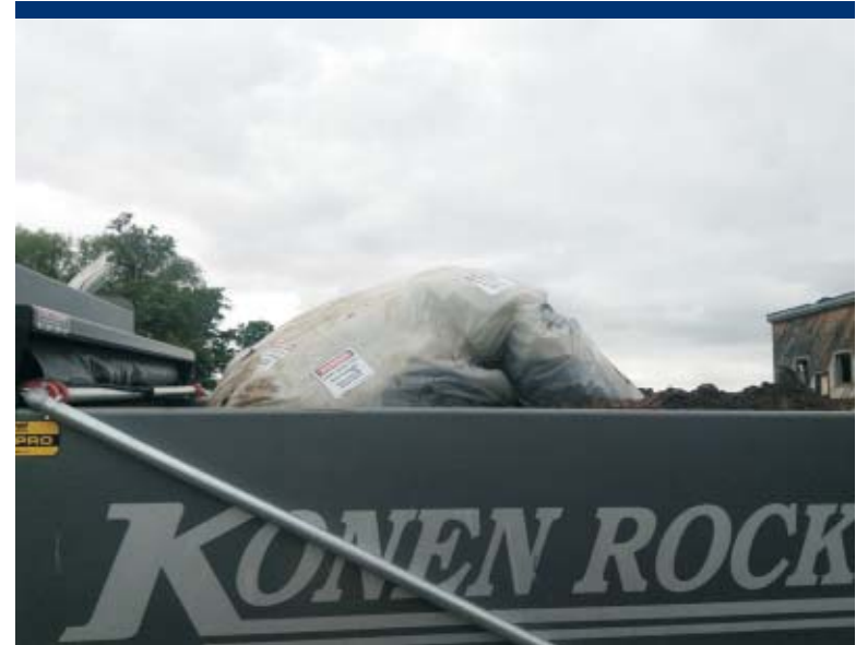
Photo 74 Double-wrapped CAB loaded in a truck for transportation and off-site disposal.
