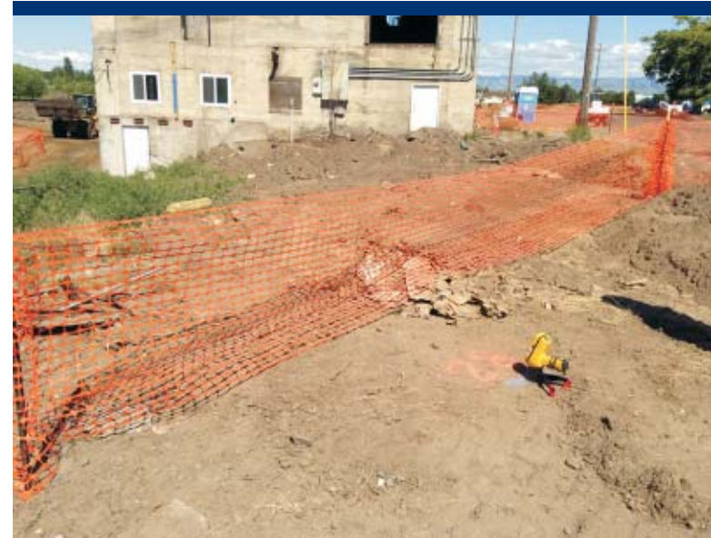
Photo 78 Fencing was installed around the lead-contaminated soil in the Upland Area.
