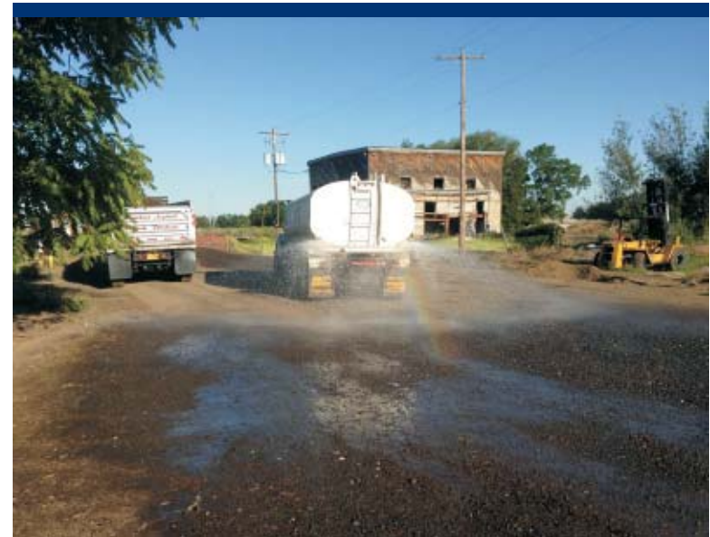
Photo 60 Dust suppression near the weigh scale and shop building.
