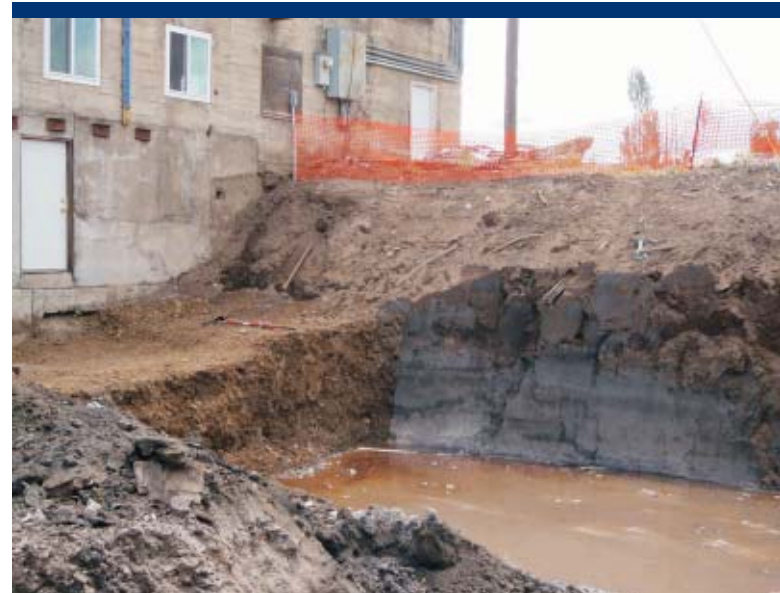
Photo 28 Exposed sidewall of former retaining wall shows heavy staining.
