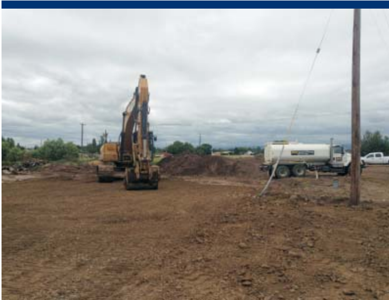
Photo 97 Compacting backfill in Upland Area with the excavator.
