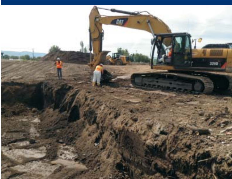
Photo 45 Collecting soil samples from the excavation in the western lobe.
