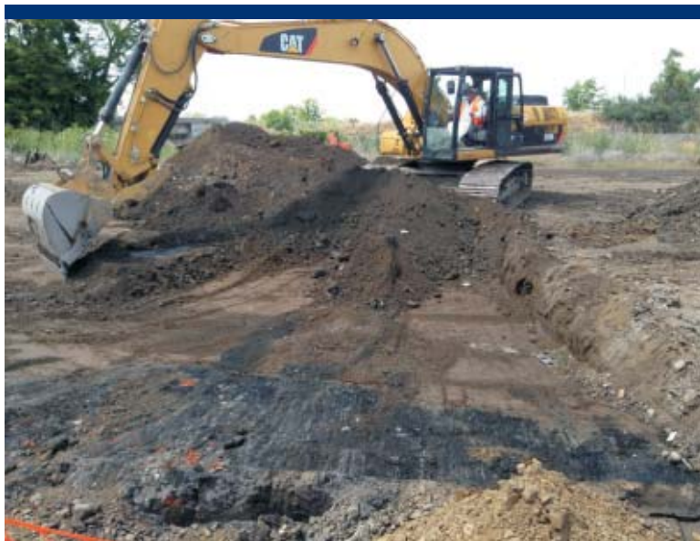
Photo 39 Excavating lead-contaminated soil from the Process Area.
