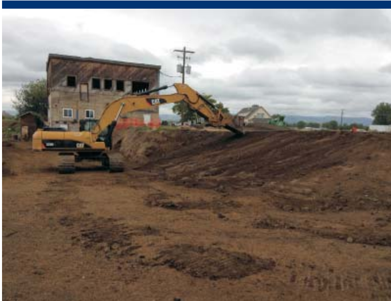
Photo 33 Grading the sidewall along the southern boundary of the SPA.
