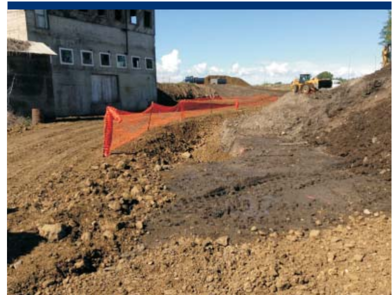
Photo 36 New haul road established and fenced off.
