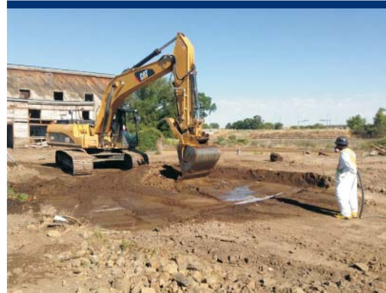
Photo 82 Excavating lead-contaminated soil from the Upland Area in OU2.
