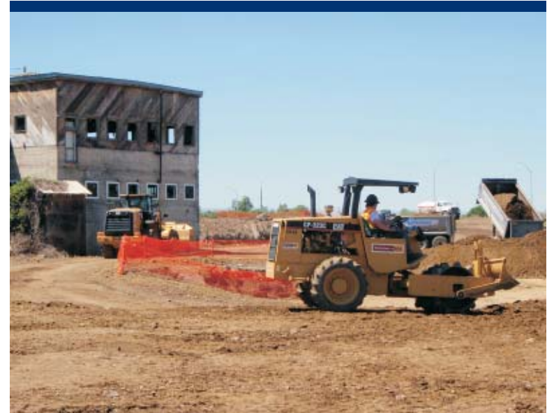
Photo 50 Front end loader, trench roller, water truck and transportation subcontractor all working in the NPA.
