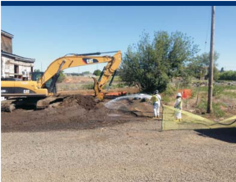
Photo 79 Excavating lead-contaminated soil from the Upland Area in OU1.
