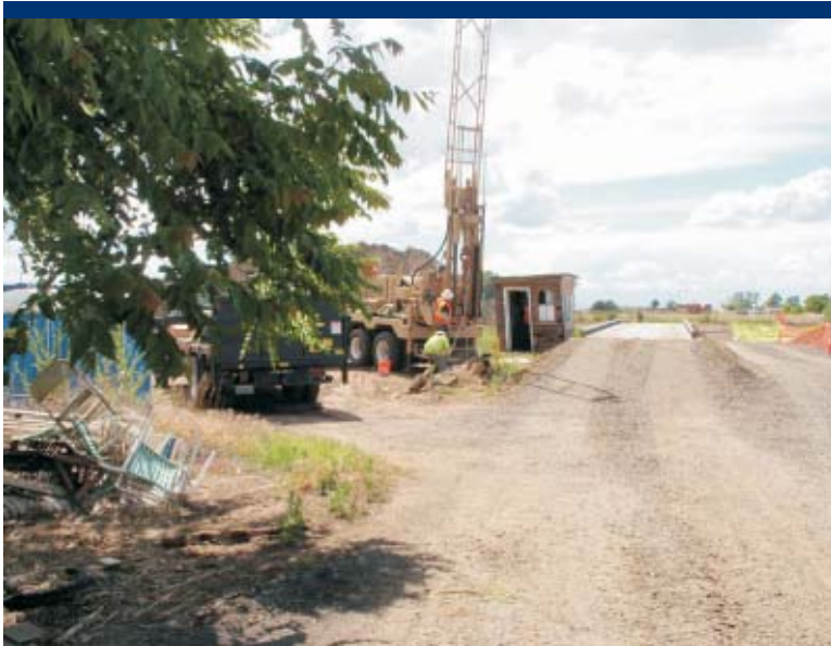
Photo 69 Abandoning MW1 near the weigh scale.
