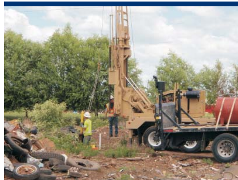
Photo 68 Abandoning MW4 in the northeastern section of the site.
