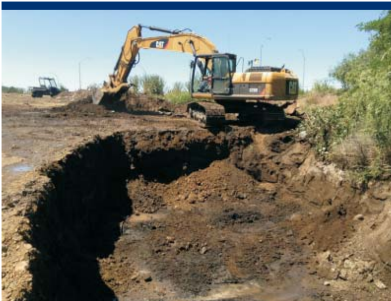
Photo 71 Excavating soil in and around the abandoned MW2 location.
