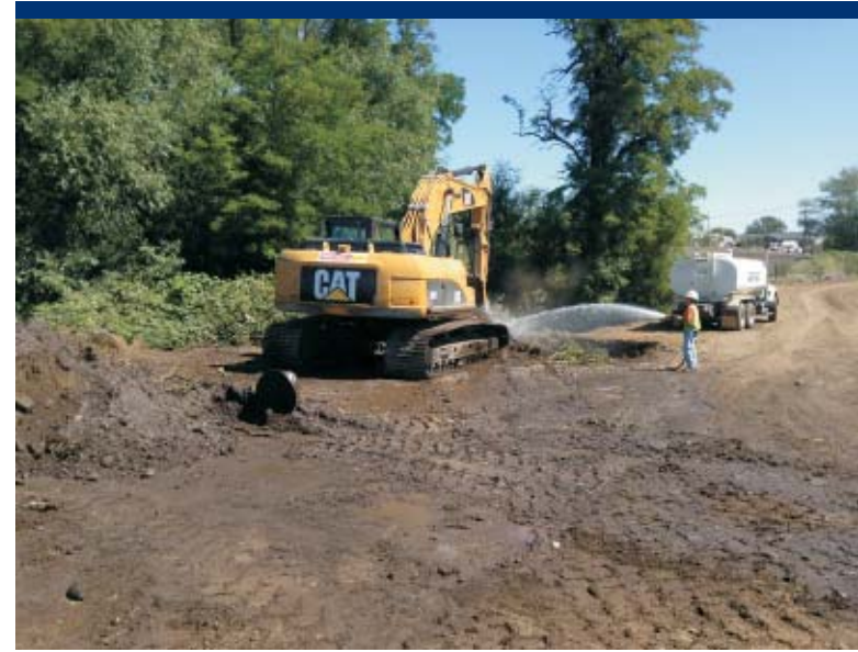
Photo 70 Excavating soil in and around the abandoned MW2 location.
