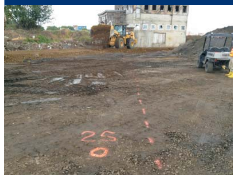
Photo 34 Front end loader building the new haul road; painted line indicates eastern boundary of NPA.
