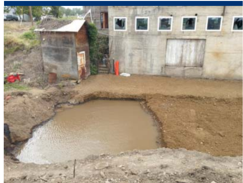
Photo 32 Remaining groundwater in the exposed excavation area in the SPA.
