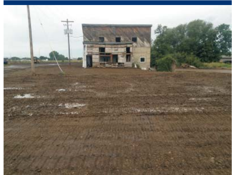
Photo 98 View of the Upland Area after compaction of backfill.
