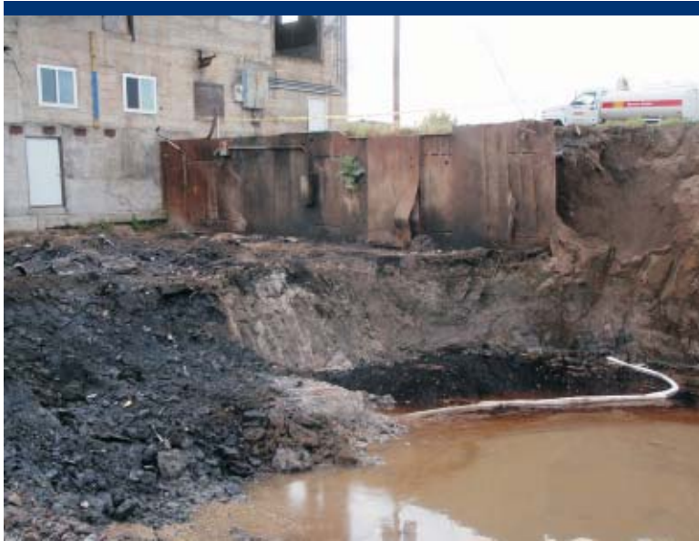
Photo 17 Heavy oil contained by a boom in the excavated area near the shop building.
