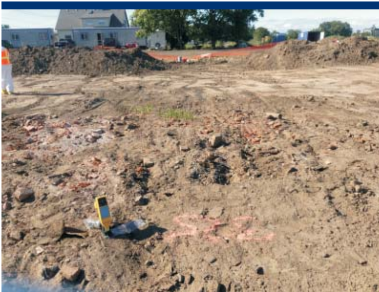
Photo 87 Performing confirmation in-situ screening with the XRF in OU3 in the Upland Area.
