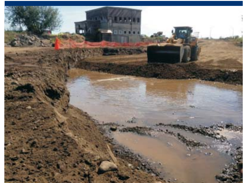
Photo 52 Backfilling the excavation in the NPA and northeastern lobe.
