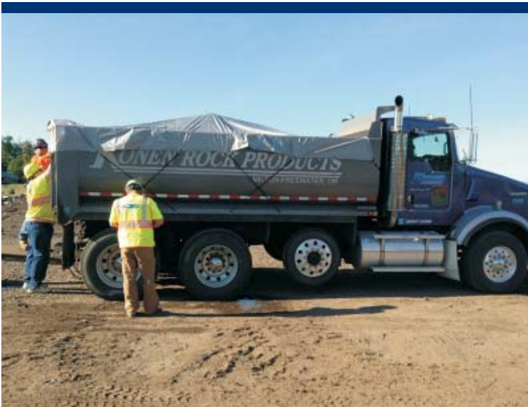
Photo 23 Haul truck being covered with a tarp before leaving the site.
