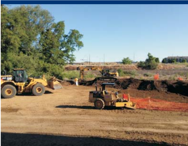
Photo 49 Excavator, front end loader and trench roller all working in the NPA.
