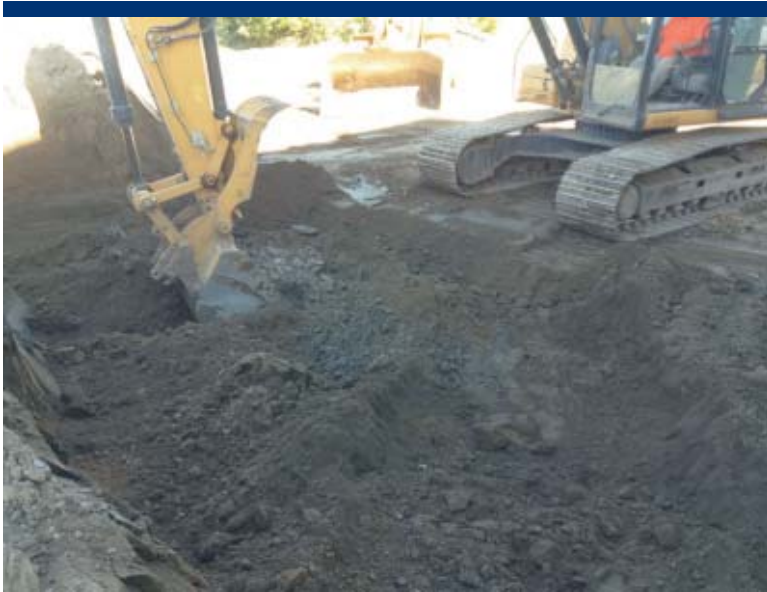
Photo 61 Excavating near former retaining wall to access PCB contaminated soil located near the groundwater.
