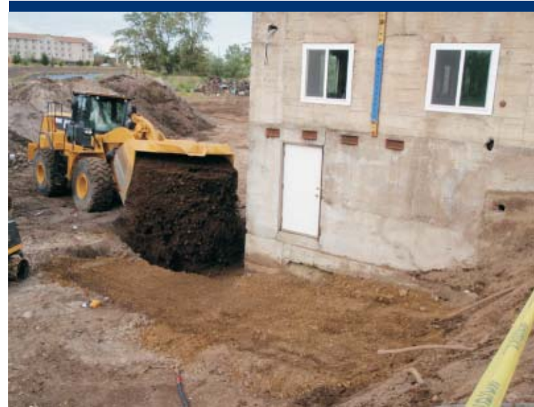
Photo 26 Placing clean backfill in the exposed excavation along the shop building foundation.
