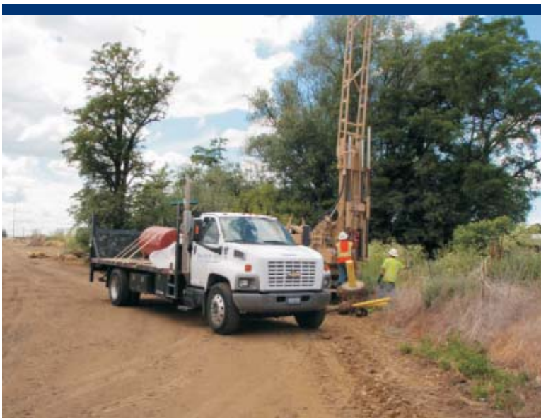
Photo 67 Abandoning MW3 along the northern border of the NPA.
