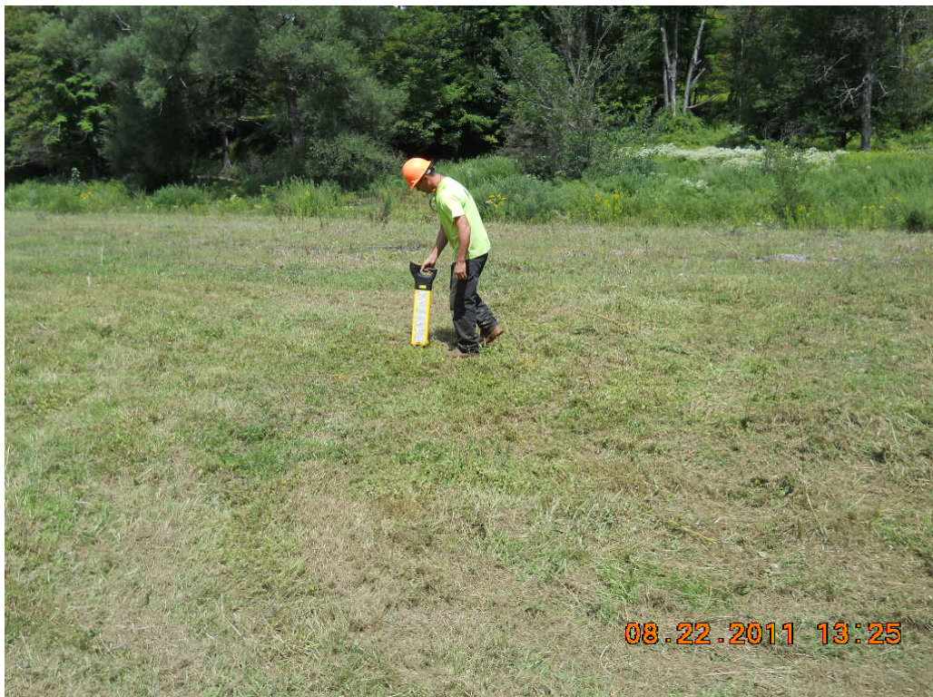
Photograph 2: View of subcontractor clearing location for underground utilities.
