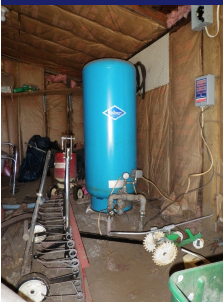
Photo 24 Holding tank located between well and spigot, sample DW12GW.
