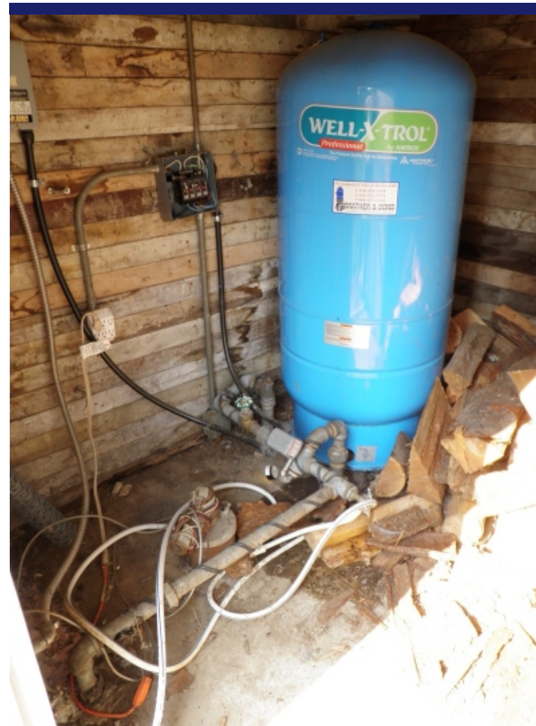
Photo 36 Wellhead and holding tank, spigot behind wall, sample DW26GW.
