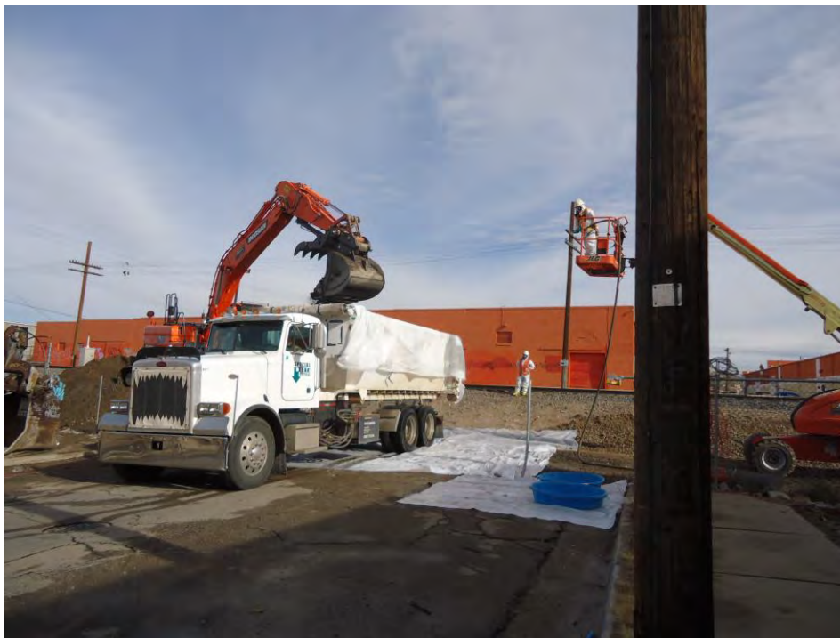
Photograph DSC00854: View looking northeast at truck loading activities along Haines Avenue NW and the NMDOT Railroad Right of Way. Dust suppression in progress.
