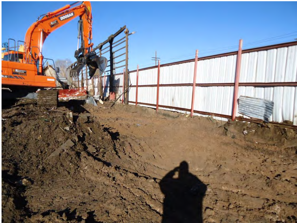
Photograph DSC00926: View looking northeast at excavation activities along Area A, Grid D fence line. Note saturated soil and removal of portions of historical (tall) wind fence.
