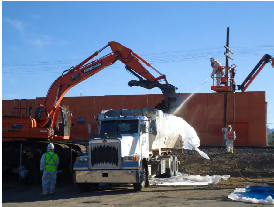
Photograph DSC00885: View looking east at truck loading in Area B. Dust suppression in progress.
