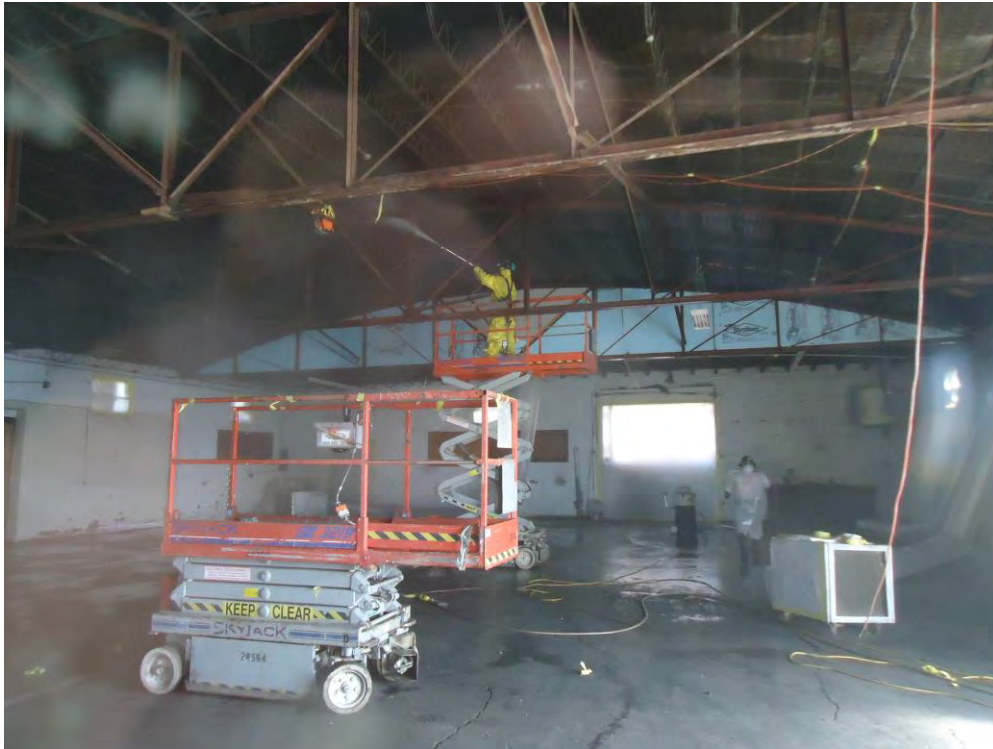
Photograph DSC01124: View (from view port) of Decontamination/Abatement activities in the eastern portion of the Main W. Silver Warehouse.
