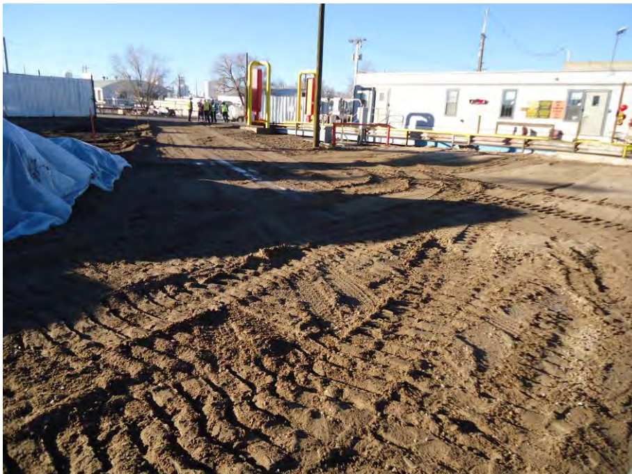
Photograph DSC01001: View looking northwest northern portion of Area A, Grid A after (partial) placement, compaction and grading of cover material.
