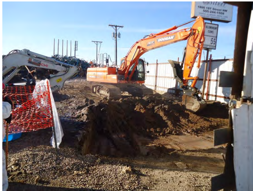
Photograph DSC00753: View looking south at excavation activities in the northwestern portion of Grid A on the W. Silver site. Dust suppression in progress.
