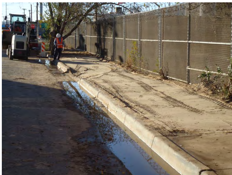
Photograph DSC00633: View of City ROW areas along the north side of Haines Avenue NW following placement and rolling of the backfill.
