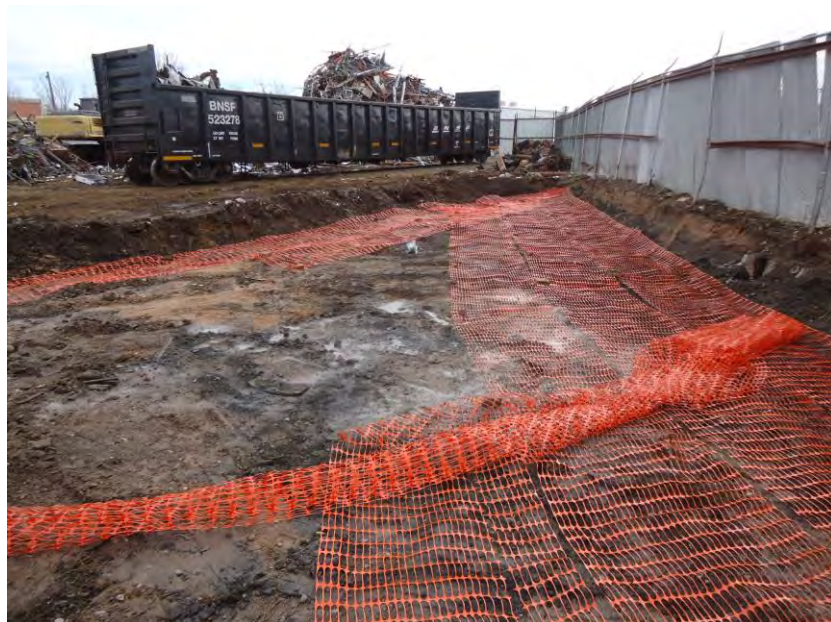
Photograph DSC00680: Close view looking southeast at final excavation depth and placement of barricade fencing in the southern portion of Grid B on the W. Silver site.
