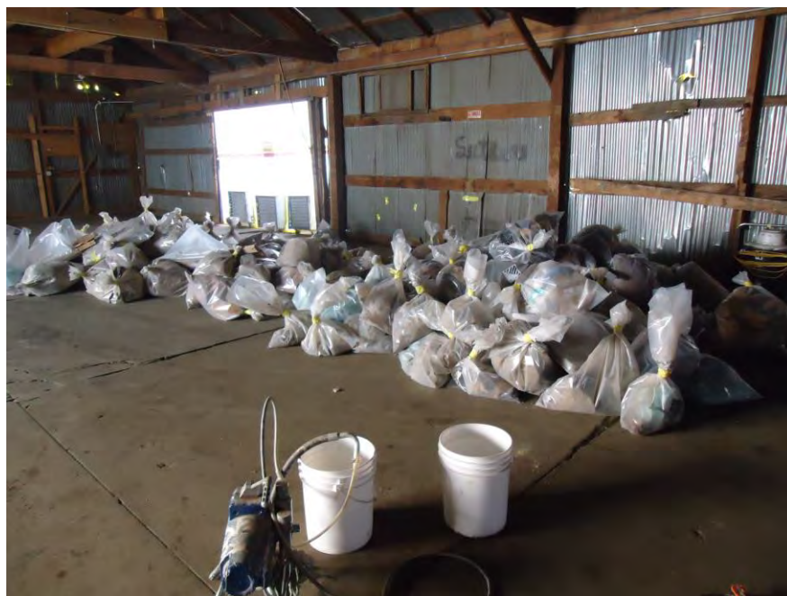
Photograph DSC00602: Interior view of exfoliation building and bagged asbestos resulting from the abatement of the building.
