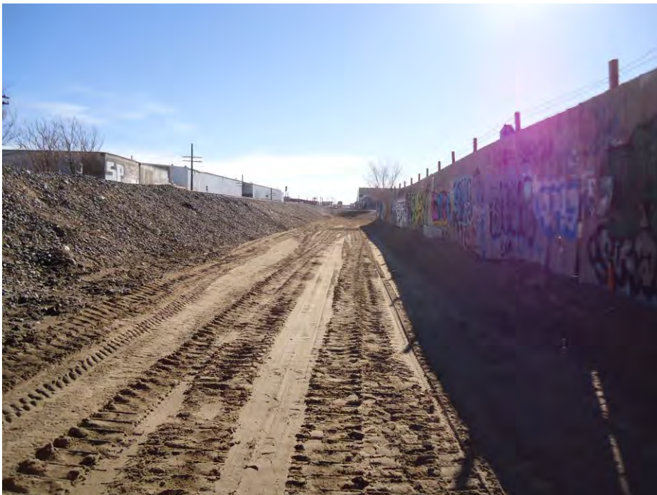
Photograph DSC00892: View looking south at Area B after cover material placed and graded.
