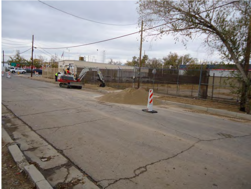
Photograph DSC00633: Final grading of “crusher fines” in the City ROW, Area E, Grids 010 and 011.
