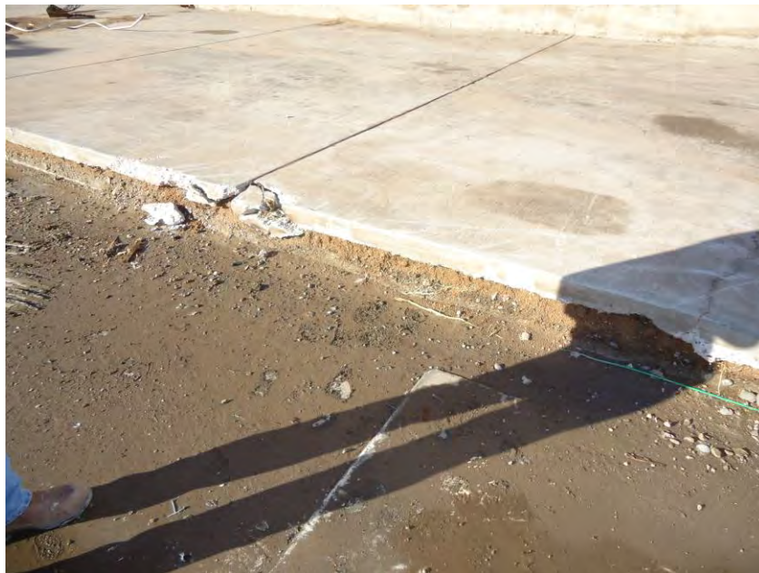
Photograph DSC00718: View looking northwest at exposed soil area where a visible vermiculite layer was observed under the concrete adjacent to the former exfoliation building concrete pad.
