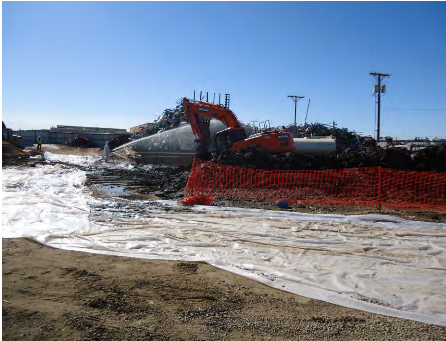
Photograph DSC00940: View looking south at loading operations from the stockpile on the W. Silver site. Poly layer is placed to allow truck with cover material to traverse to the Grid D area to dump.
