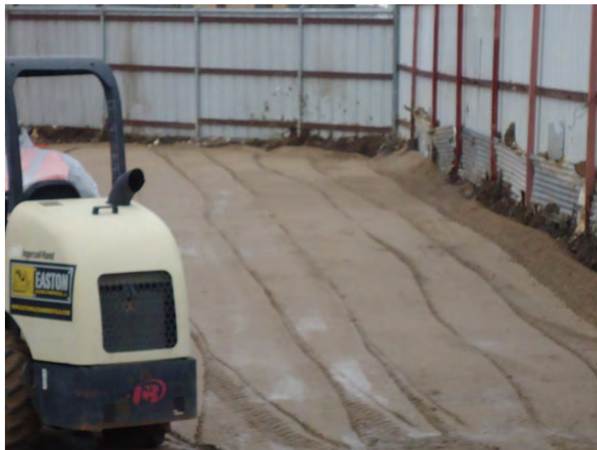
Photograph DSC00652: View of placement and compaction of "Cover Material" (Type A1A Product) within the excavated and cleared areas (B North, A South) on W. Silver site.
