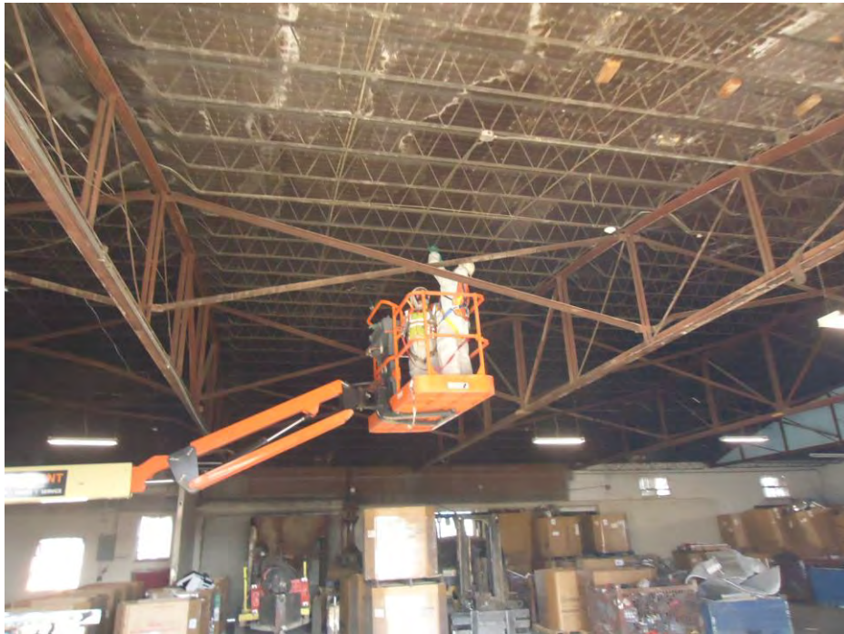
Photograph DSC00848: View of the collection of ceiling tiles/insulation samples from the W. Silver main warehouse, facing north.
