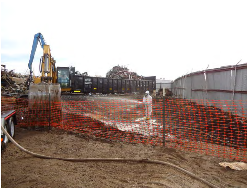
Photograph DSC00677: View looking southeast at excavation activities in the southern portion of Grid B on the W. Silver site. Dust suppression in progress.
