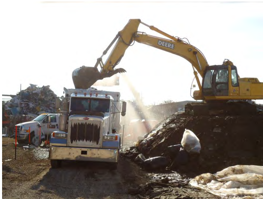
Photograph DSC0594; View east-southeast of loading operations. Note ongoing wetting.
