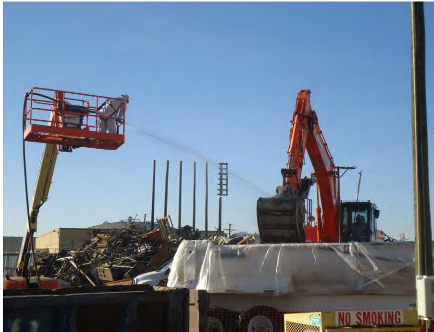
Photograph DSC00762: View looking southwest at loading from the soil stockpile in Grid A on the W. Silver site. Dust suppression in progress.
