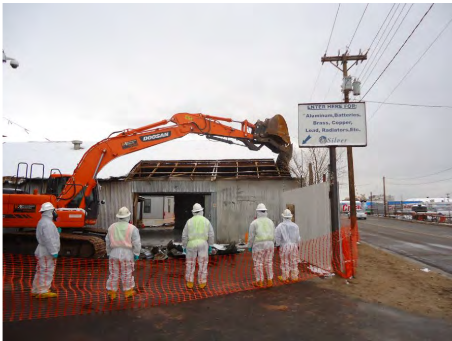
Photograph DSC00686: View looking south at initial demolition activities of the former exfoliation building, starting with removal of the sheet metal roofing,
