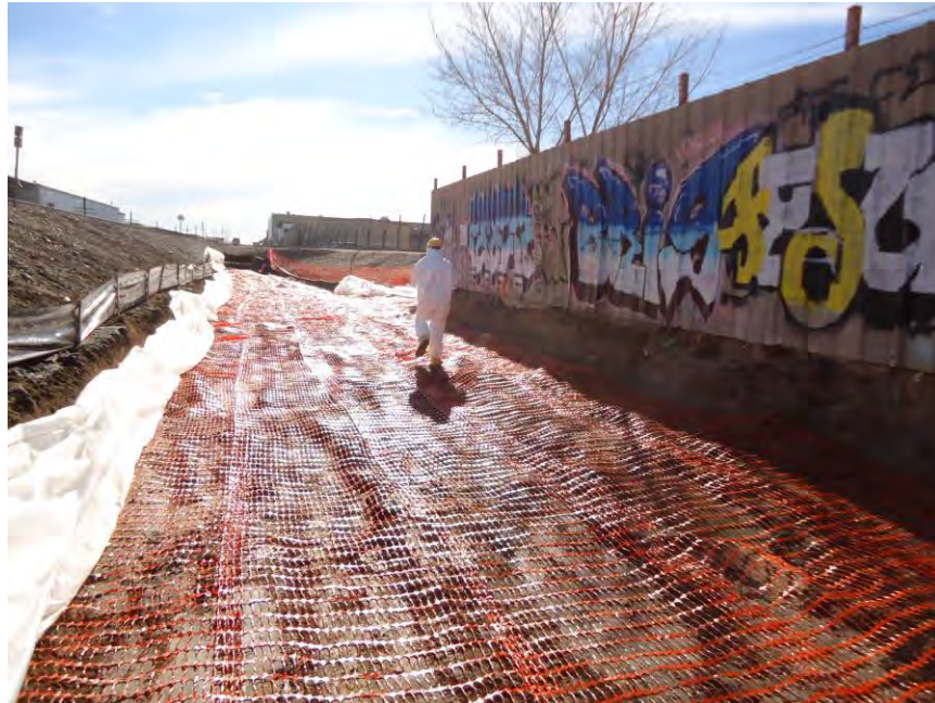
Photograph DSC00833: View looking south at confirmation sampling within excavated area the southern portion of the NMDOT Railroad ROW (Area B).
