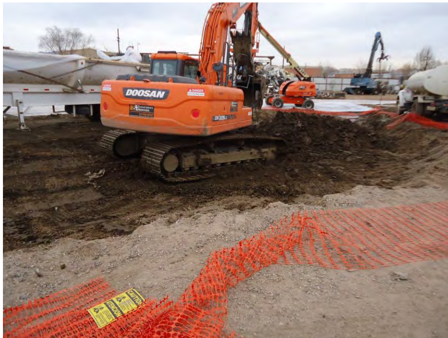
Photograph DSC00950: View looking east at loading operations and stockpile management at the W. Silver stockpile. Note current depth of approximately 30" bgs.
