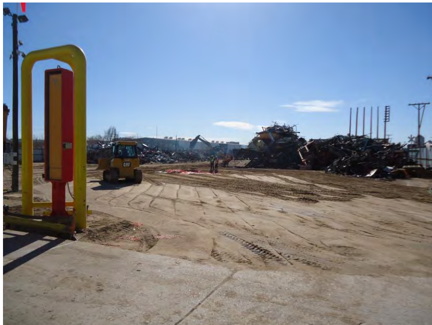
Photograph DSC01022: View looking south at final remaining placement, compaction and grading of cover material in the area of the (former) soil stockpile in Area A, Grid A.
