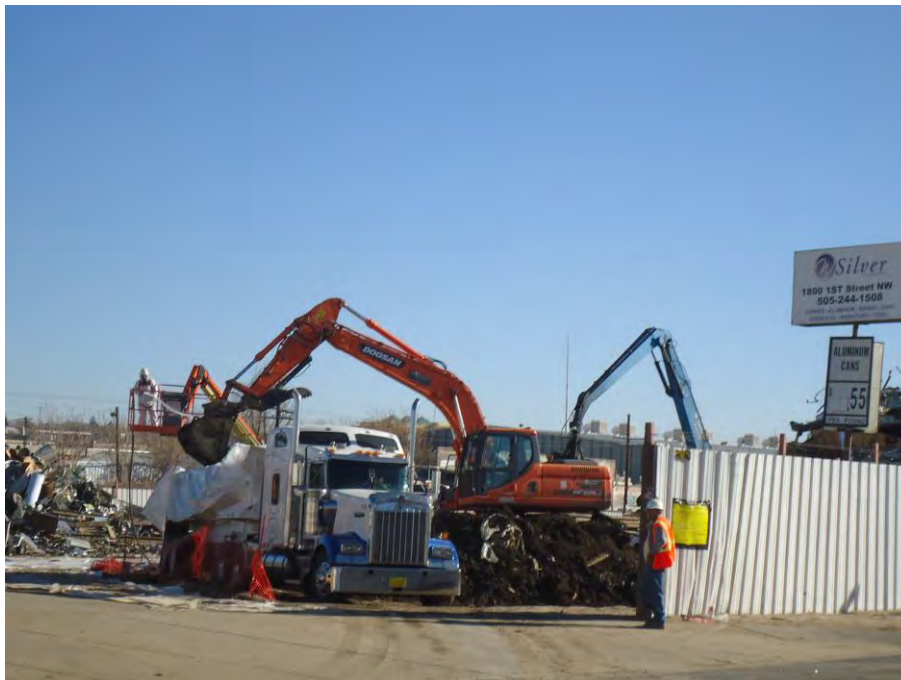
Photograph DSC00942: View looking southeast at loading operations from the W. Silver stockpile. Dust suppression in progress.
