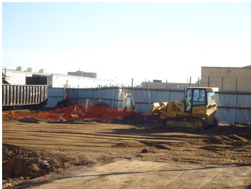
Photograph DSC00669: Close view looking south at grading and compaction of cover material in Area A, Grids A/B on the W. Silver site
