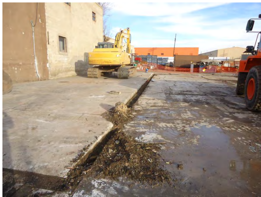
Photograph DSC00725: View looking east at excavation activities in a dirt strip (Grid 001) along the northern portion of the concrete pad adjacent to the former exfoliation building. A layer of visible vermiculite was observed in the soil under the concrete pad.
