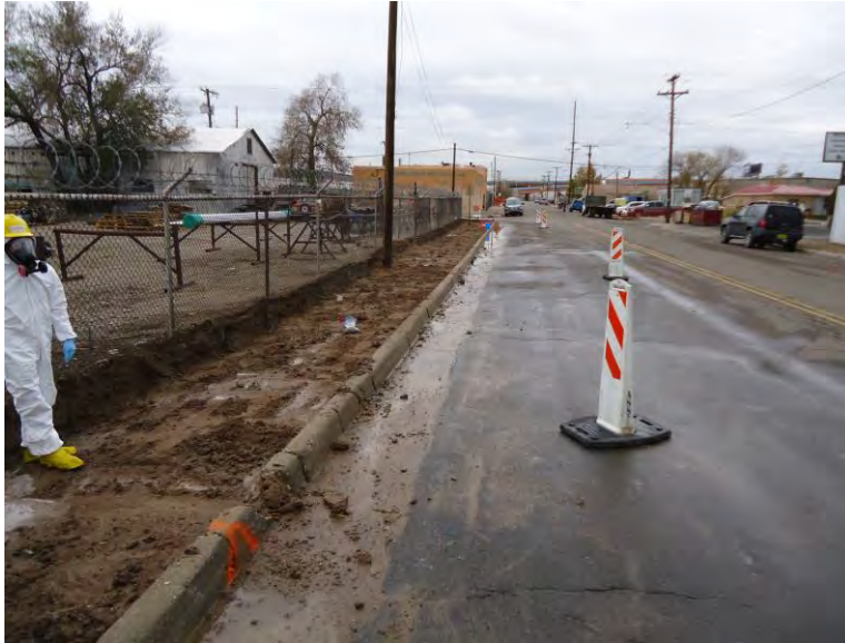
Photograph DSC00647: Expanded view of Area E, Grid 006 after conformation sample collection and prior to backfilling.
