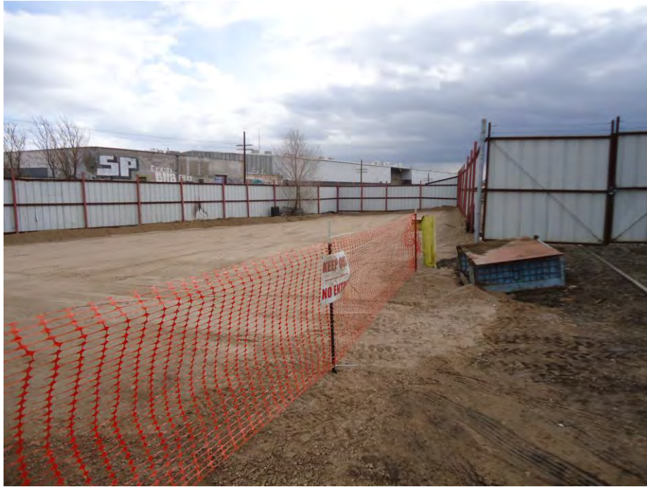
Photograph DSC00788: View looking southeast at Area A, Grid E after cover material was placed, compacted and graded immediately prior to departure for Holiday break.
