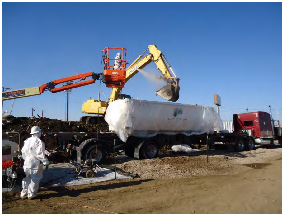
Photograph DSC00591; Expanded view southwest at loading operations. Note wetting (pressure washer) operations.
