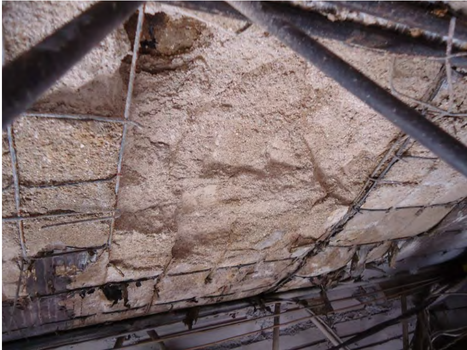
Photograph DSC01108: Close view of degraded ceiling insulation/tiles in the Main W. Silver Warehouse. Degraded areas prepped to assure adequate bonding with (Asbestos-Safe) Encasement material.
