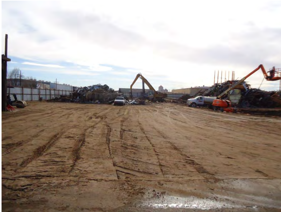
Photograph DSC01005: View looking south at Area A, Grid C following placement of cover material. Grading and compaction ongoing.
