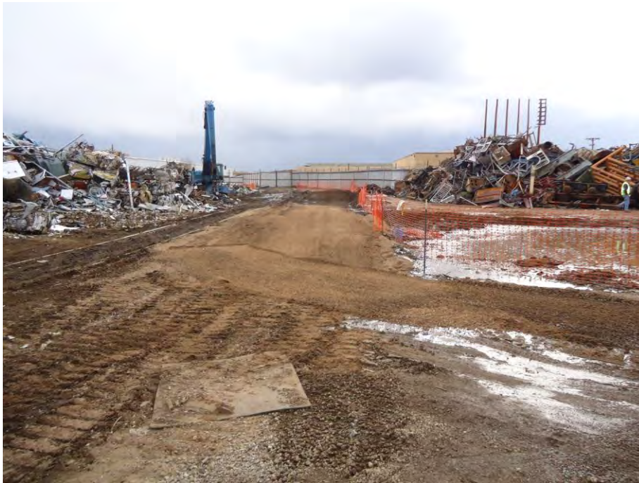
Photograph DSC00791: View looking south at cover material placed and graded along western side of rail spur on W. Silver site. Material placed to displace standing water resulting from recent rain and water used for decontamination.
