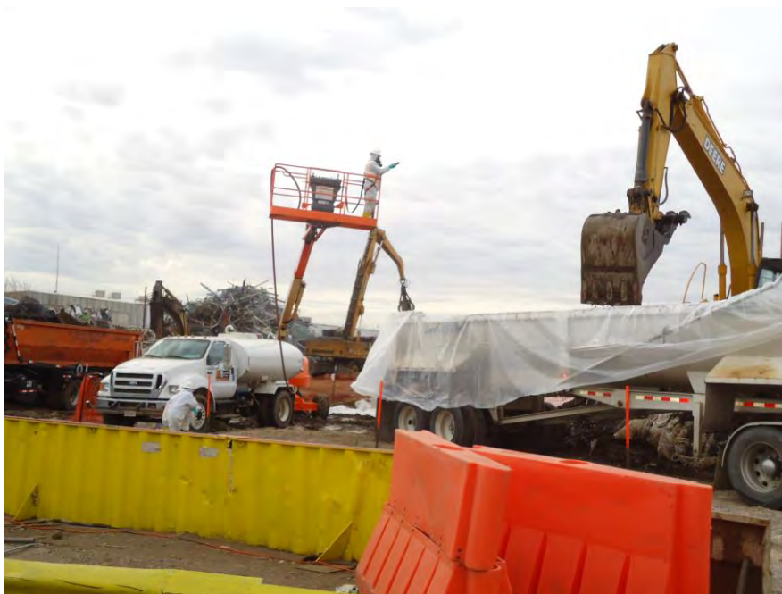
Photograph DSC0616; View southeast of loading operations. Note ongoing wetting/dust suppression activities.
