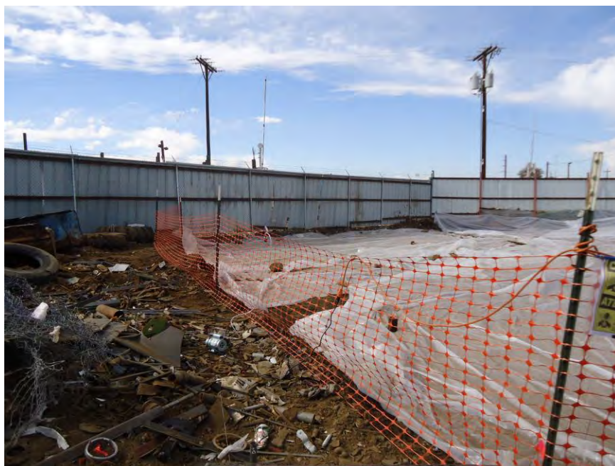
Photograph DSC00610; View southeast of excavated and covered grid on W. Silver site. Note air sampling location on barricade fencing.
