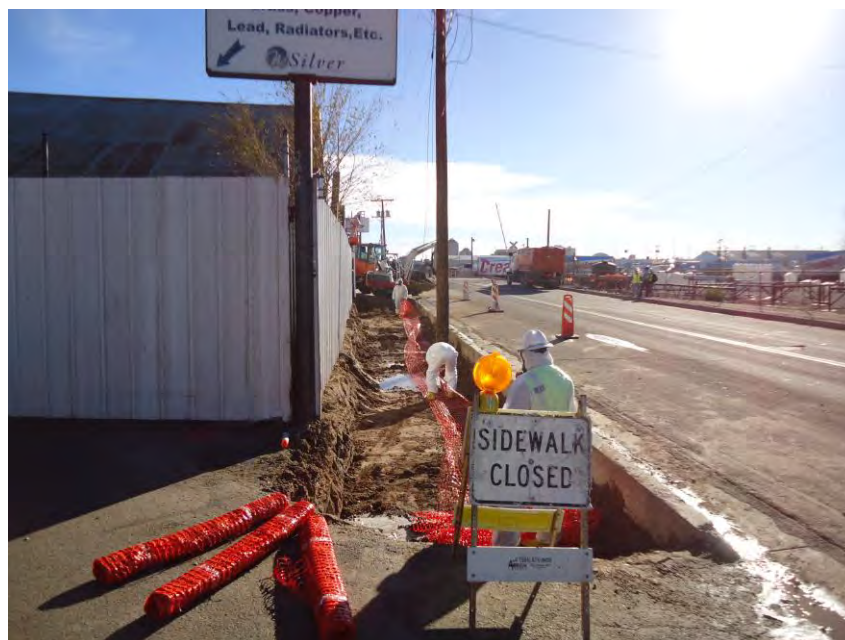
Photograph DSC00673: Expanded view looking south at final excavation depth and ongoing confirmation sampling and placement of barricade fencing in Grid 001 of the City ROW prior to backfilling
