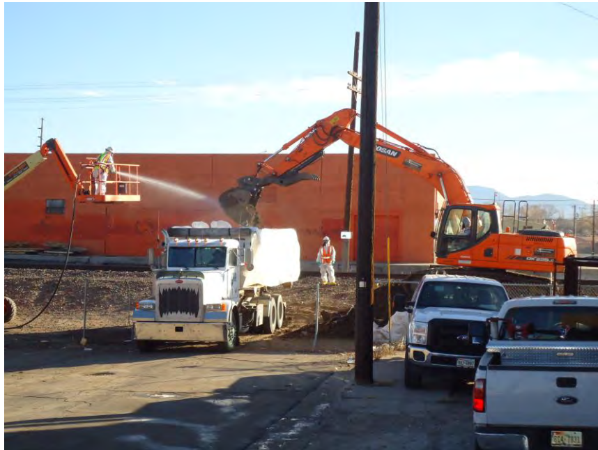
Photograph DSC00827: View looking east at truck loading activities along Haines Street and the NMDOT Railroad Right of Way. Dust suppression in progress.
