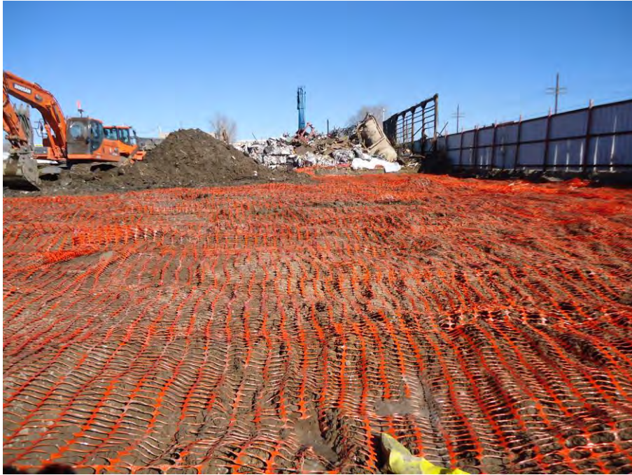
Photograph DSC00931: View looking north at excavated areas of W. Silver Area A, Grid D with barricade fencing in excavation base prior to placement of cover material.
