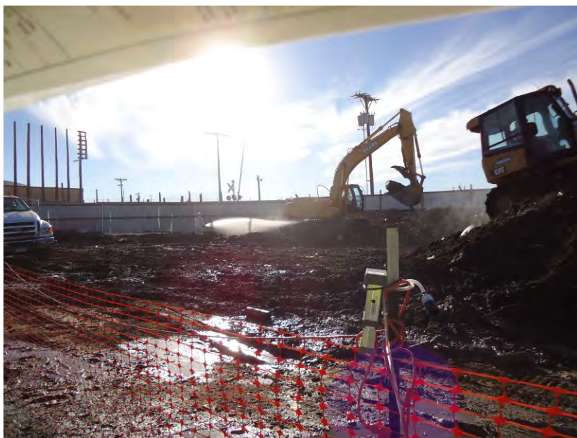
Photograph DSC00567; View facing west at excavation and stockpiling activities. Note apparent adequate wetting.
