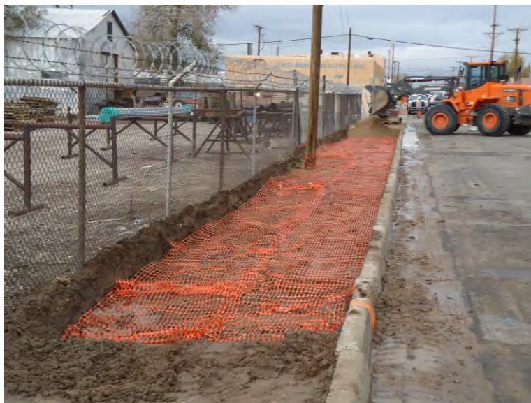
Photograph DSC00649: View of Area E, Grid 006 with barricade fencing in the excavation prior to backfilling.
