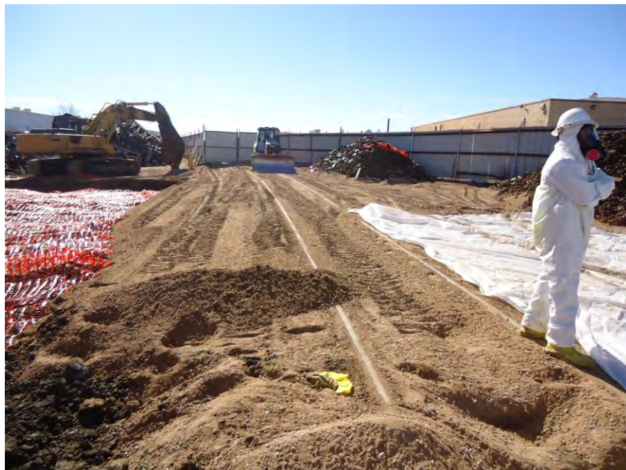
Photograph DSC00933: View looking south at Area A, Grids D and E along rail spur after initial placement and compaction of cover material.
