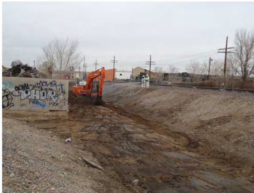
Photograph DSC00816: View looking north at excavation activity in the southern portion of Area B. Dust suppression in progress.
