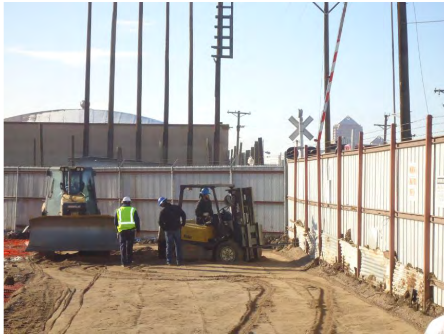
Photograph DSC00654: Photo south of forklift stuck on test track of compacted Cover Material.
