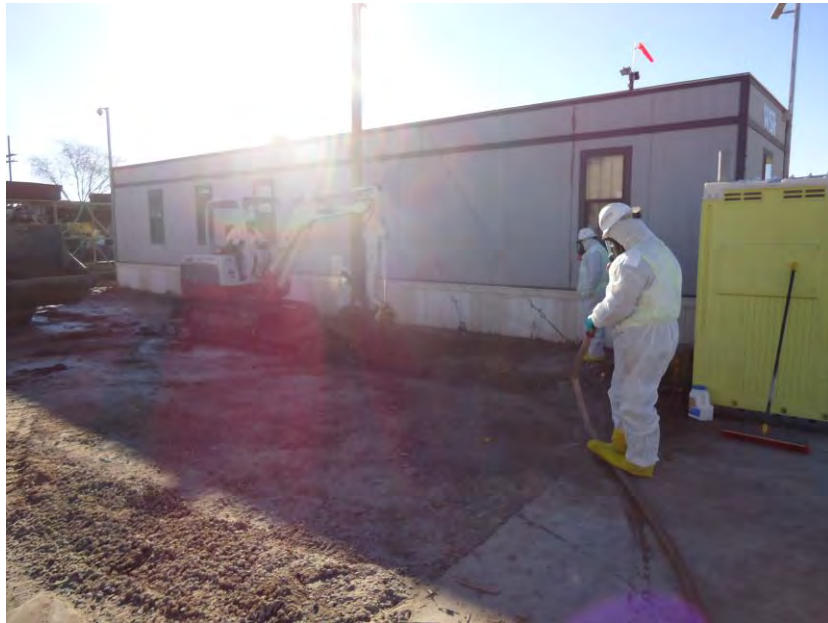
Photograph DSC00750: View looking southeast at excavation activities in Grid 002 of Area A on the W. Silver site. Dust suppression in progress.
