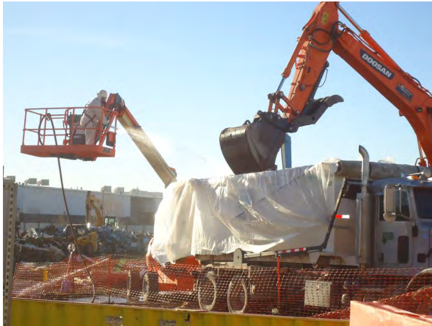
Photograph DSC00757: View looking southeast at loading from the soil stockpile in Grid A on the W. Silver site. Dust suppression in progress.
