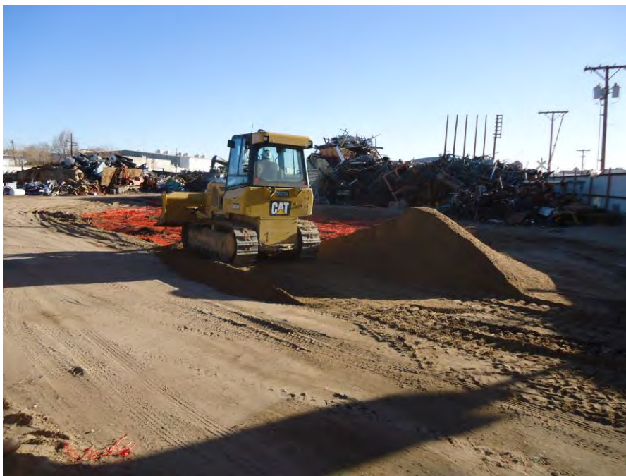
Photograph DSC01018: View looking southeast at remaining placement, compaction and grading of cover material in the area of the (former) soil stockpile in Area A, Grid A.
