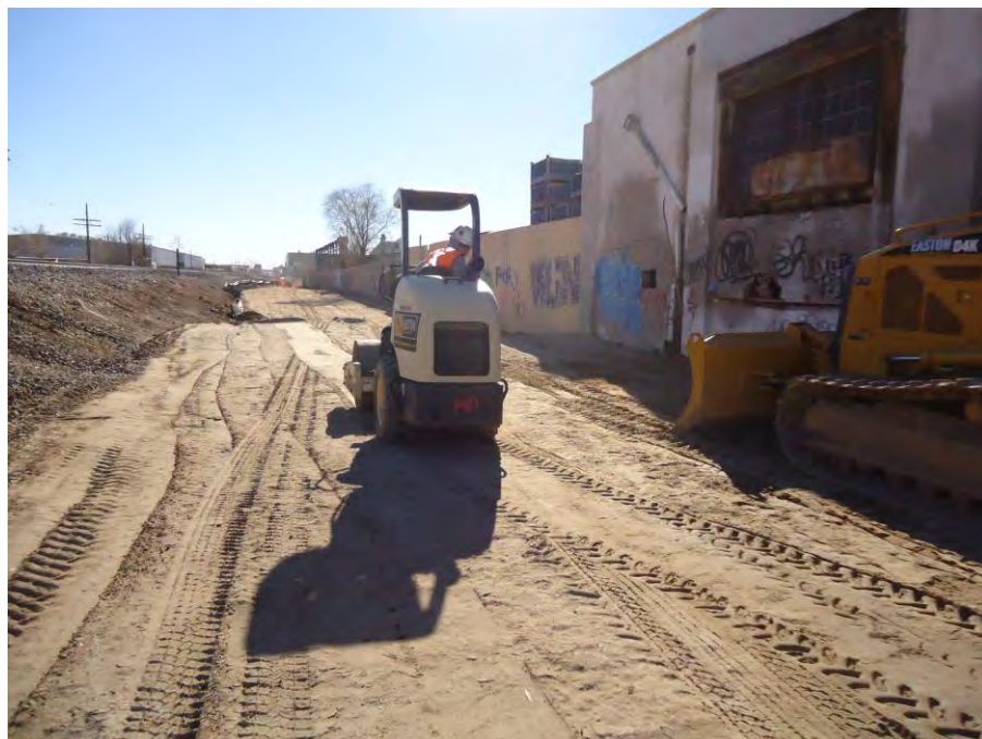
Photograph DSC00888: View looking south at compacting and grading of cover material placed in the northern portion of Area B.
