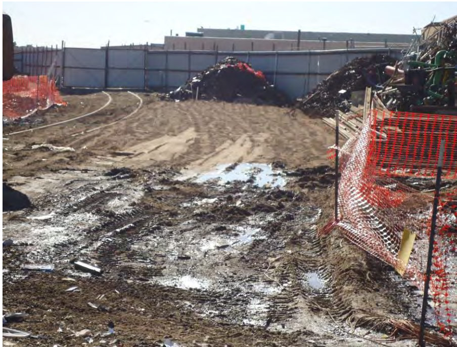
Photograph DSC00904: View looking south at Area A, Grid D west of the rail spur after excavation and placement of cover material.
