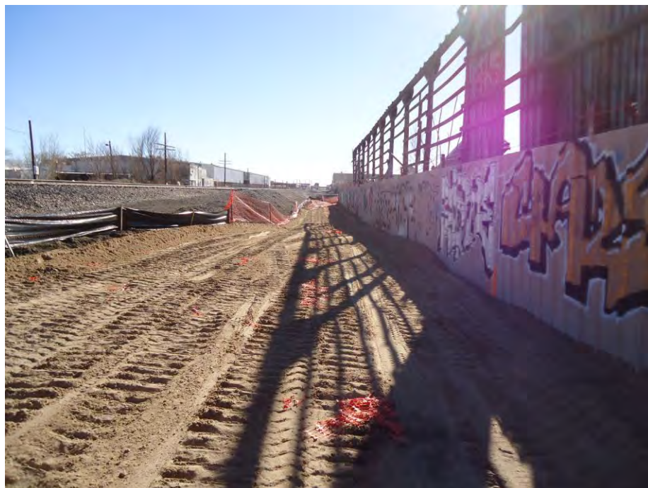
Photograph DSC00884: View looking south at initial layer of cover material placed in the southern portion of Area B. Additional cover material, compacting and grading still required.
