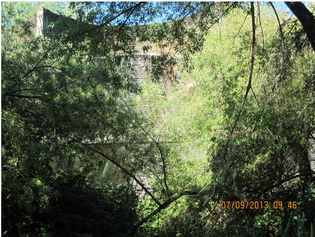
Photo 4. View at Downstream Base of Dam Showing Excessive Vegetation Growth.
