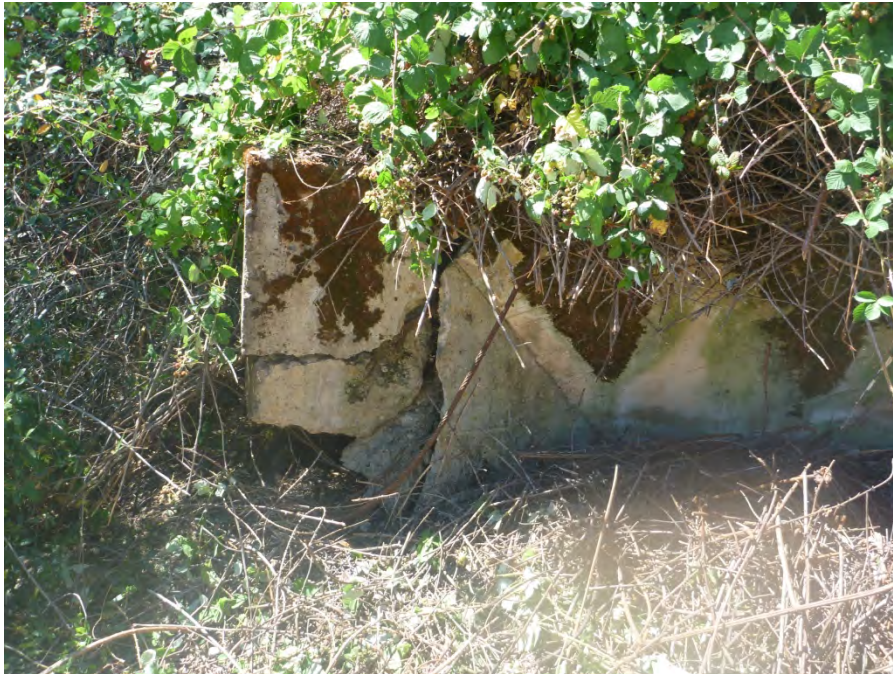
Figure 10 Upper Portion or Remains of Buttrass 1
