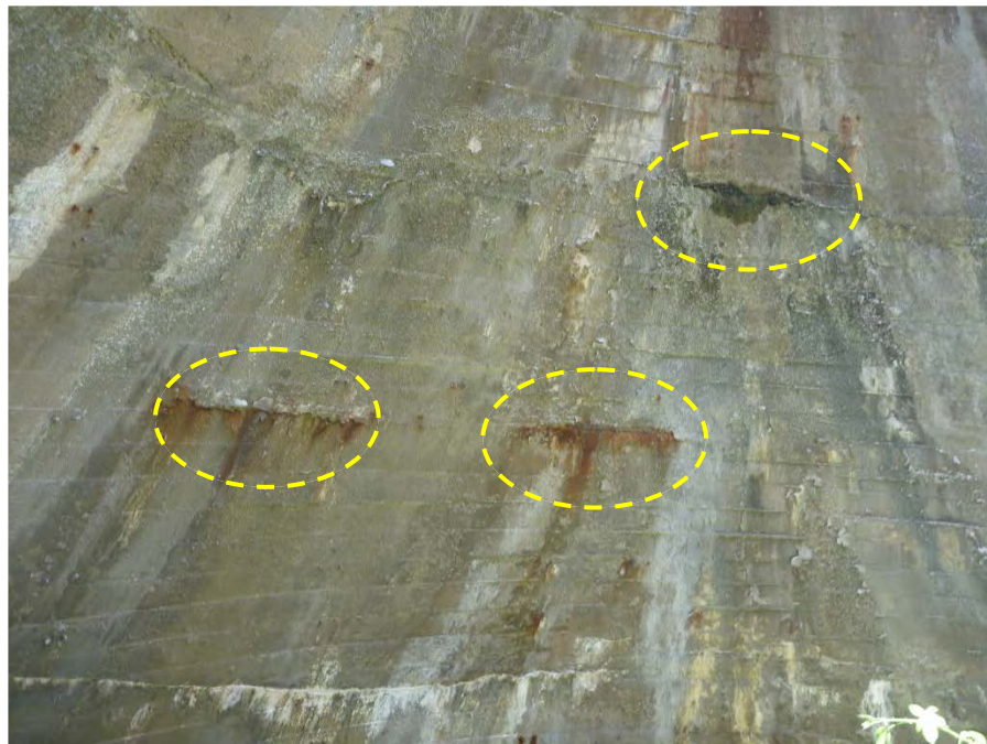
Figure 6 Rust Staining from Embedded Cable
