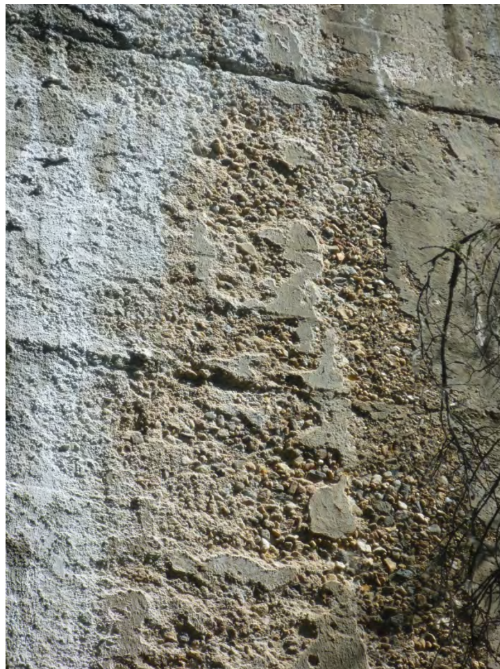
Figure 9 Exposed Aggregate of Buttress Wall
