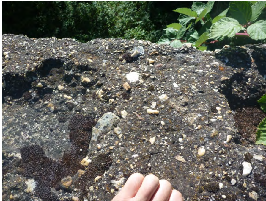
Figure 3 Worn Surface of Concrete (Typical)
