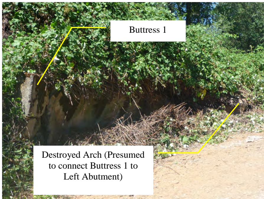
Figure 13 Arch Connecting Buttress 1 to Left Abutment
