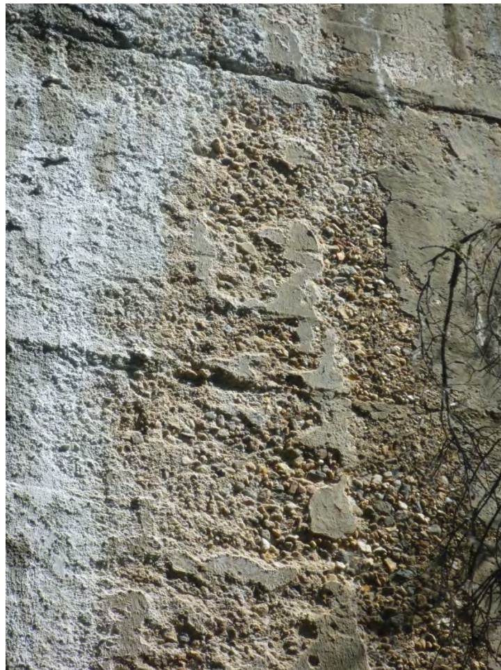
Figure 9 Exposed Aggregate of Buttress Wall
