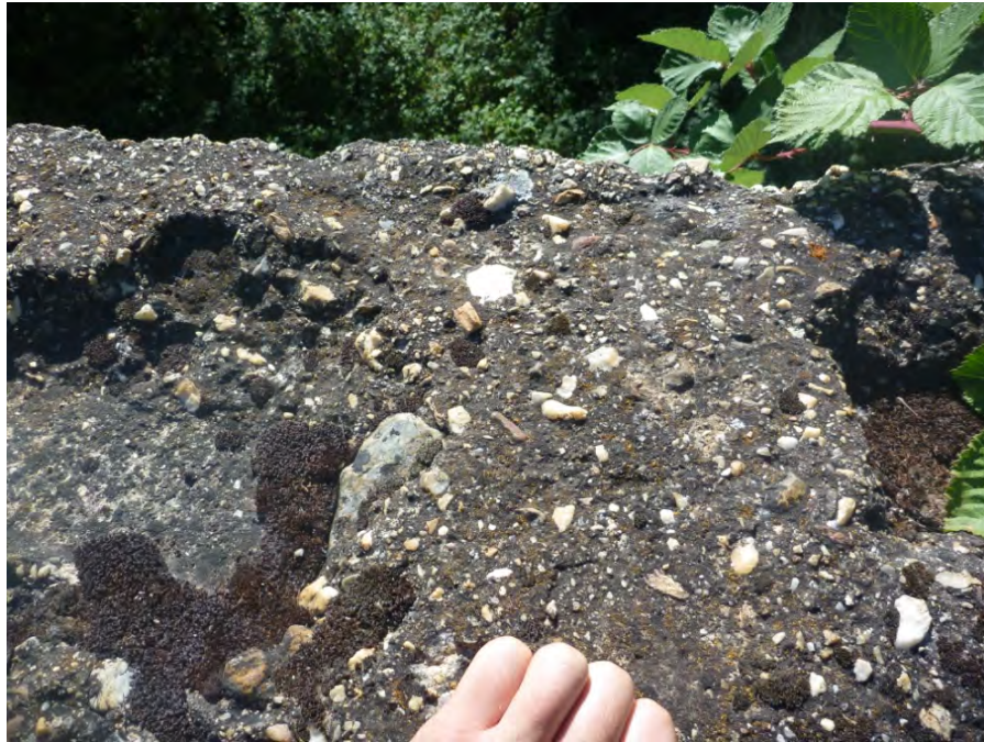
Figure 3 Worn Surface of Concrete (Typical)
