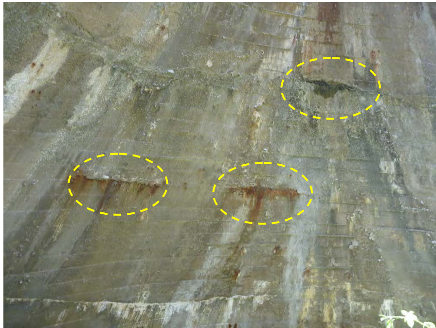
Figure 6 Rust Staining from Embedded Cable
