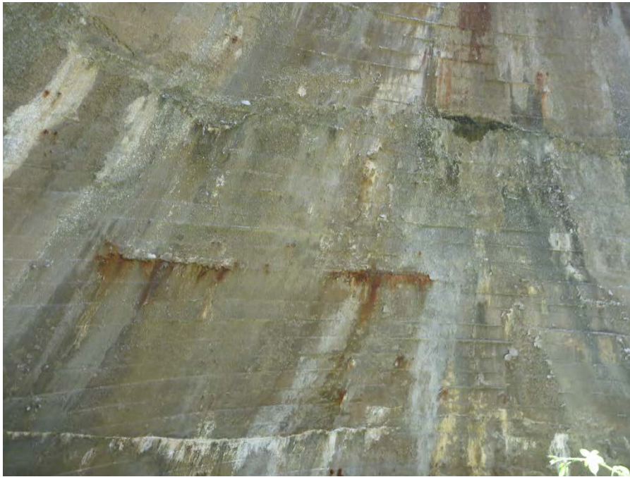
Figure 4 Rust Staining on Downstream Arch Face (insufficient cover around wire ropes)
