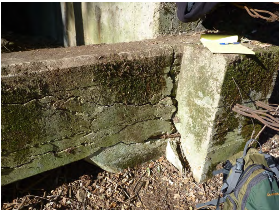
Figure 9 Concrete Brace at Arch 5
