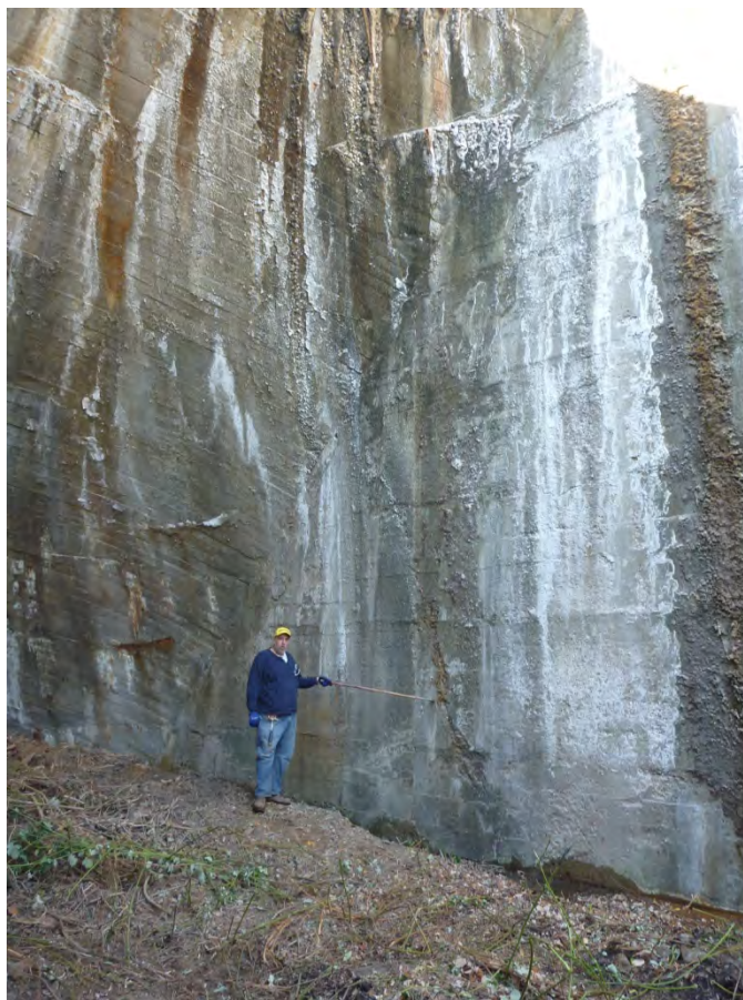
Figure 15 Diagonal Crack in Buttrass #8
