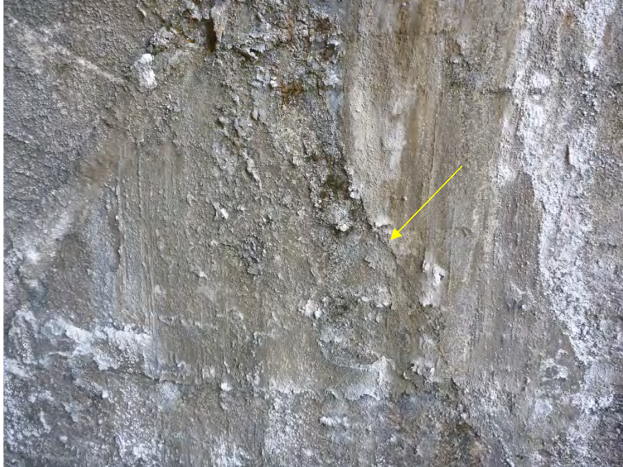
Figure 14 Diagonal Crack on Right Side of Buttrass #6
