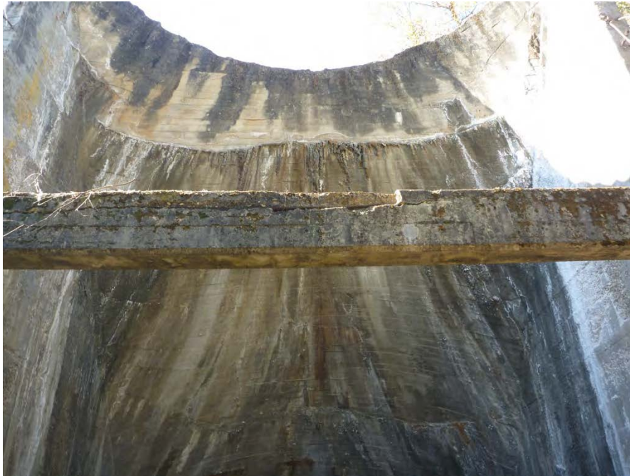
Figure 10 Bracing at Arch 7 Showing Signs of Cracking, Delamination, and Spalling (Typical)
