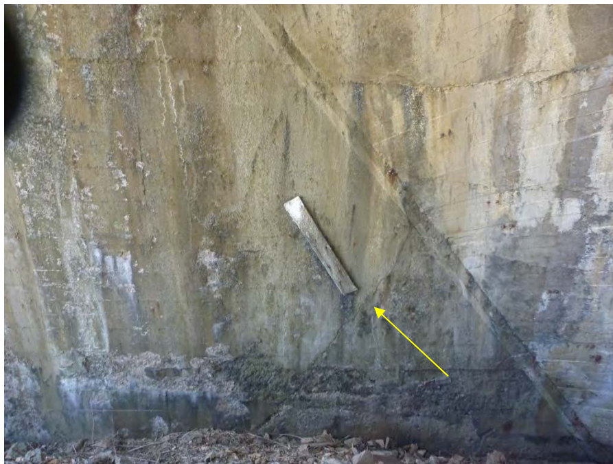
Figure 13 Diagonal Crack on Left Side Buttress #6
