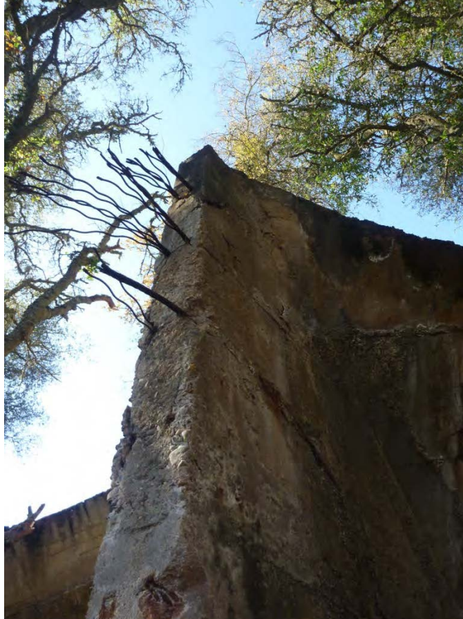
Figure 12 Buttress Wall #4 Showing Signs of Cracking and Spalling Around Embed Wire rope
