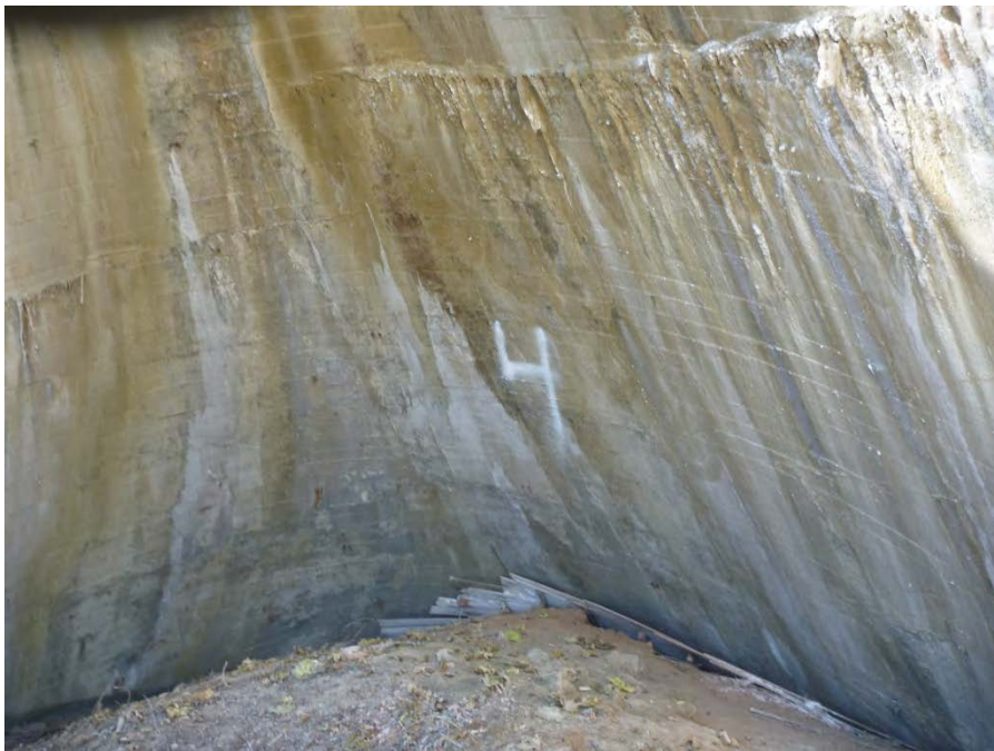
Figure 5 Leftover Formwork from Construction of the Dam
