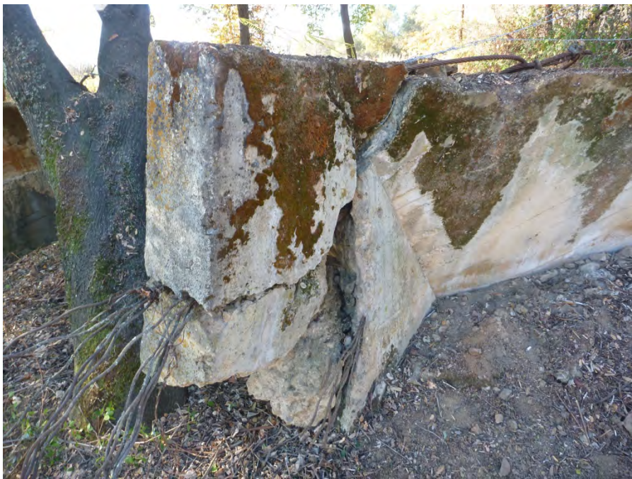
Figure 11 Buttress Wall 2 in Severe Deterioration
