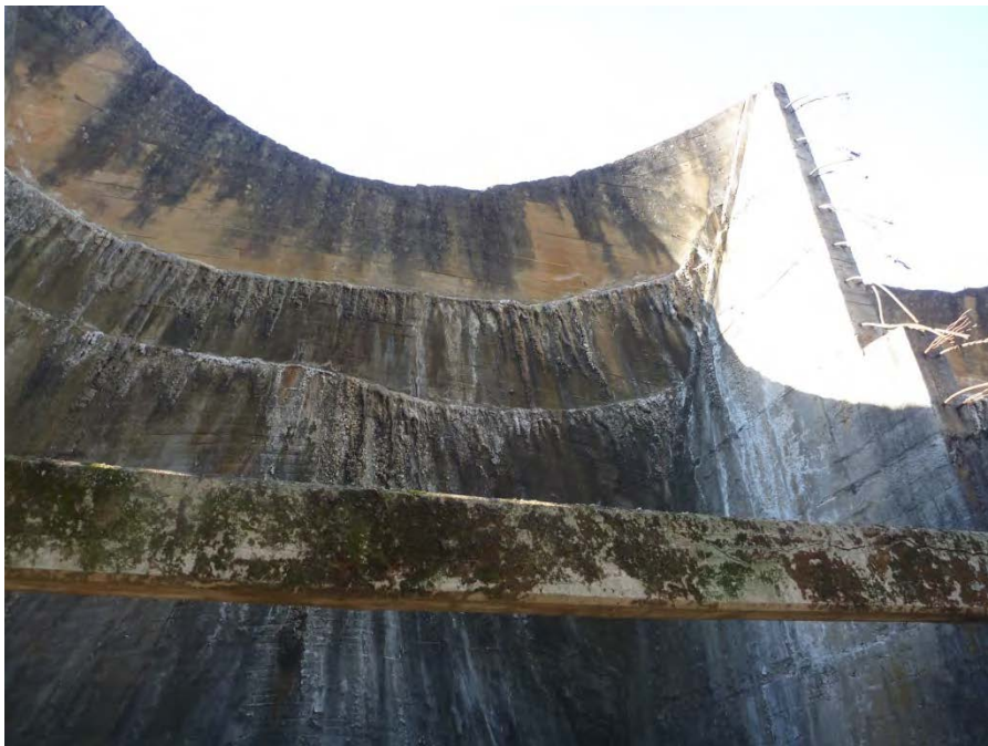
Figure 3 Typical Efflorescence, Rust Staining, and Algae Build up on Arches and Buttress Walls
