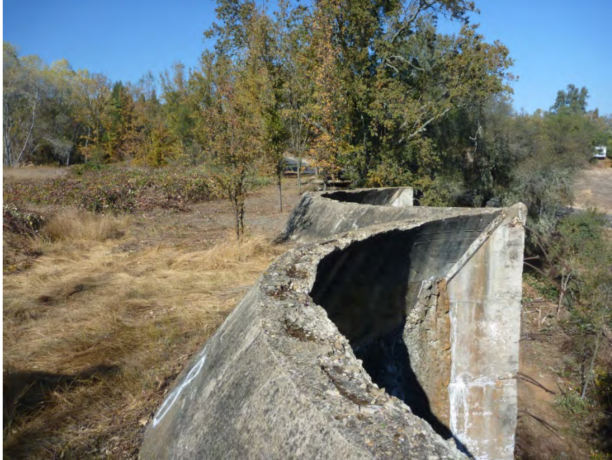
Figure 2 View to the Left of Arch 8, Typical Worn Concrete Surface
