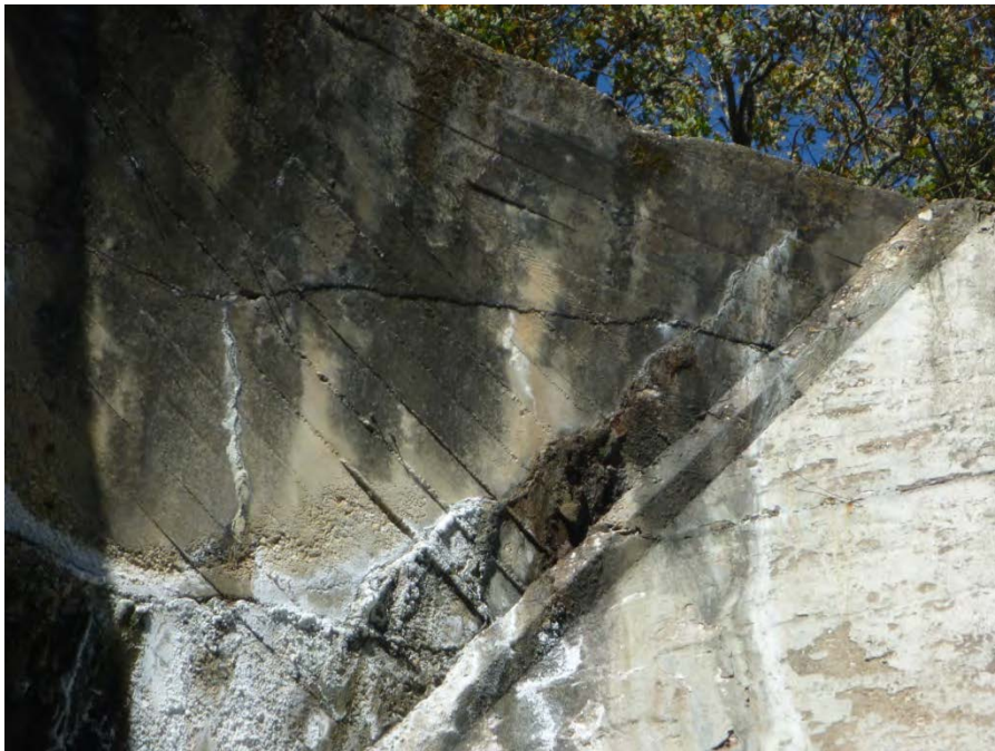
Figure 7 Crack in Arches 7, 8, 9, & 10 Typical Both Sides
