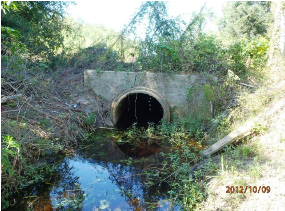
Photo 15: View of the 42-inch RCP culvert where Stream 01 enters the VCC property at North Kate Street.
