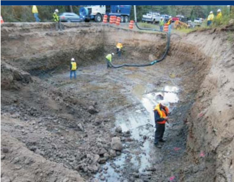
Photo 13 Pit characterization and vacuum truck operation.
