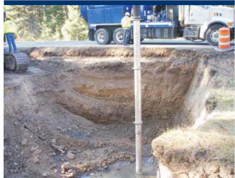
Photo 10 Vacuum truck removing contaminated groundwater from the excavation pit.
