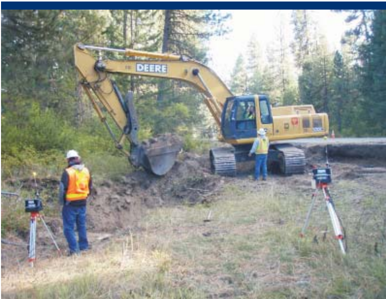
Photo 7 Excavation of contaminated soil with START performing air monitoring.
