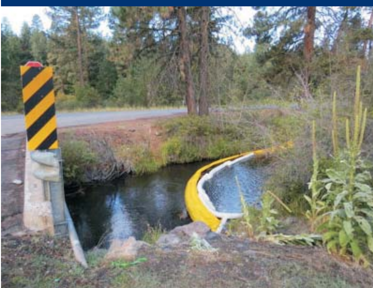
Photo 17 Boom deployed in Beaver Creek near SW002 sample location.
