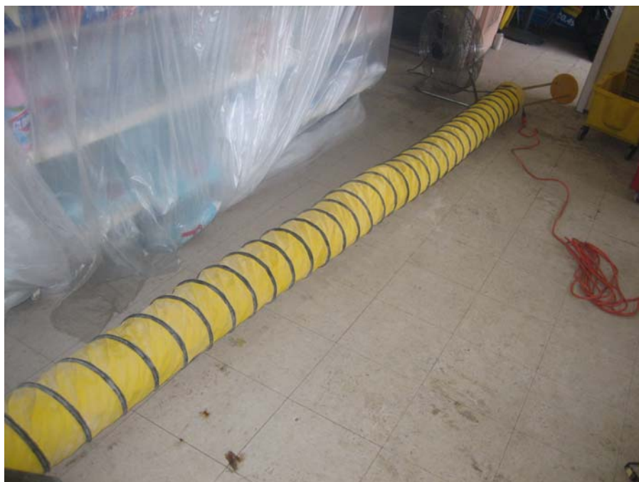
10) Directing Exhaust from the Drill Rig Operations - Mexican Store
