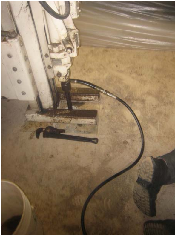
17) Hose introducing product into the geoprobe tooling
