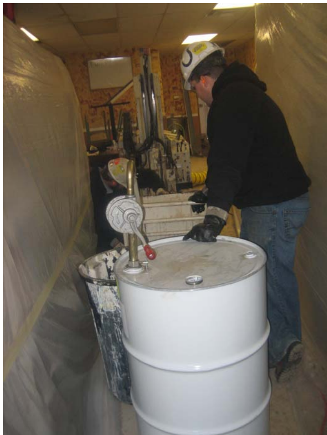
16) Hand Pump on the CAP-18 drum to pump product in the 5 gal-bucket
