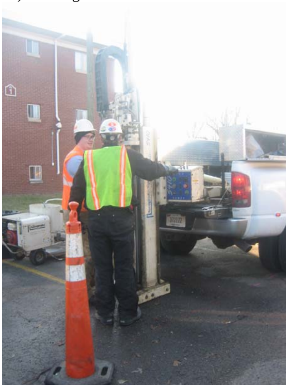
30) Injection West of Building 1
