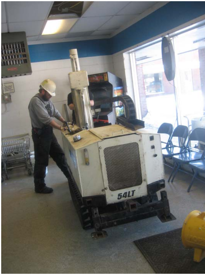
23) Drilling/Injection Location in the Laundromat
