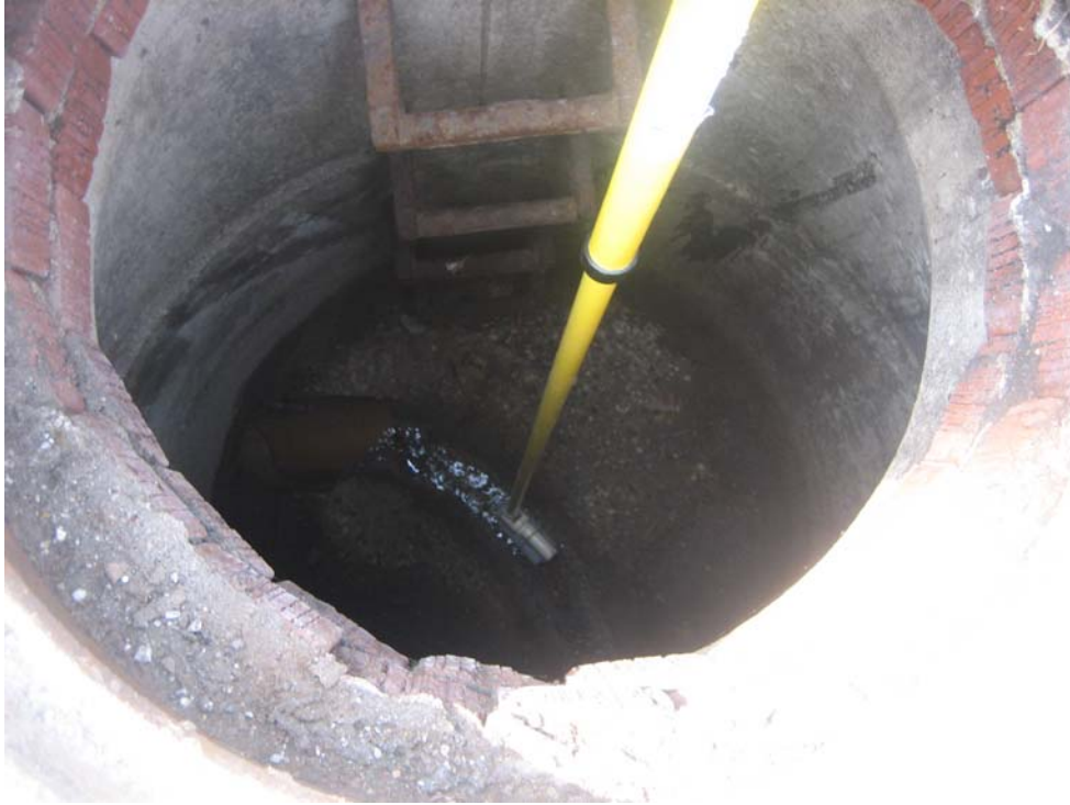
37) Sewer sampling location SS-P-01
