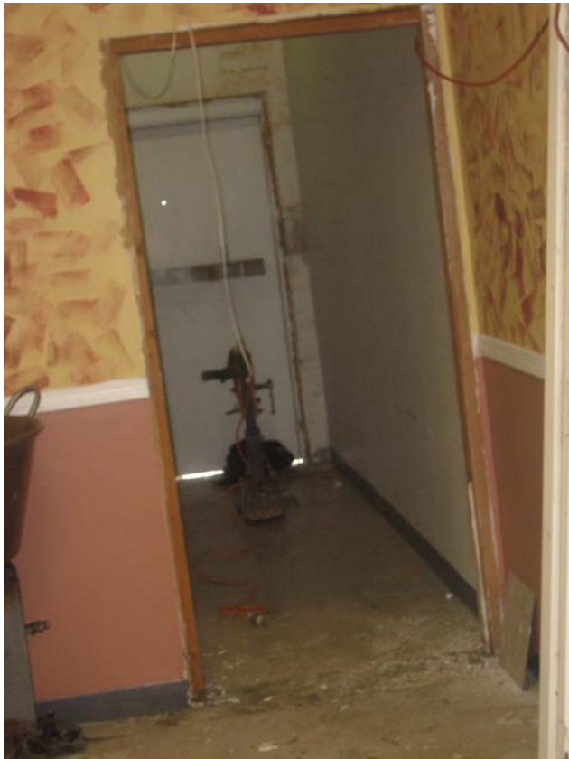
4) Mexican Store Back Door – Door & Trim taken off to enable Rig Entry
