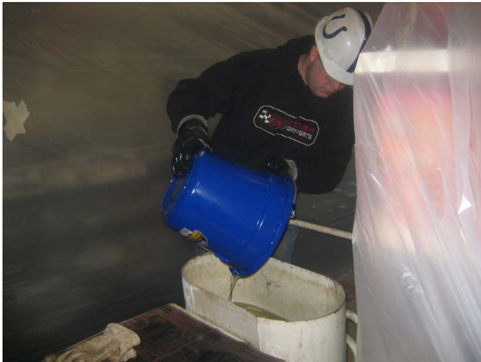
18) Measured Quantities of Product being poured into the Hopper
