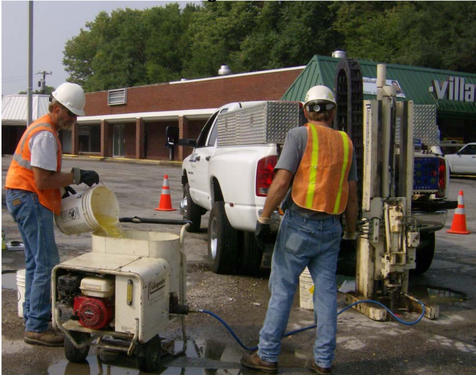
Figure 15E – Photo of CAP-18 Injection Process August 2007
