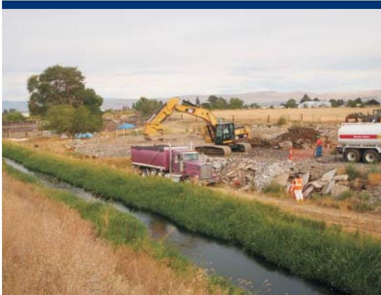
Photo 31 ERRS loads concrete debris into truck for off-site disposal.
