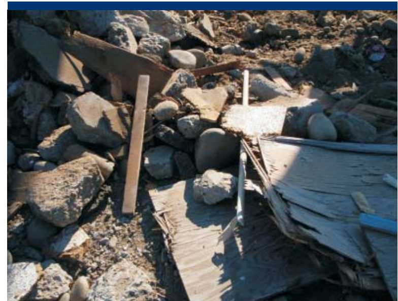
Photo 18 Debris pile with acoustical ceiling tile and wood debris.
