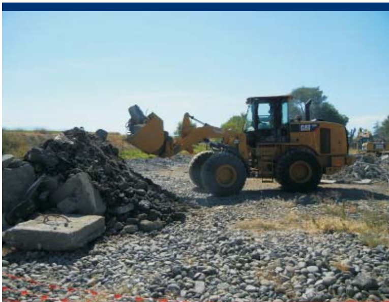
Photo 7 ERRS places concrete into stockpile in southeast quadrant.
