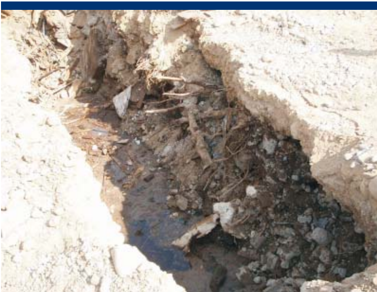
Photo 29 Interior of trench in southeast quadrant, with trash and debris in south side wall.
