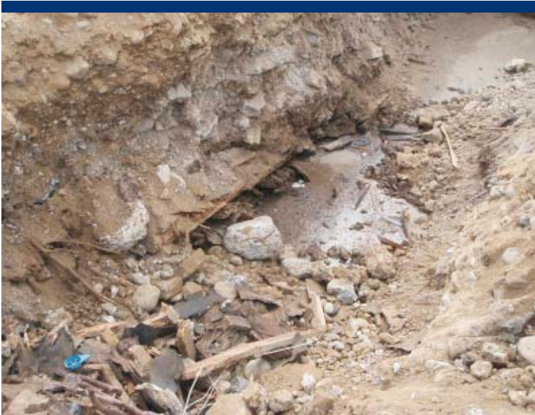
Photo 27 Groundwater and trash in bottom of trench in northeast quadrant.
