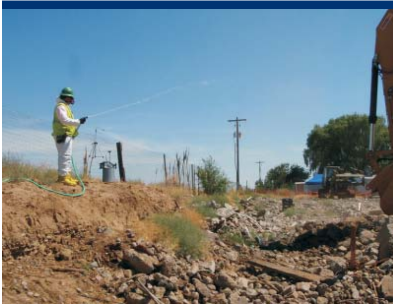
Photo 9 Water truck operator sprays water for dust control.
