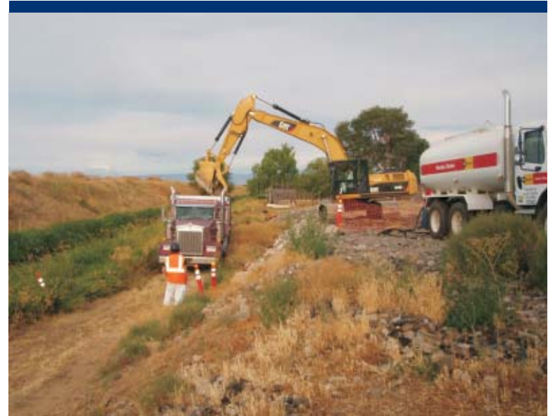
Photo 32 ERRS loads concrete debris into truck for off-site disposal.
