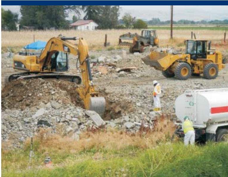
Photo 5 Excavation of a test pit in the southwest quadrant.
