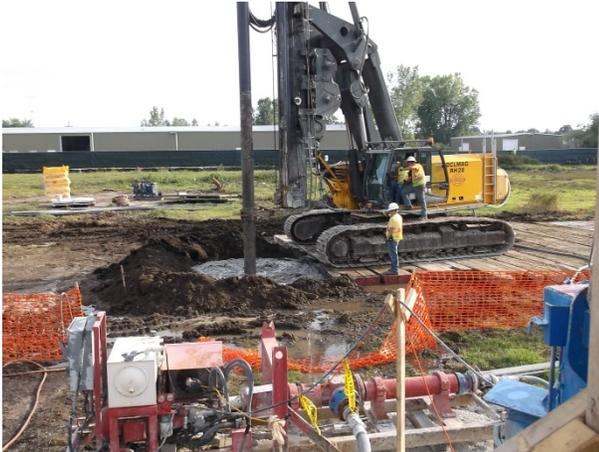
**Photo 1:** Drilling of ISS shakedown test column.
