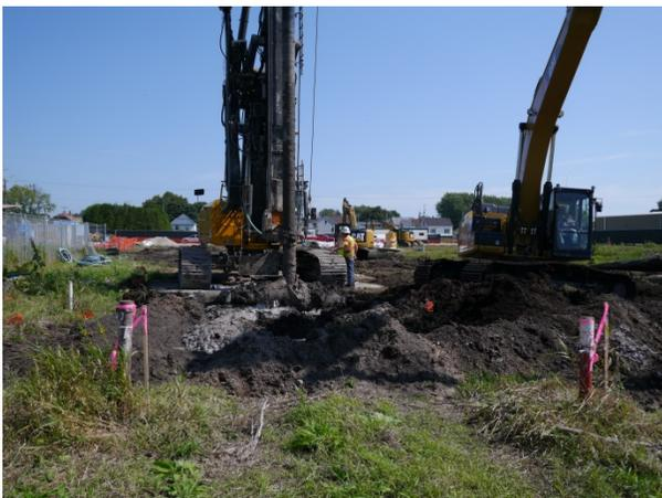
**Photo 2:** Drilling of ISS pilot test column.
