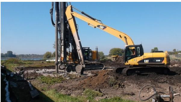
**Photo 3:** ISS drilling.
