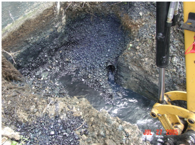
Photo Description: Drain pipe leaking liquid waste
