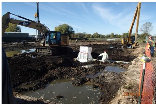
**Photo 3:** Asbestos pipe removal.
