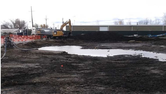
Photo 2: Ponded contact water being pumped to frac tank.
