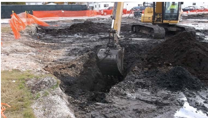
Photo 3: Excavation of peat material in the Excavation Area.
