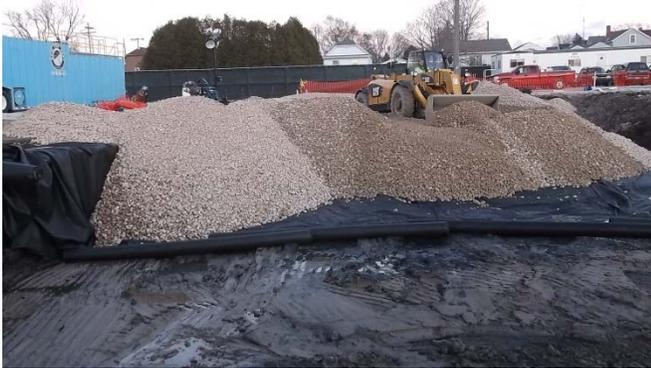
**Photo 1:** Placing filter fabric and stone backfill in the northern portion of the Excavation Area.
