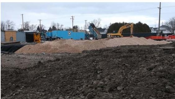
**Photo 3:** Placing stone backfill in the northern portion of the Excavation Area.
