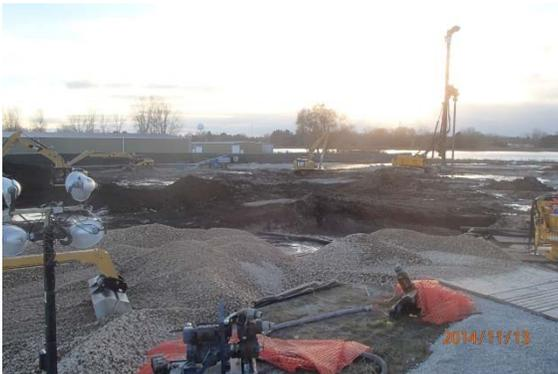
**Photo 2:** Placing stone backfill in the northern portion of the Excavation Area and ISS drilling.
