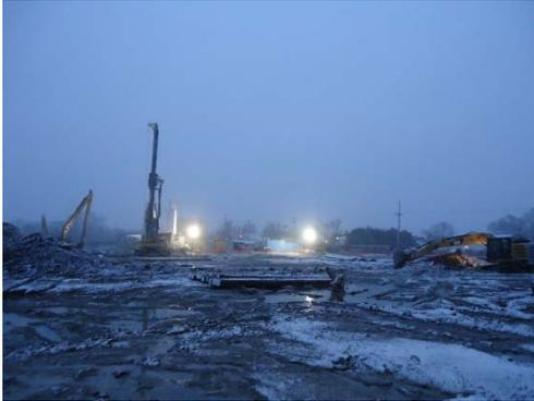
**Photo 1:** ISS drilling and peat removal in ISS Area.
