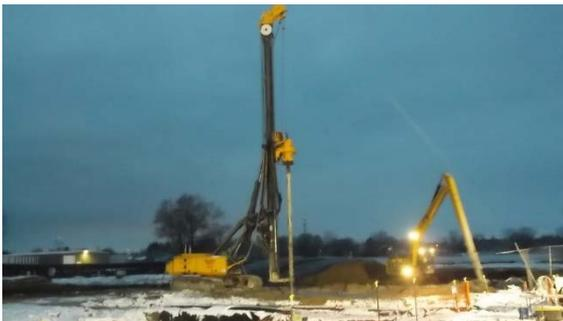
**Photo 3:** ISS drilling and covering of inactive stockpiles.
