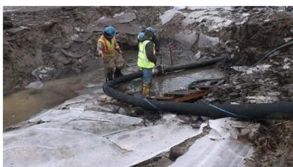
**Photo 2:** Connecting hose from WPS pipe connection to roll-off dumpster.
