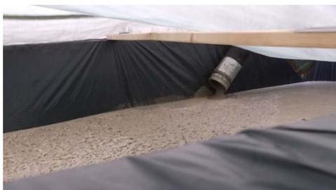
**Photo 3:** Grout from WPS pipe flowing through hose connection and into roll-off dumpster.
