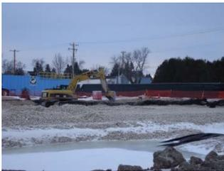
**Photo 2:** Grading stone backfill in the Excavation Area.
