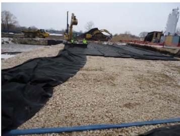
**Photo 3:** Placing filter fabric over graded stone backfill in the Excavation Area.
