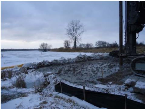
**Photo 2:** ISS drilling along the Ordinary High Water Mark of the West Twin River.
