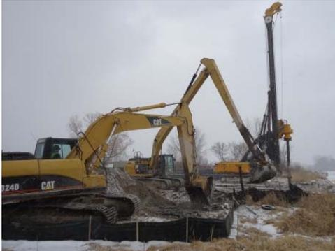
**Photo 1:** ISS drilling and test pit excavation for excavation limit sample collection in the U.S. Oil property Excavation Areas.
