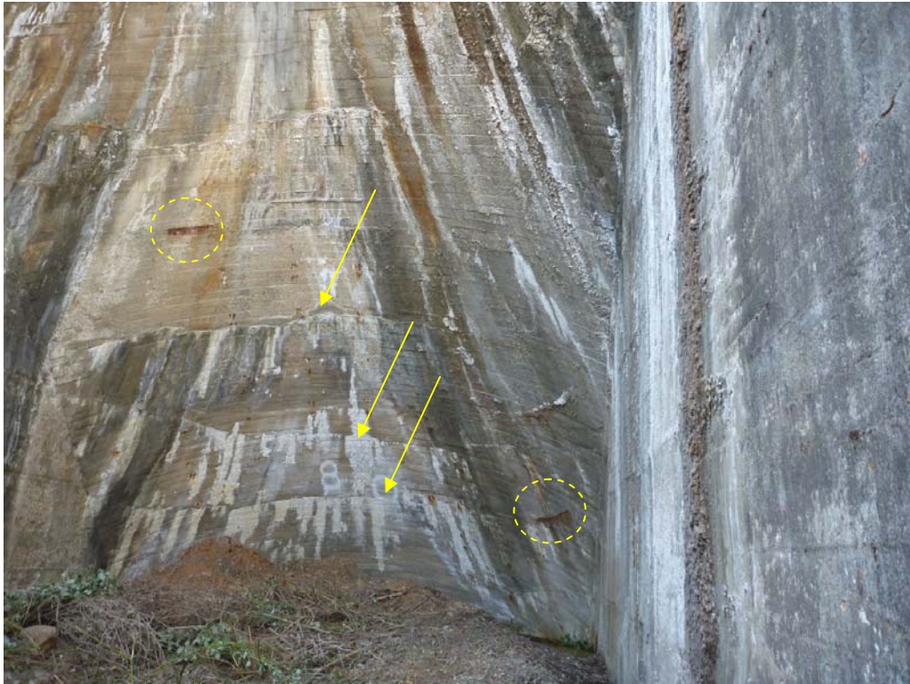
Figure 16. Corrosion of Cables within Arch #8 and Weakened Concrete Planes
