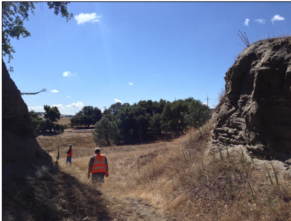
Photo 6-2. Breach at Right Abutment - Looking Downstream or Southeast (25 Sep 13)
