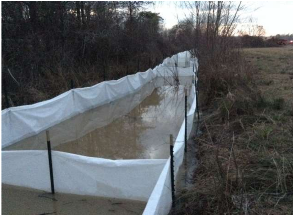
Photo 1 - Photograph of installed absorbent fence.
