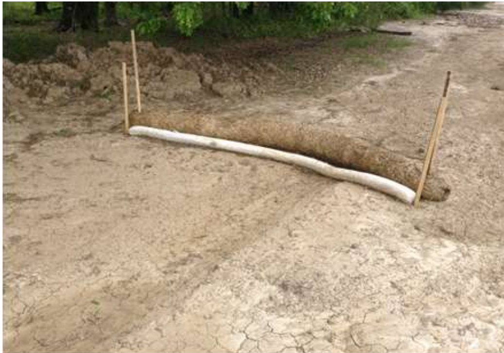
Photo 4 - Photograph of installed absorbent material and hay wattles.
