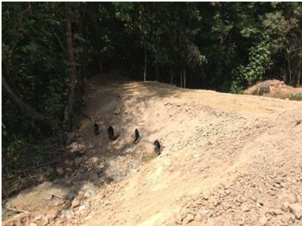
Photo 6 - Photograph of installed underflow dam.
