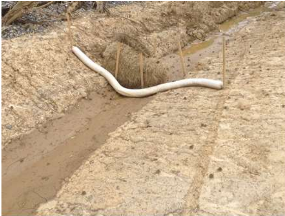
Photo 5 - Photograph of installed absorbent material and hay wattles.
