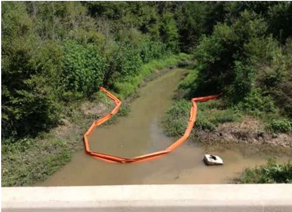
Photo 2 - Photograph of installed containment boom.
