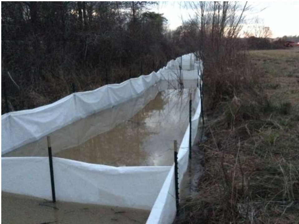
Photo 1 - Photograph of installed absorbent fence.
