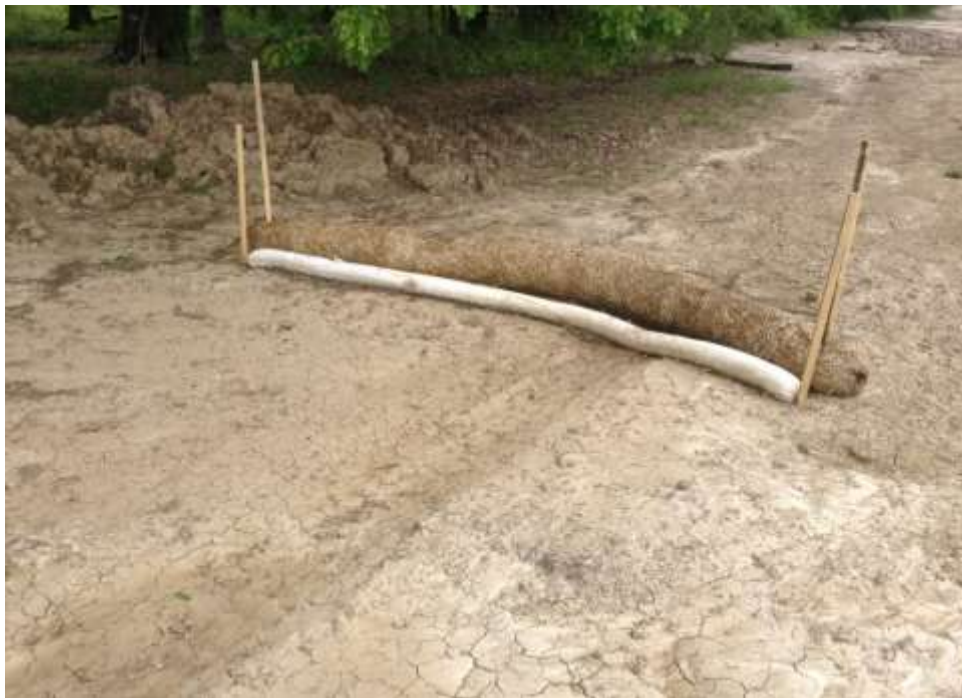
Photo 2 - Photograph of installed absorbent material and hay wattles.
