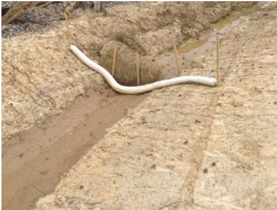
Photo 3 - Photograph of installed absorbent material and hay wattles.
