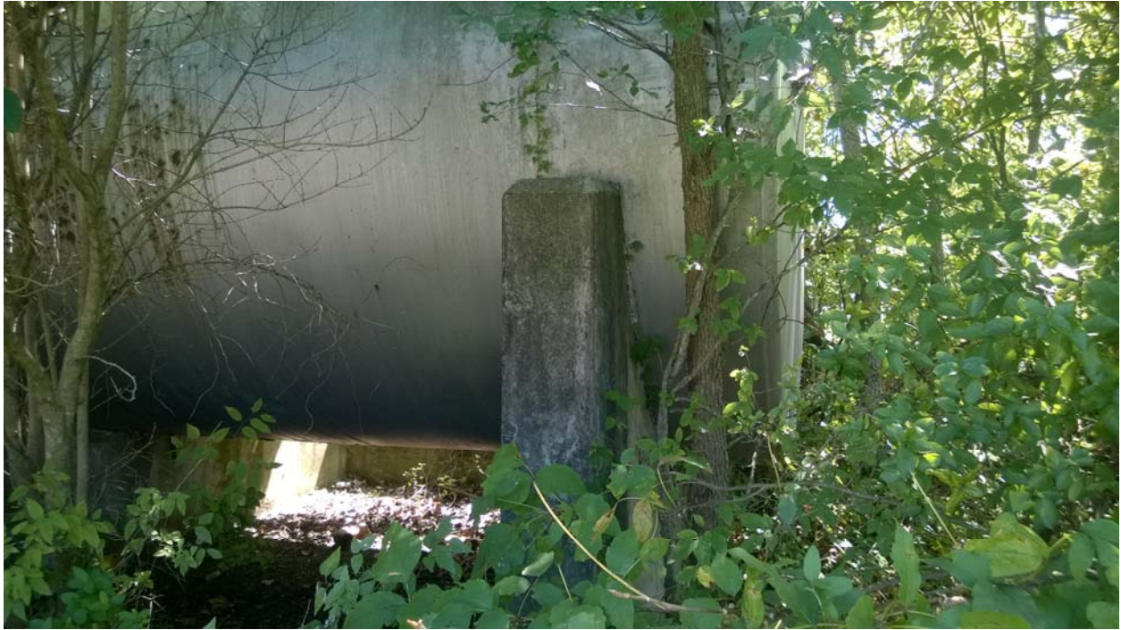
Two 25,000-gallon heating fuel oil tanks. Appears to have earthen secondary containment with concrete support. Onsite care taker states that the tanks are empty.
