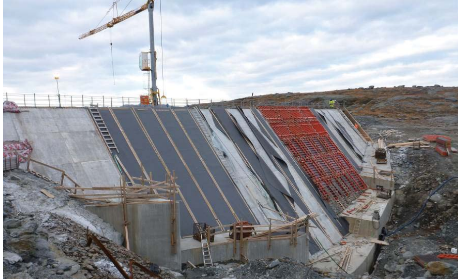
Figure 7. New slab on the upstream side with insulation of the concrete during hydration due to the cold climate in the late autumn 2014.
