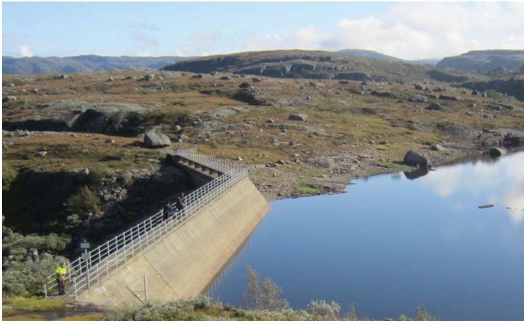
Figure 1. Dam Krokavatn. 50 m long slab buttress dam (near side) and the spillway on the far side. Notice that the dam axis has a corner on the far side between the buttress dam and the spillway.
