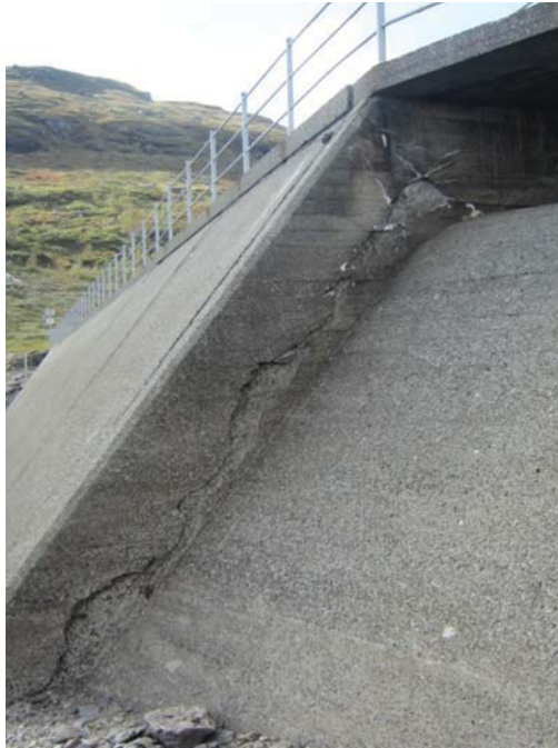
Figure 2. Cracking of concrete at the buttress wall at the corner between the spillway and the slab buttress dam, due to 15 mm expansion of the upstream slab.
