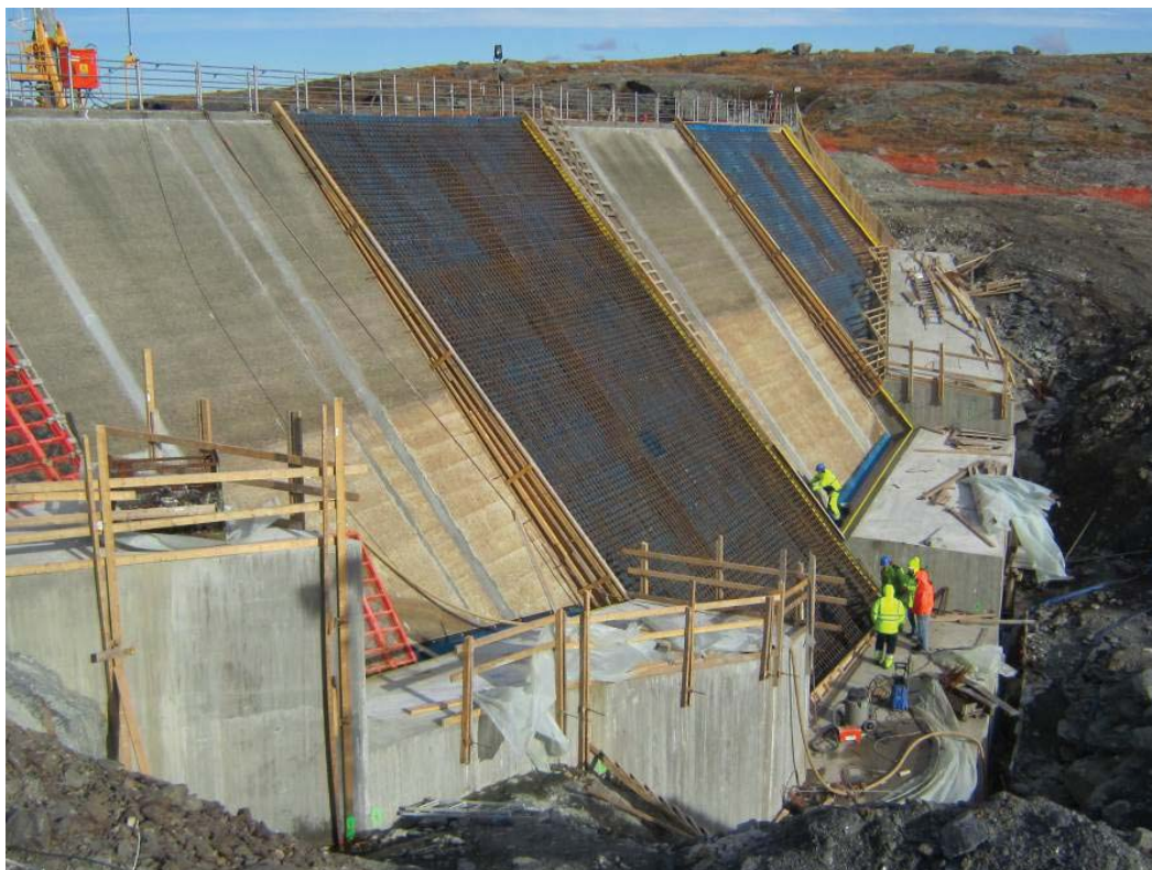
Figure 6. Reinforcement of two of the upstream slabs.
