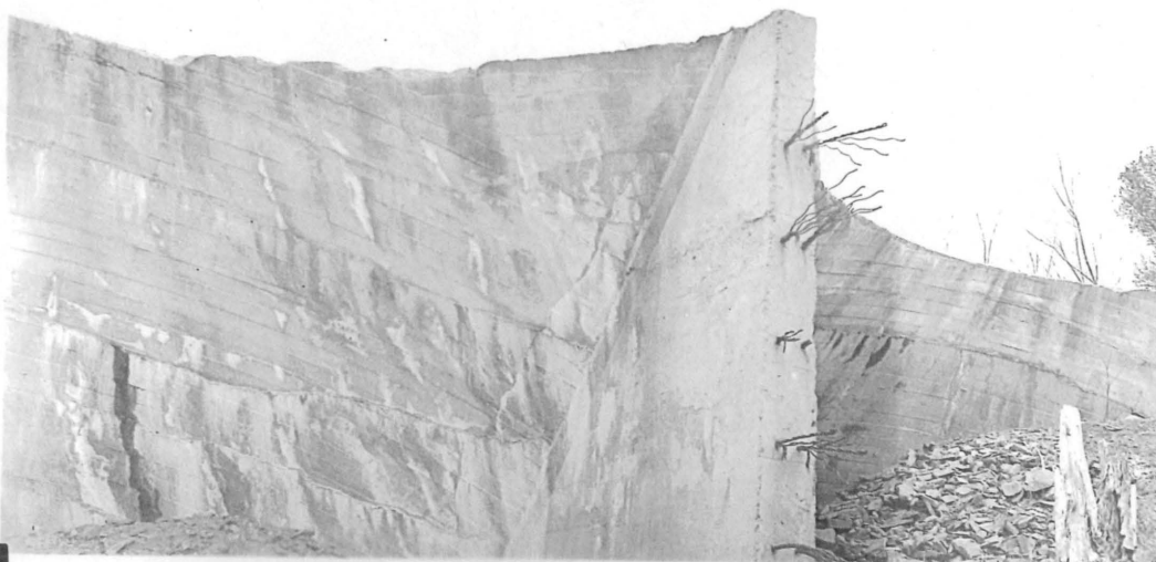
Crack at left end of arch 2-3. (Photo #2).
