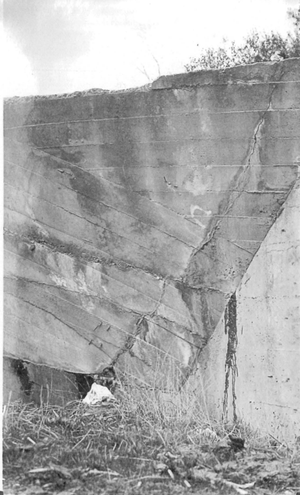
Photo #1. Crack at left end of arch 1-2.
