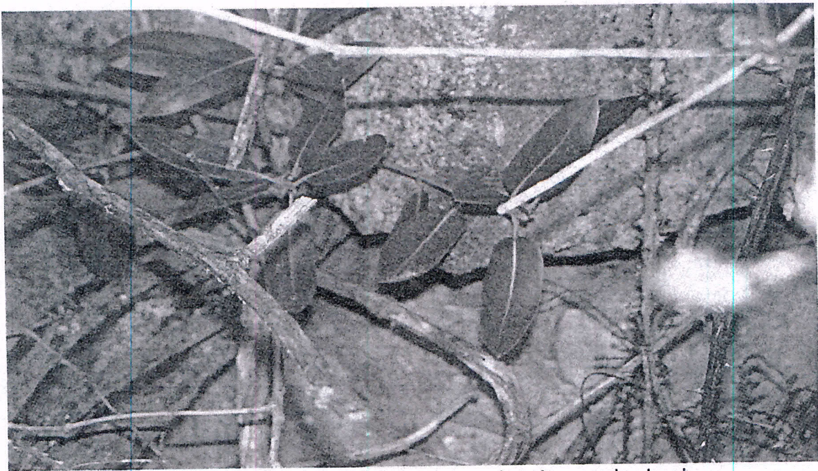
Close-up of blackberry bushes growing in cracks in dam.
