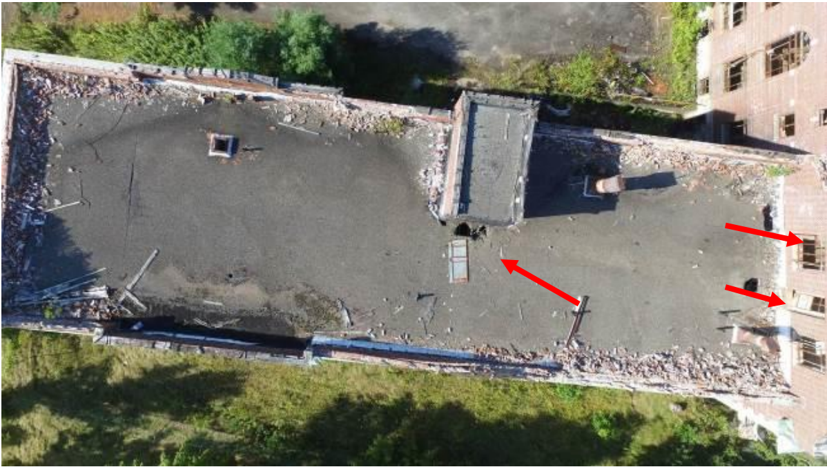
Photograph 27: Panoramic photograph of roof west of central entrance showing additional holes in roof.
