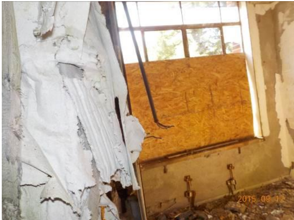
Photograph 36: The same room where sample P001-BA-030 was collected. There is an abundant amount of deteriorated pipe wrap in the room and a partially boarded up window.
