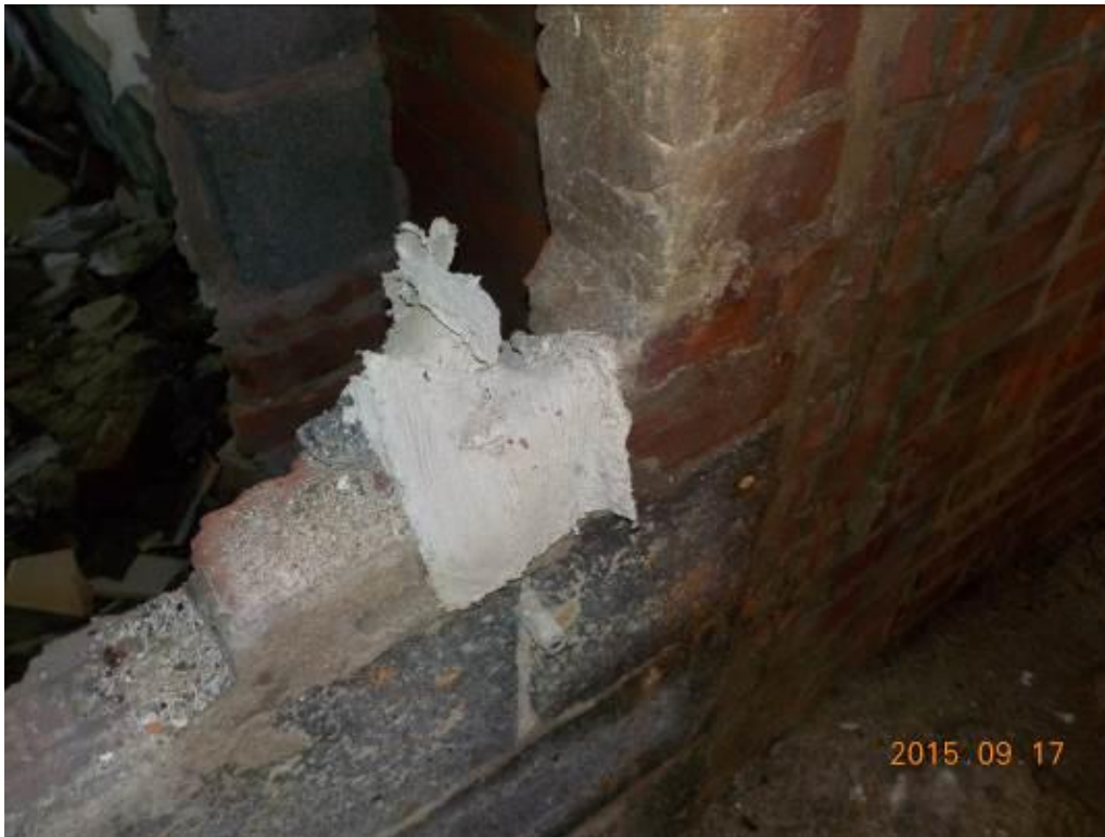
Photograph 28: Location P001-BA-022. The sample was collected from pipe wrap fallen onto partially collapsed wall. Analytical results indicate that the sample contains 50.00% chrysotile asbestos.
