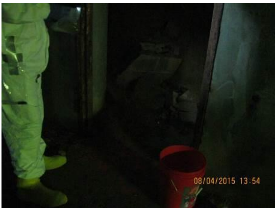
Photograph 8: Location P001-BA-008 in west wing basement. The sample was collected from a debris pile on floor. Analytical results indicate that the sample contains 4.82% chrysotile asbestos.
