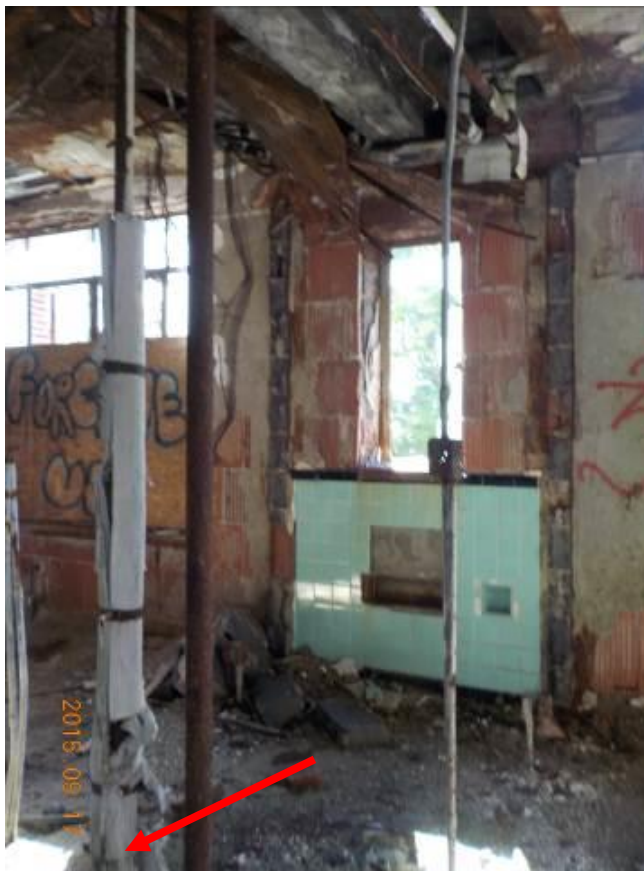
Photograph 31: Location P001-BA-026. The sample was collected from deteriorated pipe wrap on vertical pipe. Broken, opened window in background. Analytical results indicate that the sample contains 66.70% chrysotile asbestos.
