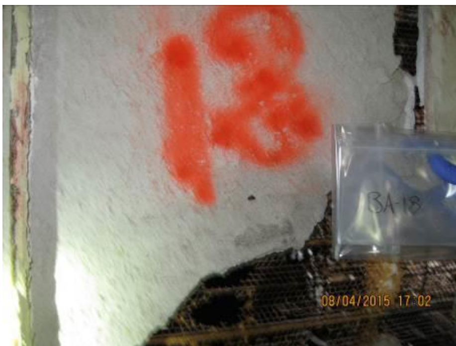
Photograph 18: Location P001-BA-018 in west wing first floor. The sample was collected from degrading drywall. Analytical results indicate that the sample was non-detect for asbestos.
