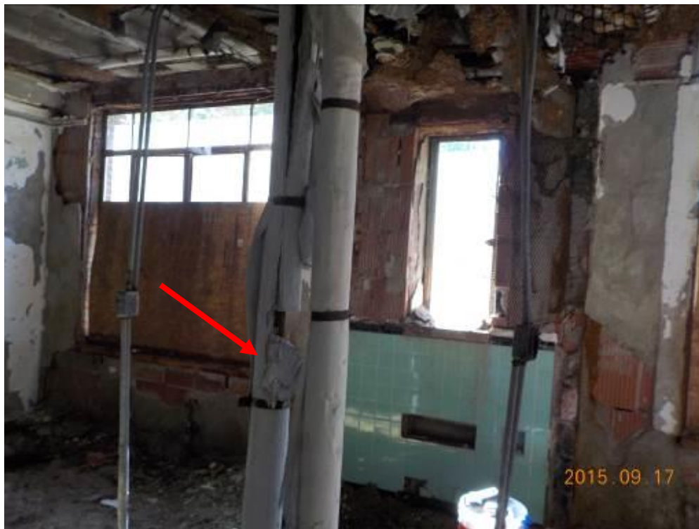
Photograph 30: Location P001-BA-025. The sample was collected from deteriorated pipe wrap on vertical pipe. Analytical results indicate that the sample contains 57.10% chrysotile asbestos.
