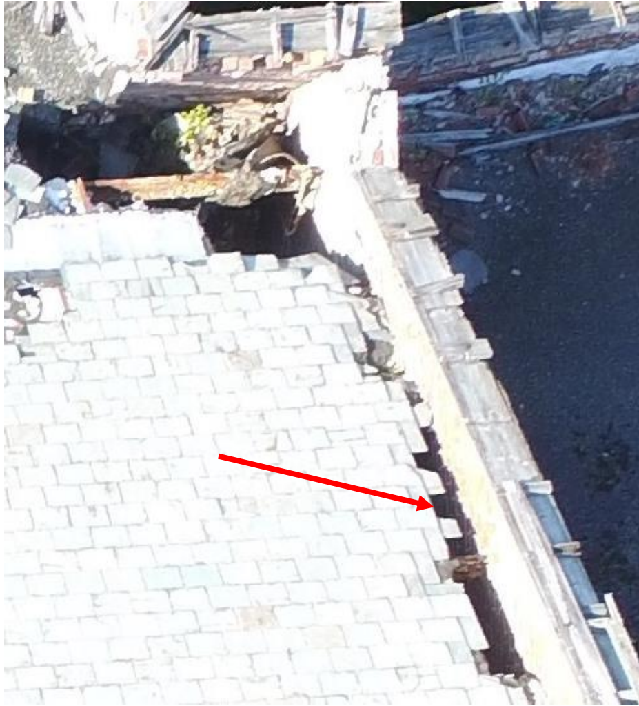
Photograph 25: Close-up of Photograph 24 showing possible parting of roof from east wall.
