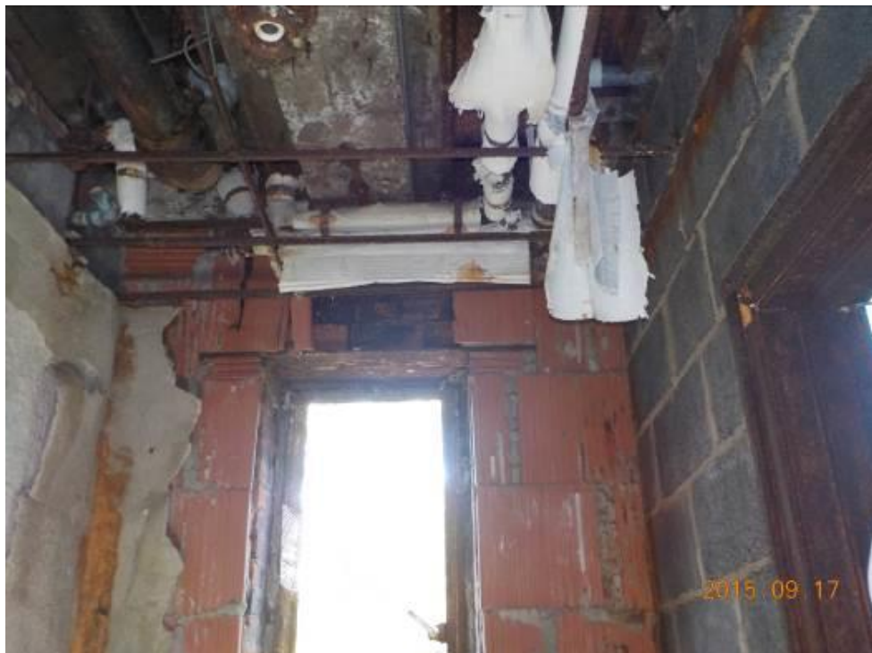
Photograph 38: The same room where sample P001-BA-031 was collected. There is an abundant amount of deteriorated pipe wrap in the room.
