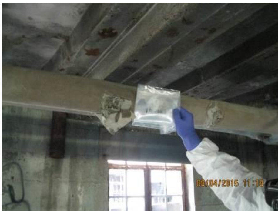
Photograph 2: Location P001-BA-002 in the west wing basement. The sample was collected from pipe insulation. Analytical results indicate that the sample contains 57.10% chrysotile asbestos.
