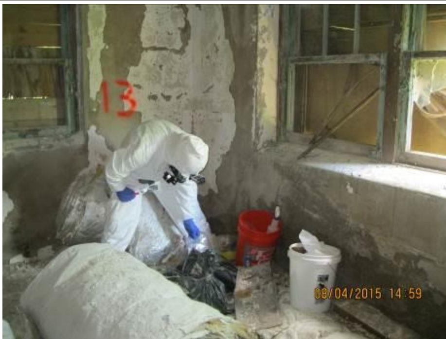
Photograph 13: Location P001-BA-013 in east wing basement. The sample was collected from “Asbestos” labeled poly trash bag. Analytical results indicate that the sample contains 19.10% chrysotile asbestos.
