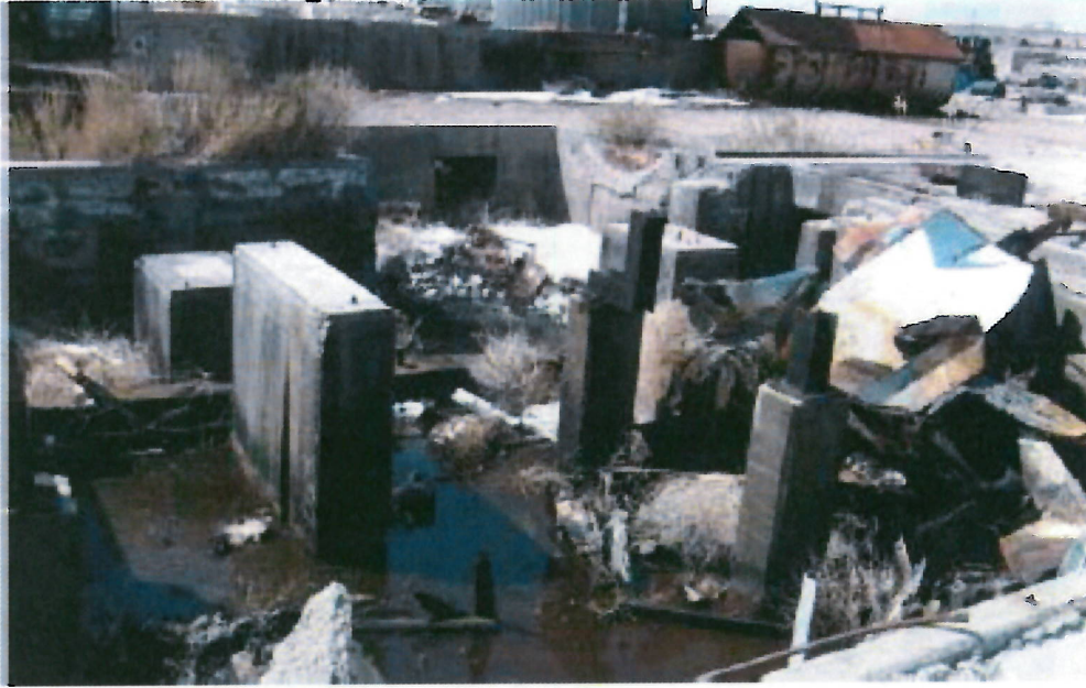
Vault under the building that housed a portion of the retort vessel. Vessel rested on the shorter concrete pylons at left center and center frame. Water results are represented by CTSW02.
