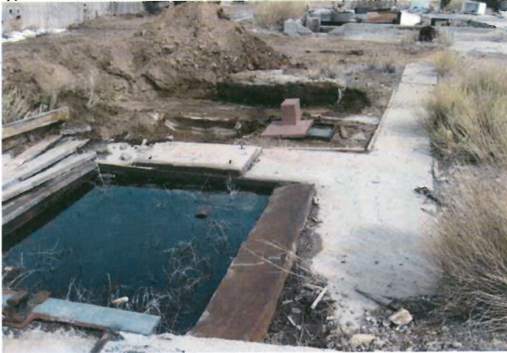
Test Pit 12. Near pit is the sump where the retort tank drained when opened. The primary drip pad extends behind the photographer. The retort vessel extended through the notch in the foundation onto the pylons shown in the previous photo.
