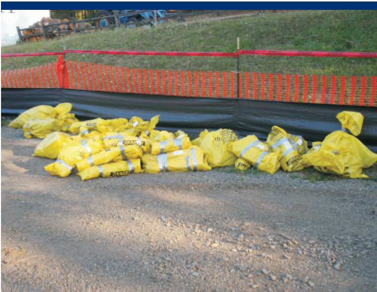
Photo 16 Bagged asbestos-cement pipe (ACP) staged at 291 118th St.
