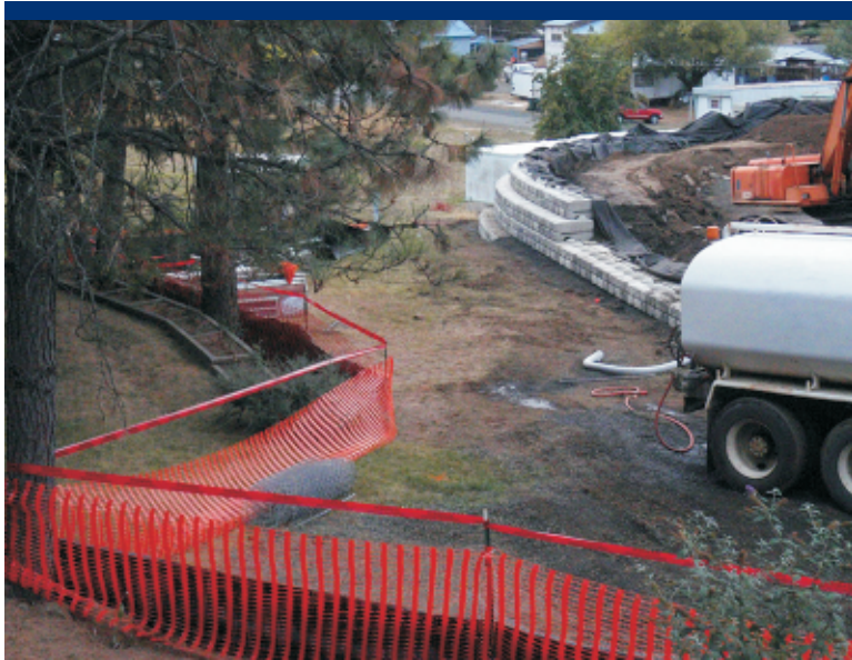
Photo 22 South terminal end of the retaining wall under construction.
