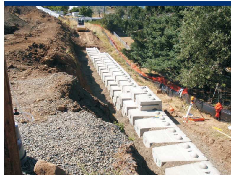
Photo 17 Base blocks of the wall for the north side of the parking lot retaining wall.
