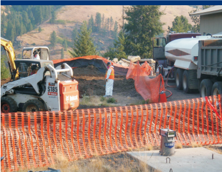
Photo 5 Excavation of asbestos-contaminated soil from 4753 Transfer Station Road.
