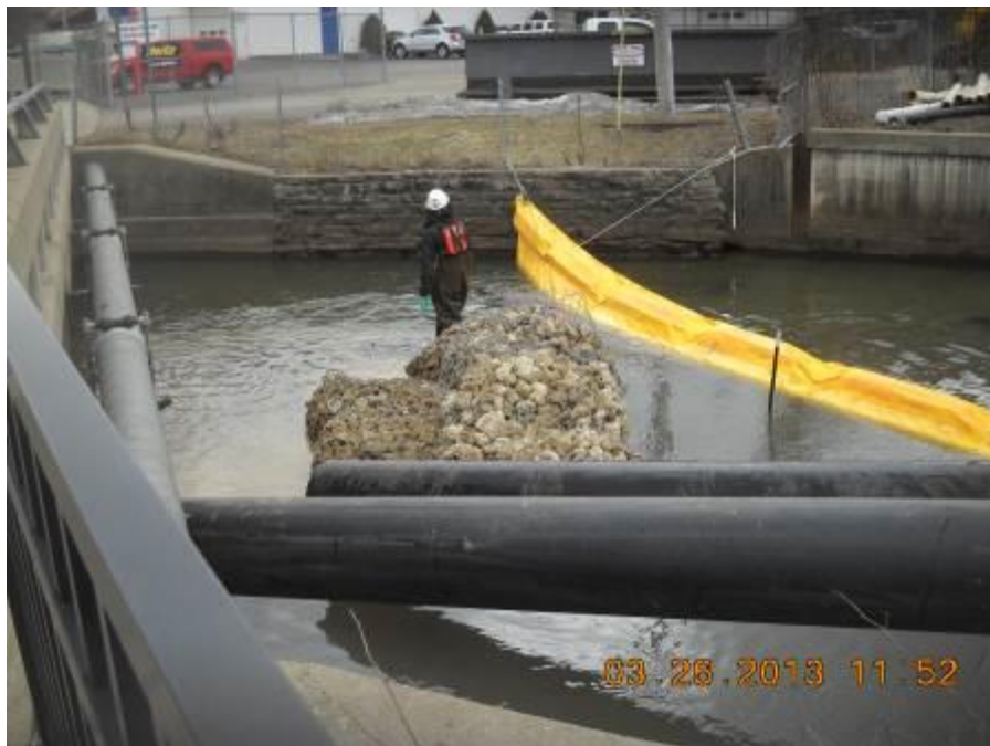
Site: Portage Creek Area Site – SA5-A Photograph No.: 12 Direction: East Subject: Placement of gabion baskets at the northern end
