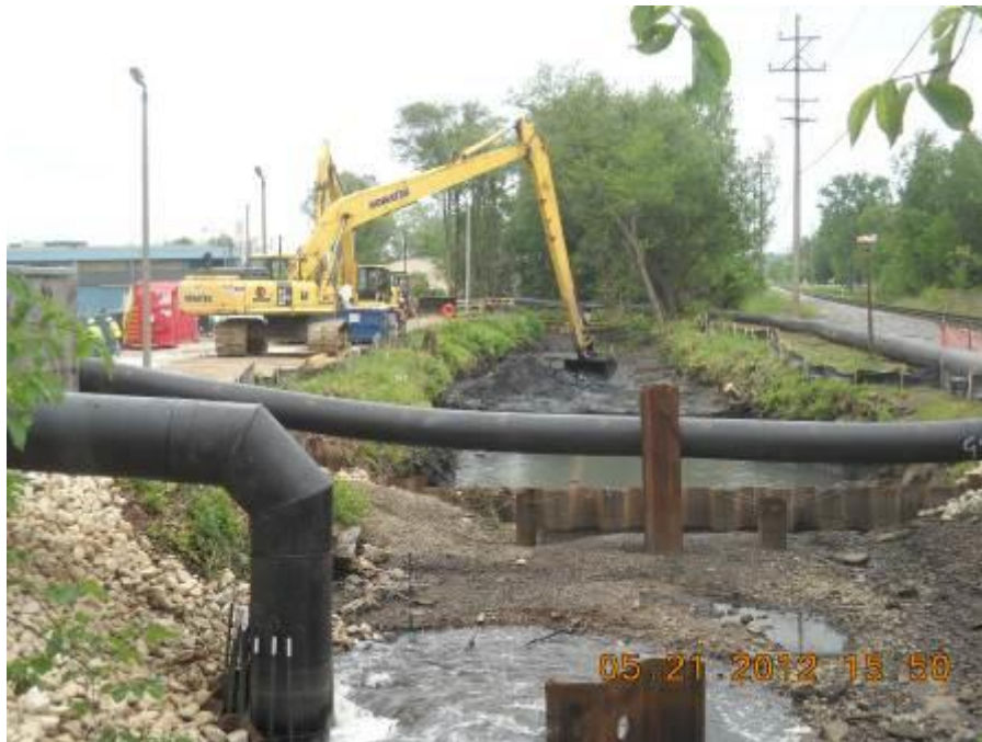
Site: Portage Creek Area Site – SA6 Photograph No.: 21 Direction: South Subject: Excavation of sediment from Grid 2
