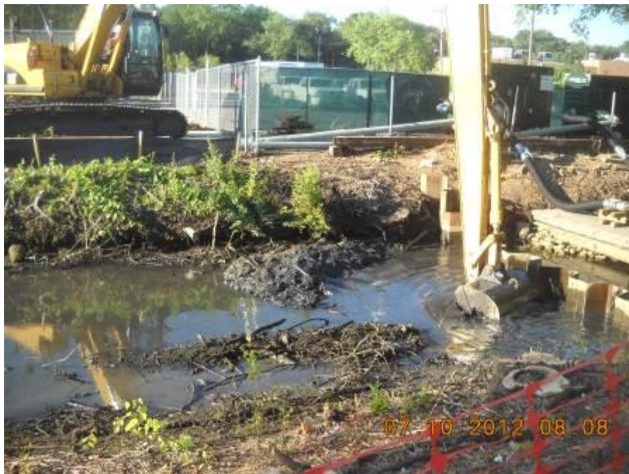
Site: Portage Creek Area Site – Axtell Creek Photograph No.: 6 Direction: Southwest Subject: Excavation of contaminated sediment
