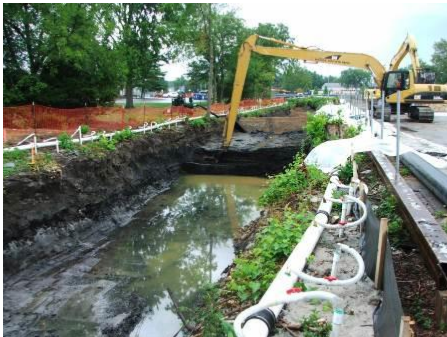
Site: Portage Creek Area Site – Axtell Creek Photograph No.: 18 Direction: East Subject: Further excavation of sediment from Grids 1 and 2
