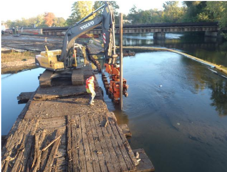
Site: Allied Portage Creek Slope Area - SA1-A Photograph No.: 16 Direction: North Subject: Removal of downstream sheet-pile cofferdam
