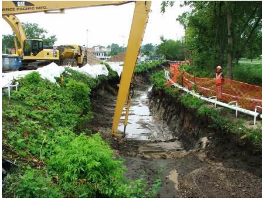
Site: Portage Creek Area Site – Axtell Creek Photograph No.: 21 Direction: West Subject: Excavation of contaminated sediment
