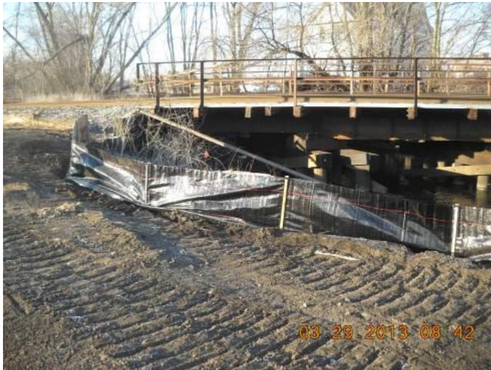
Site: Portage Creek Area Site - SA3-A Photograph No.: 3 Direction: West Subject: Silt fence installed along southern bank
