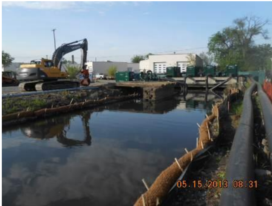
Site: Portage Creek Area Site – SA5-A Photograph No.: 23 Direction: South Subject: Removal of the south cofferdam
