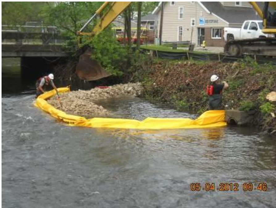
Site: Portage Creek Area Site – SA6 Photograph No.: 8 Direction: Southwest Subject: Installation of a sediment curtain prior to the installation of the concrete catch basin
