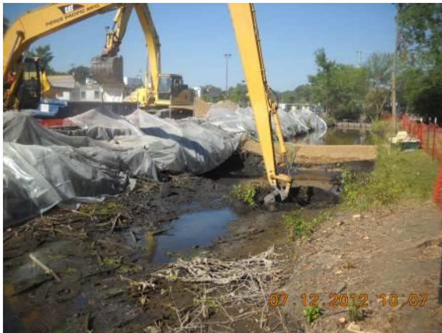
Site: Portage Creek Area Site – Axtell Creek Photograph No.: 10 Direction: Southwest Subject: Excavation of contaminated sediment
