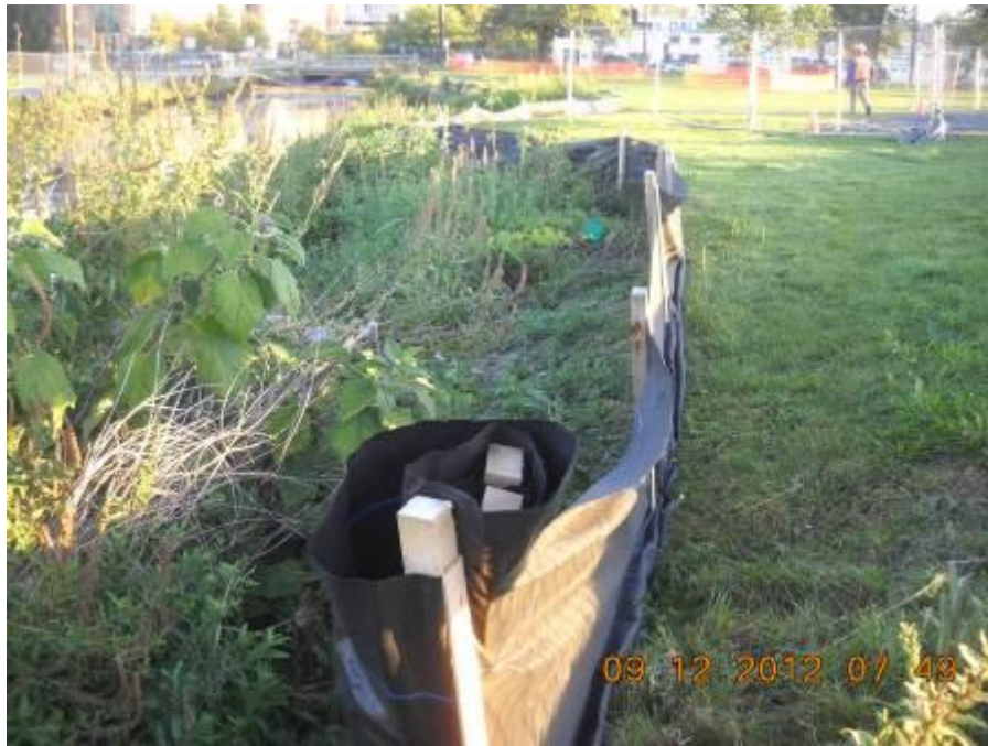
Site: Portage Creek Area Site – SA5-C Photograph No.: 5 Direction: North Subject: Silt fencing along the east bank
