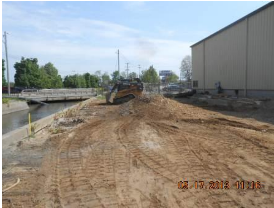
Site: Portage Creek Area Site – SA5-A Photograph No.: 27 Direction: North Subject: Re-grading eastern bank at north end
