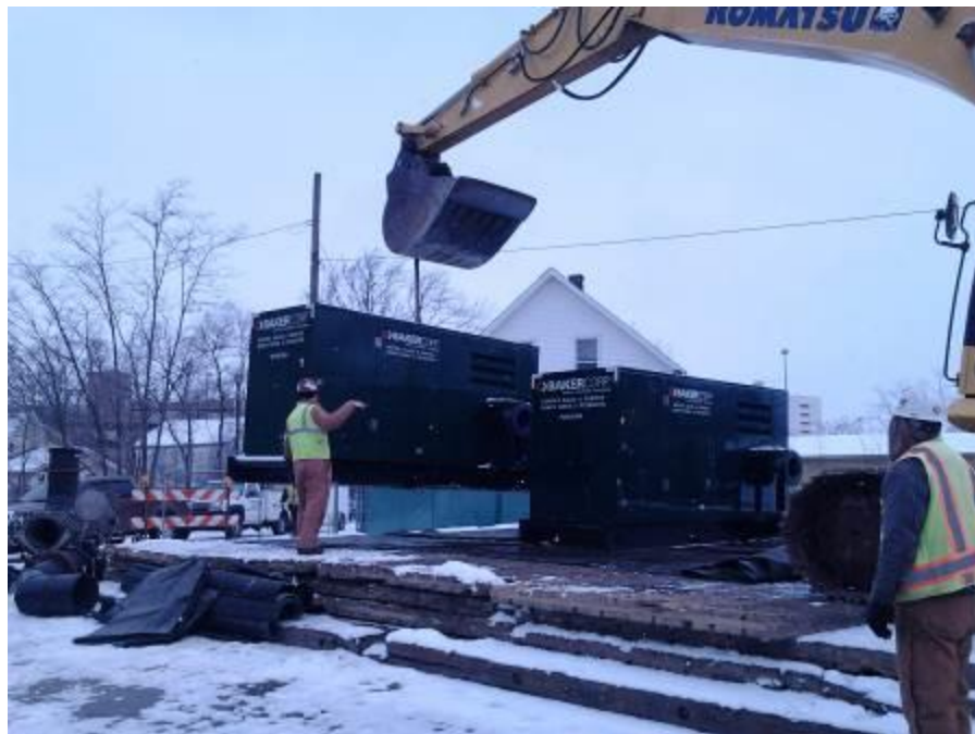
Site: Portage Creek Area Site – SA5-A Photograph No.: 8 Direction: West Subject: Placement of bypass pumps
