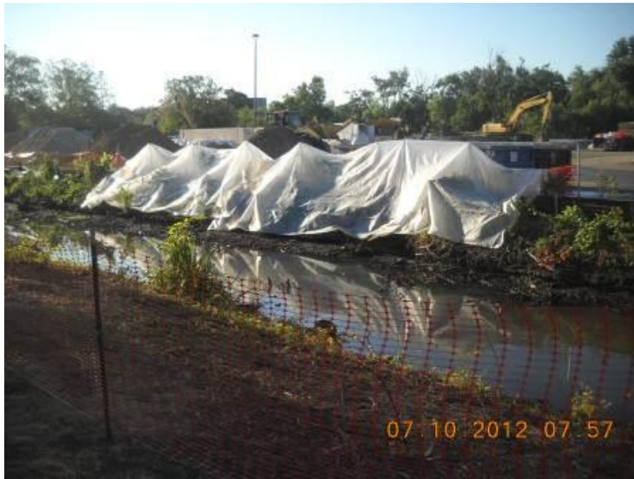
Site: Portage Creek Area Site – Axtell Creek Photograph No.: 5 Direction: Southeast Subject: Polyethylene sheeting laid along the bank
