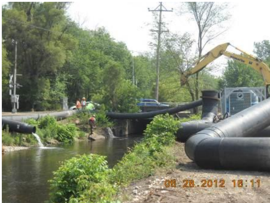
Site: Portage Creek Area Site – SA6 Photograph No.: 34 Direction: Southeast Subject: Disassembly of the surface water bypass system
