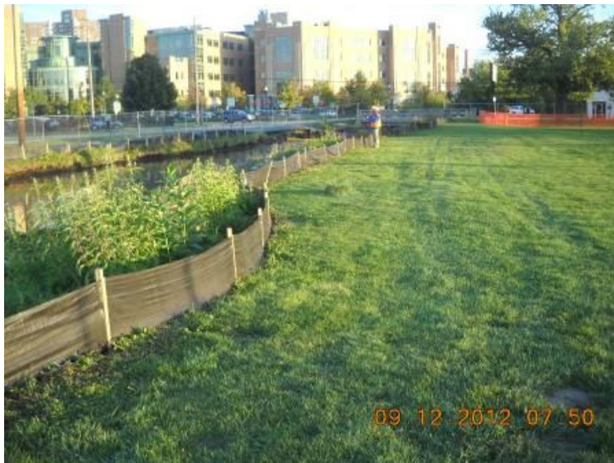
Site: Portage Creek Area Site – SA5-C Photograph No.: 6 Direction: North Subject: Silt fencing installed along the east bank
