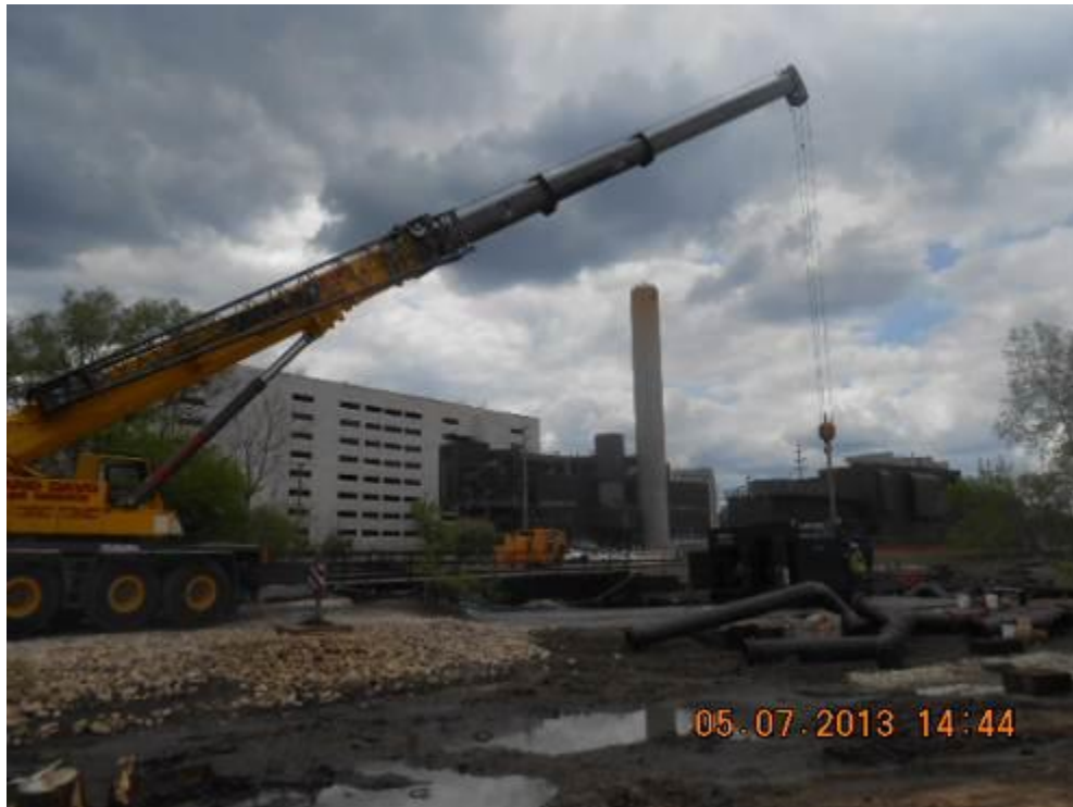
Site: Portage Creek Area Site - SA3-A Photograph No.: 7 Direction: Northwest Subject: Crane lifting the bypass pumps into place
