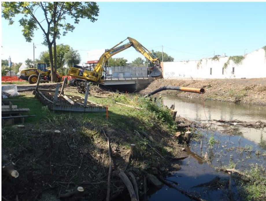
Site: Portage Creek Area Site - SA1-A Photograph No.: 6 Direction: South Subject: Discharge piping installation
