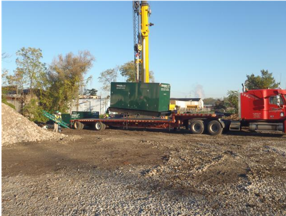
Site: Portage Creek Area Site - SA1-A Photograph No.: 17 Direction: North Subject: Removal of bypass pumps
