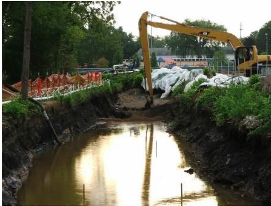
Site: Portage Creek Area Site – Axtell Creek Photograph No.: 19 Direction: East Subject: Excavation of contaminated sediment
