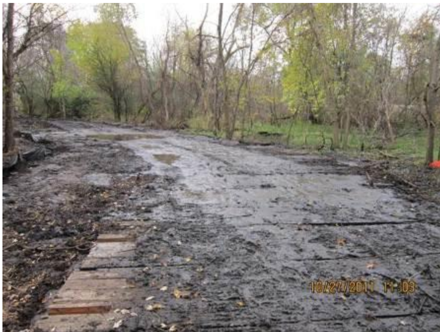
Site: Portage Creek Area Site – SA7 Photograph No.: 12 Direction: South Subject: Access road timber mats underwater
