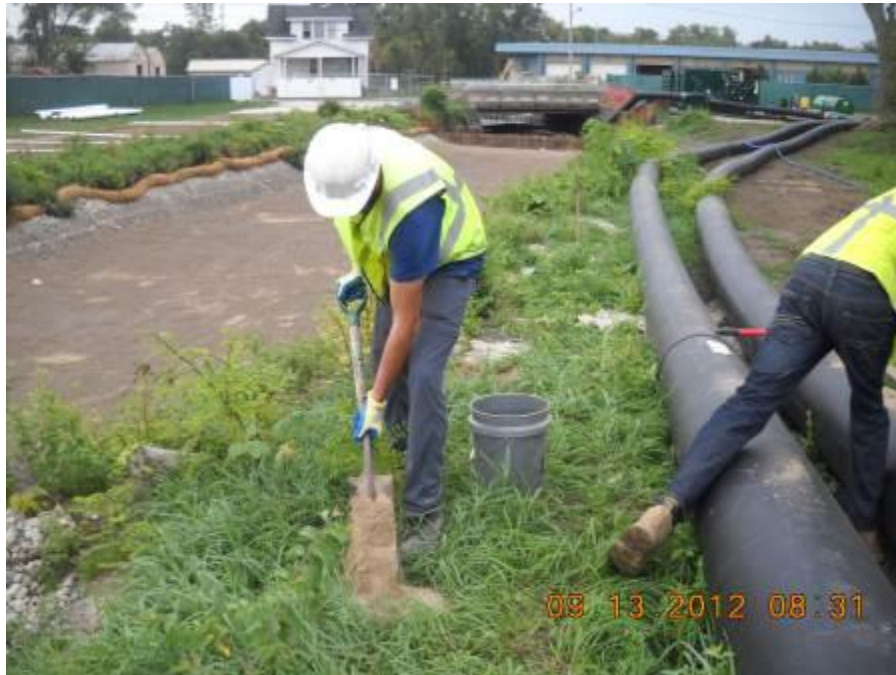
Site: Portage Creek Area Site – SA5-D Photograph No.: 23 Direction: South Subject: Re-filling sipper well hole on east bank
