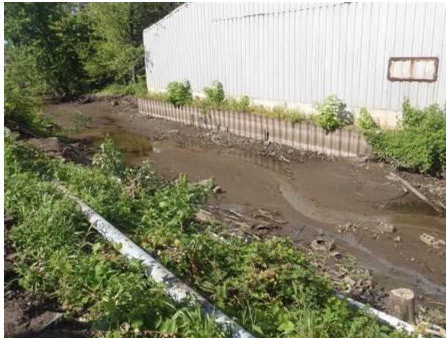
Site: Portage Creek Area Site - SA1-C and SA1-B Photograph No.: 18 Direction: South Subject: Dewatering of Grid 4 in SA1-B
