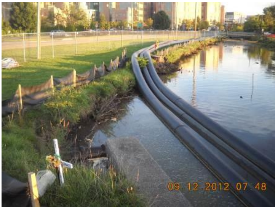
Site: Portage Creek Area Site – SA5-C Photograph No.: 4 Direction: North Subject: Silt fencing along the west bank
