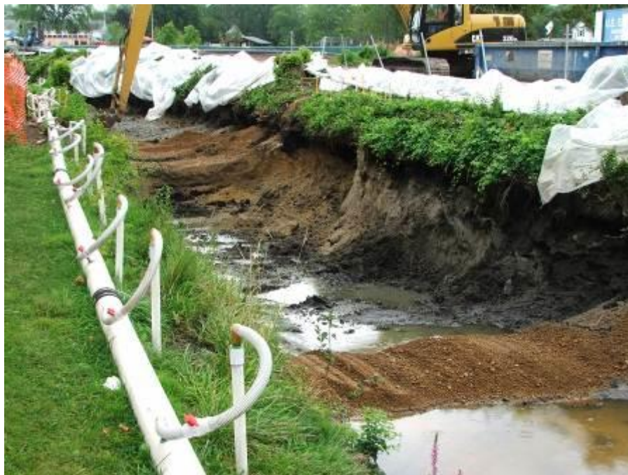
Site: Portage Creek Area Site – Axtell Creek Photograph No.: 20 Direction: Southeast Subject: Excavation of contaminated sediment
