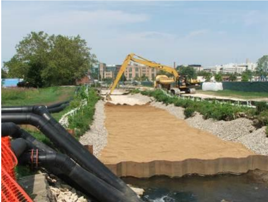
Site: Portage Creek Area Site – SA5-D Photograph No.: 17 Direction: North Subject: Placement of sand/gravel mix
