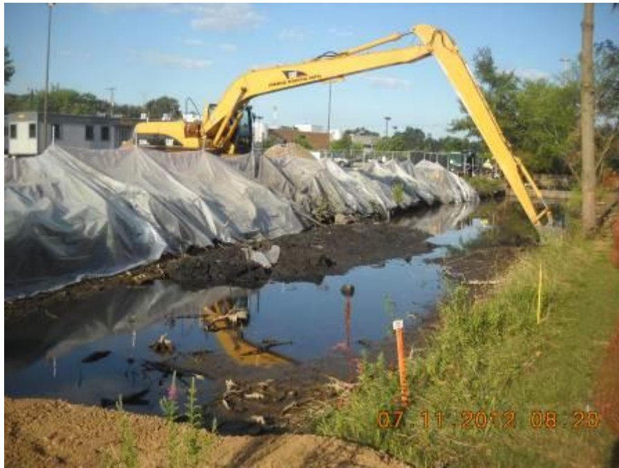
Site: Portage Creek Area Site – Axtell Creek Photograph No.: 9 Direction: Southwest Subject: Excavation of contaminated sediment
