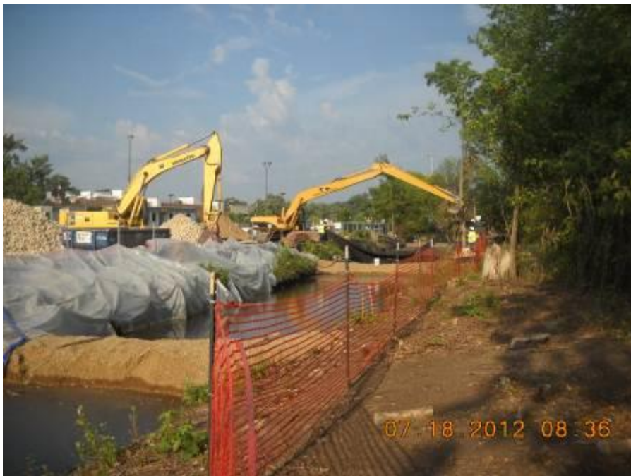
Site: Portage Creek Area Site – Axtell Creek Photograph No.: 12 Direction: Southwest Subject: Excavation of contaminated sediment
