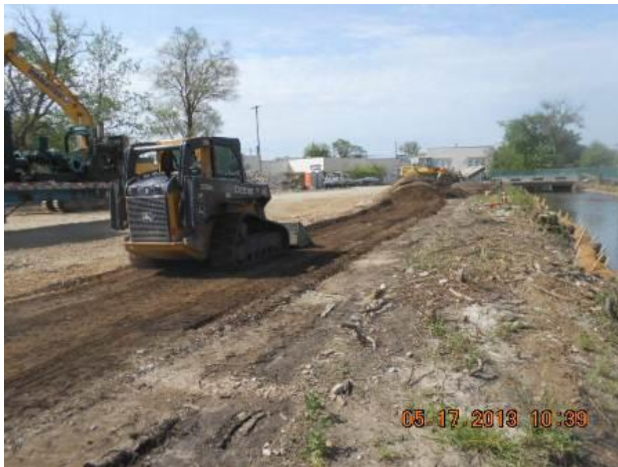
Site: Portage Creek Area Site – SA5-A Photograph No.: 26 Direction: South Subject: Leveling eastern bank
