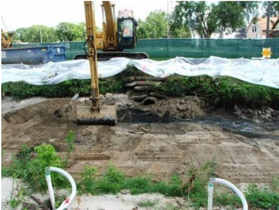
Site: Portage Creek Area Site – SA5-D Photograph No.: 5 Direction: East Subject: Excavating contaminated sediment
