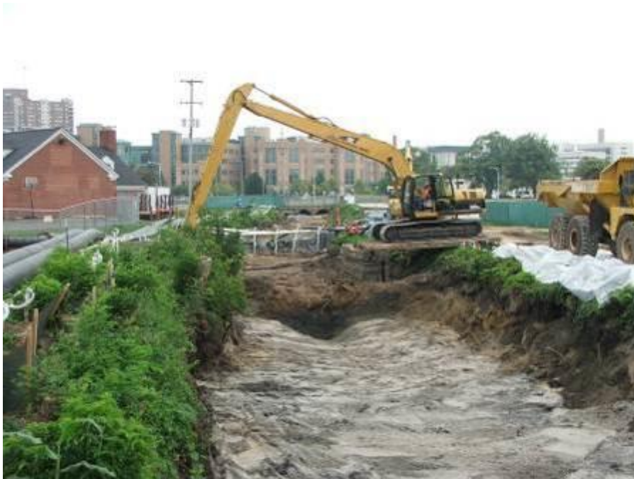
Site: Portage Creek Area Site – SA5-D Photograph No.: 18 Direction: North Subject: Excavation of contaminated sediments
