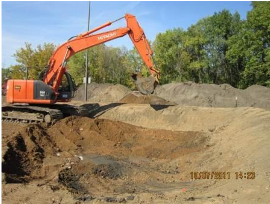
Site: Portage Creek Area Site Photograph No.: 13 Direction: North Subject: Excavation for sump in staging area
