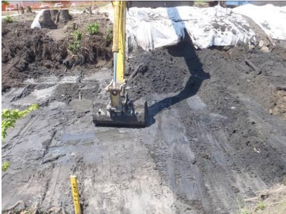
Site: Portage Creek Area Site - SA3-A Photograph No.: 13 Direction: NA Subject: Grid 2 showing gray contamination layer
