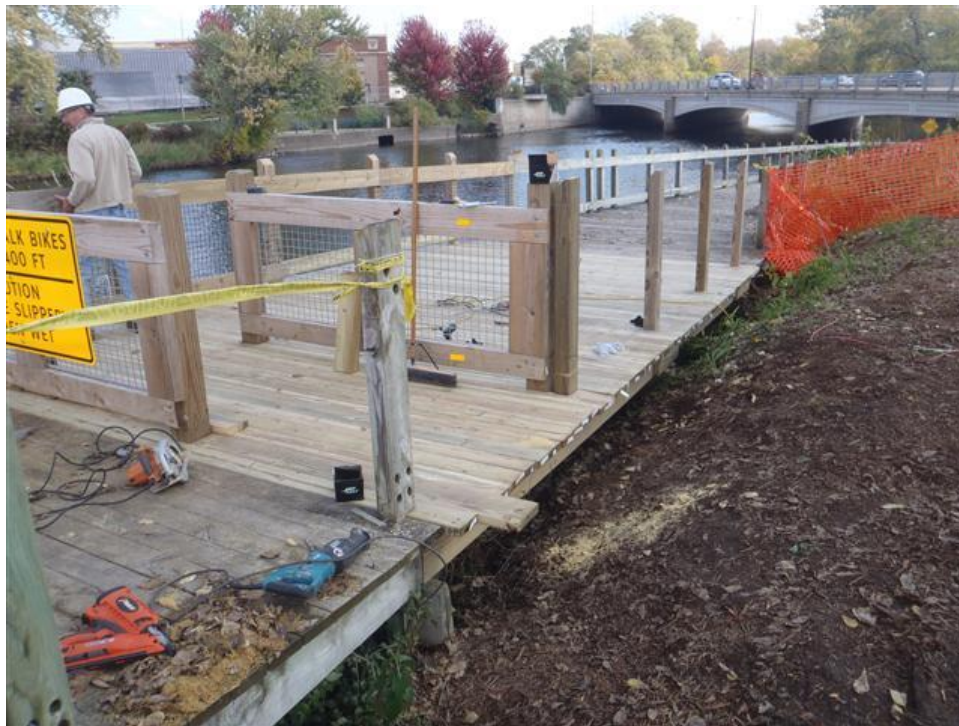
Site: Portage Creek Area Site - SA1-A Photograph No.: 20 Direction: Southeast Subject: Reconstruction of city boardwalk
