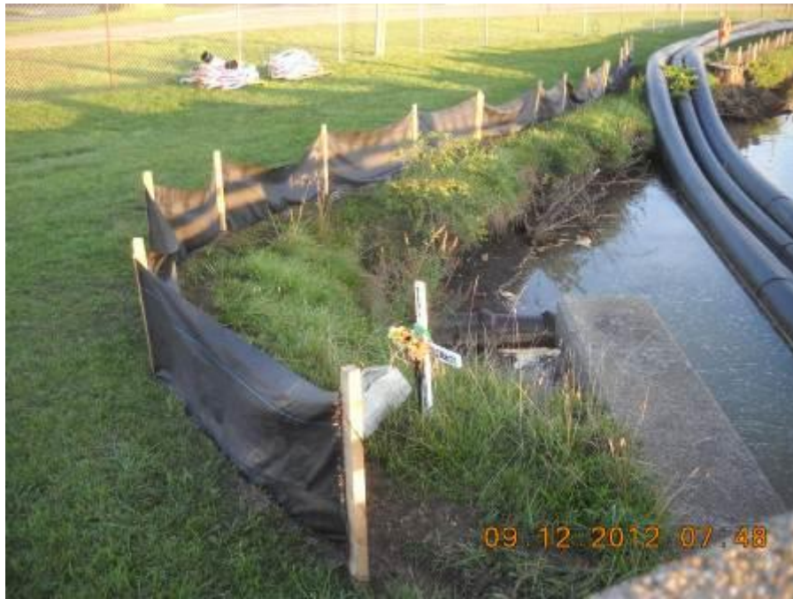
Site: Portage Creek Area Site – SA5-C Photograph No.: 3 Direction: Northwest Subject: Silt fencing along the west bank
