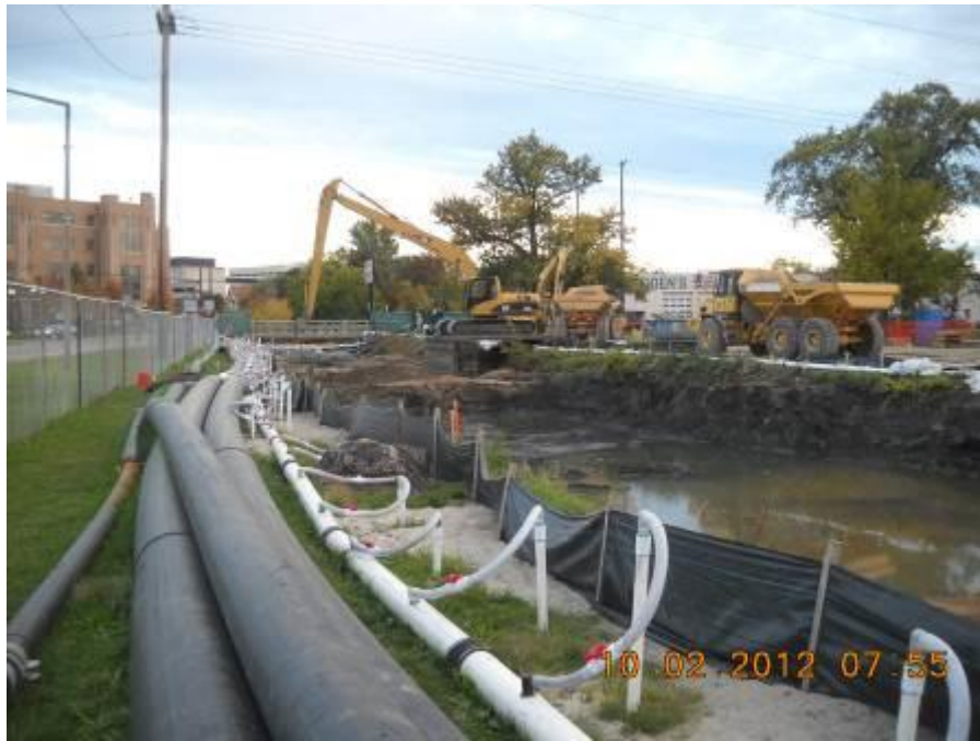
Site: Portage Creek Area Site – SA5-C Photograph No.: 17 Direction: North Subject: Excavation of contaminated sediments
