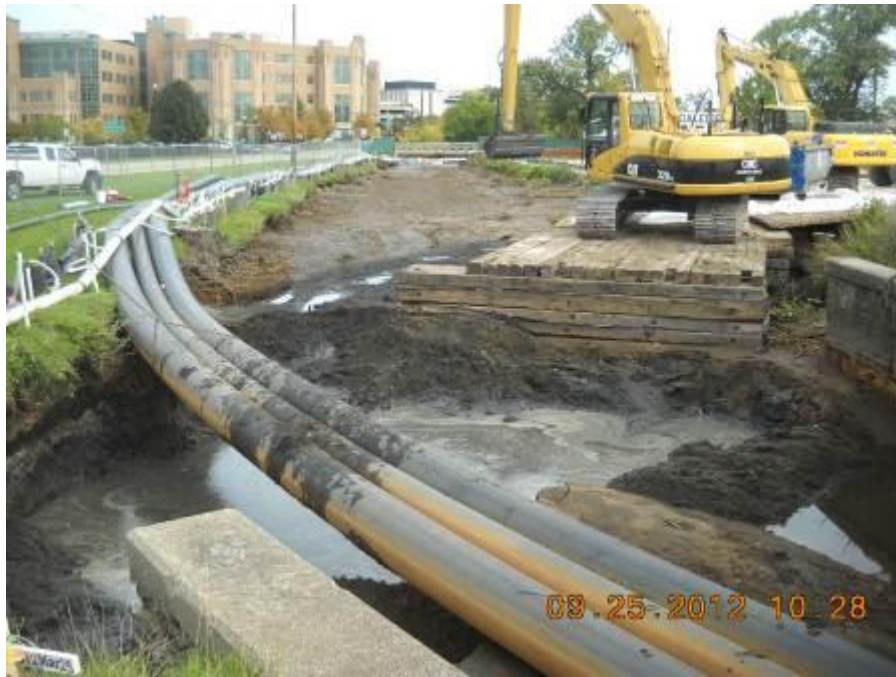
Site: Portage Creek Area Site – SA5-C Photograph No.: 13 Direction: North Subject: Excavation of contaminated sediment
