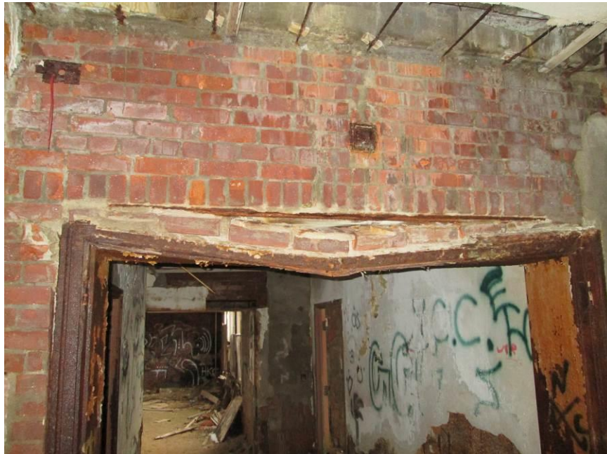
Photograph 23 – Brick Supported on Failing Steel Door Frame – East Wing – First Floor
