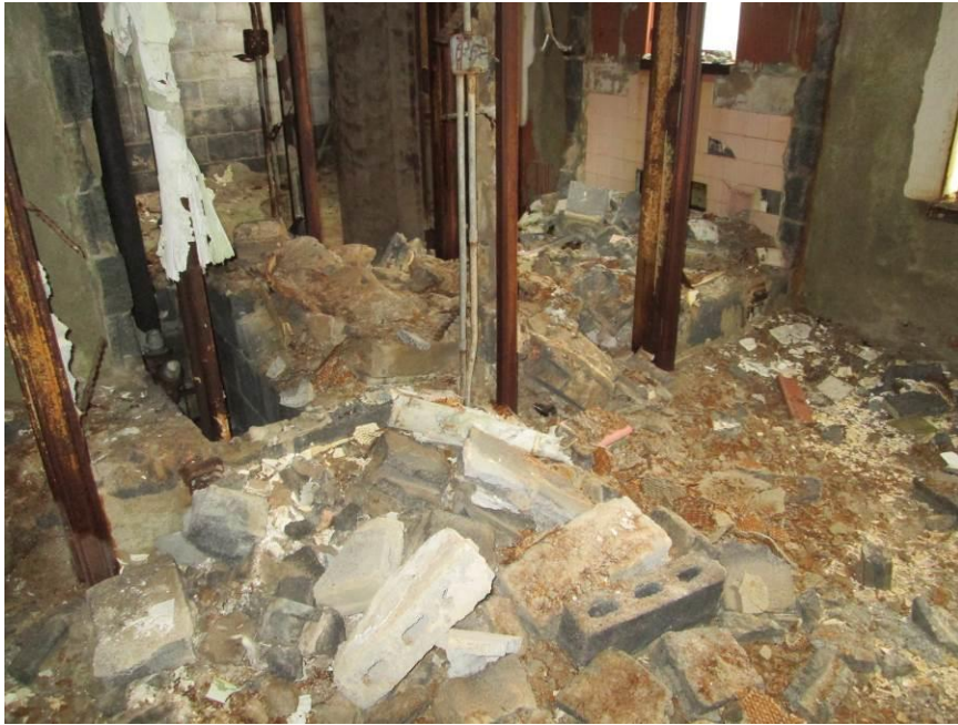
Photograph 8 – Demolition Debris on 1 st Floor in Main Hospital Patient Room
