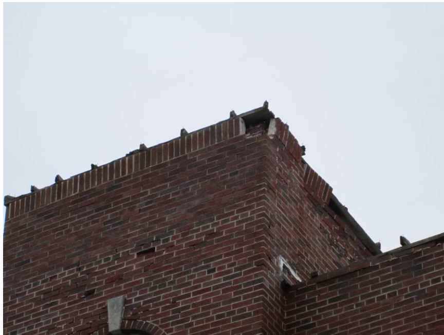
Photograph 33 – Crumbling Brick at Parapet of West Wing Main Hospital
