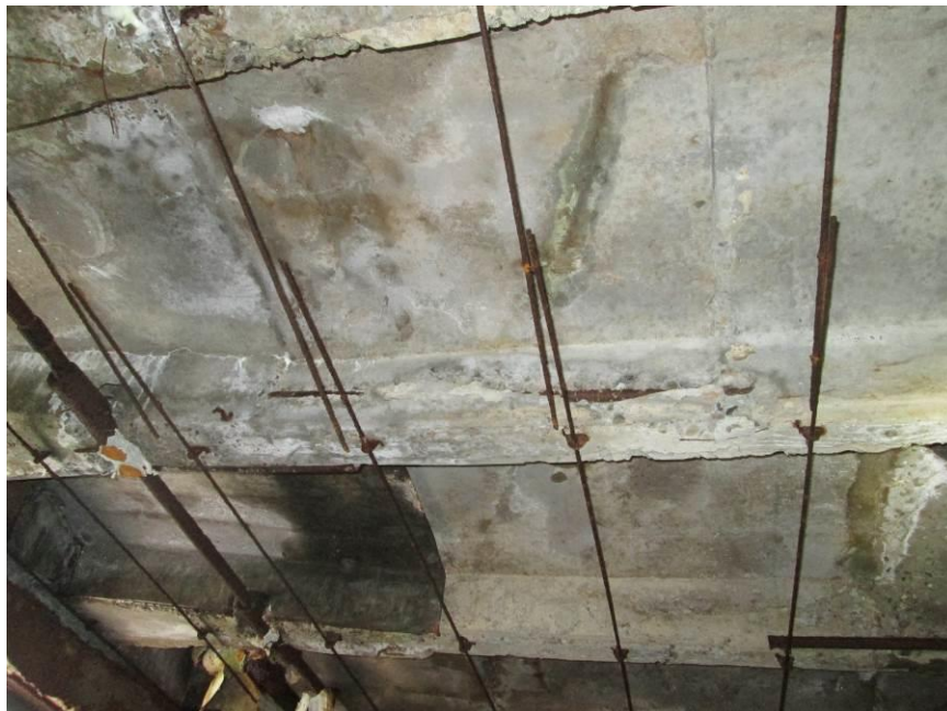
Photograph 27 – Damaged Concrete Joist Framing – East Wing – Second Floor
