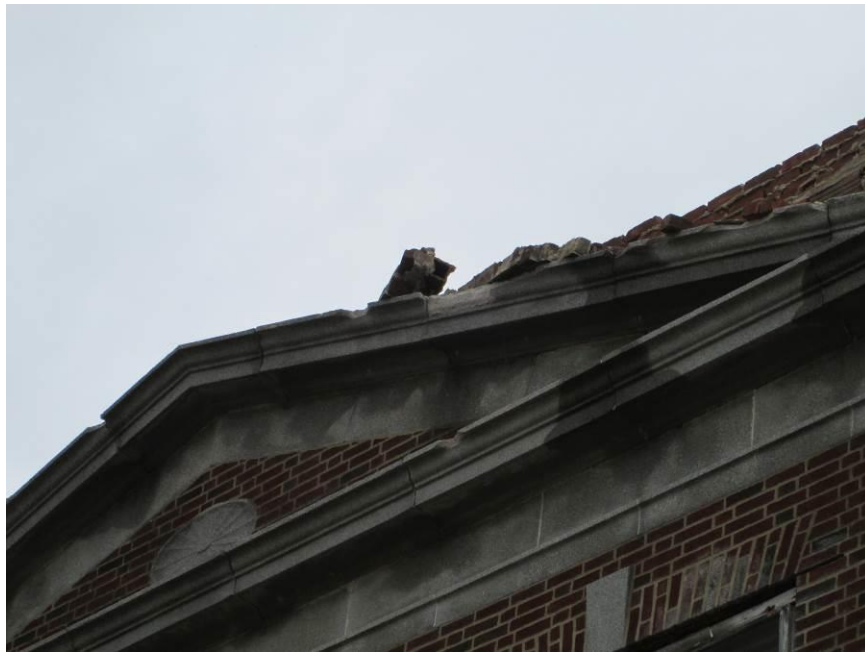
Photograph 37 – Brick Fall Hazard at Children's Wing Entry
