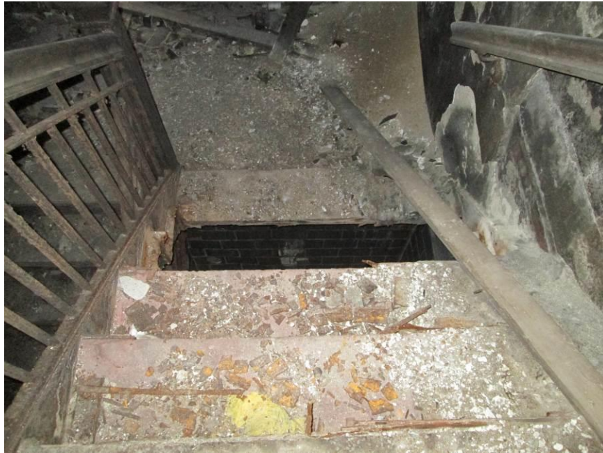
Photograph 15 – Failed Stair Treads and Risers at Back-Stage Stair
