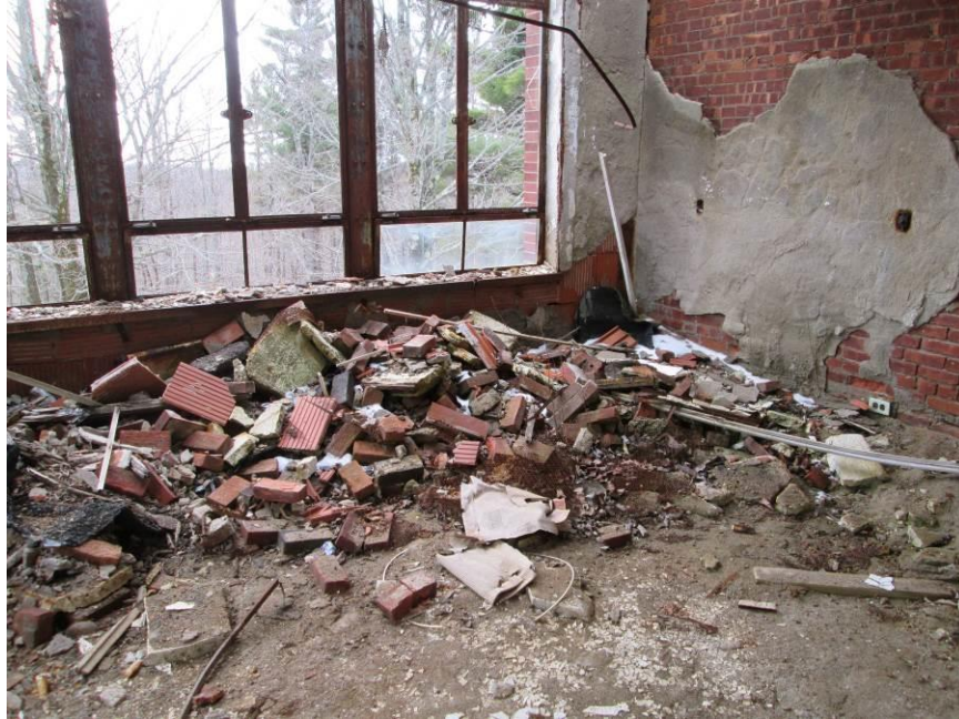
Photograph 26 – Debris Below Roof Framing Collapse and Above Deteriorated Joist Framing
