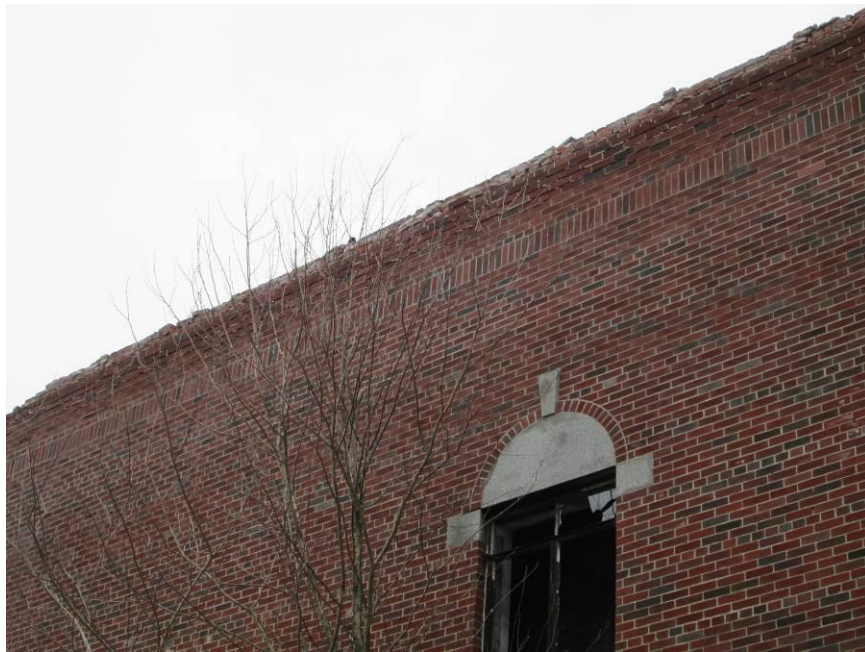
Photograph 35 – Crumbling Brick at Leaning Parapet of West Wing Main Hospital
