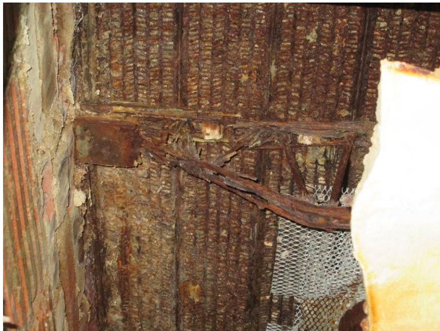
Photograph 29 – Failed Roof Joists in Eastern Children's Wing
