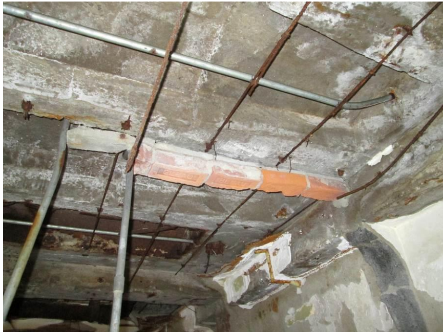
Photograph 5 – Loose Ceiling Material in West Wing, Typical Most Locations
