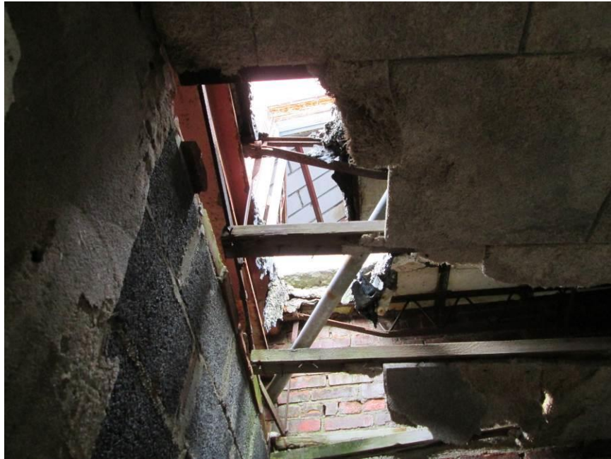
Photograph 4 – Hanging Ceiling Tiles Surrounding Collapsed Roof Decking (Main Hospital Adjacent to Center Core)
