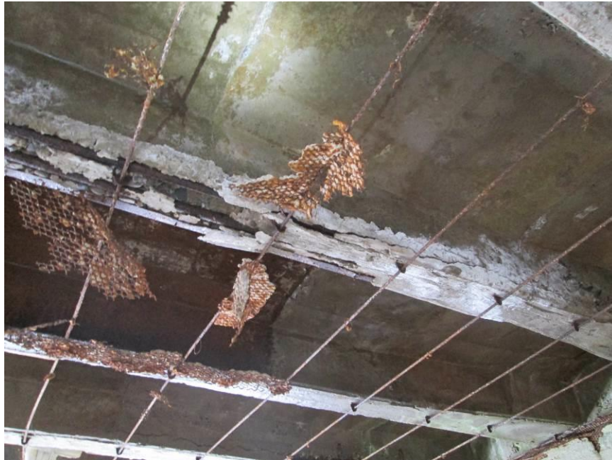
Photograph 24 – Unsafe Concrete Joist Framing – Second Floor
