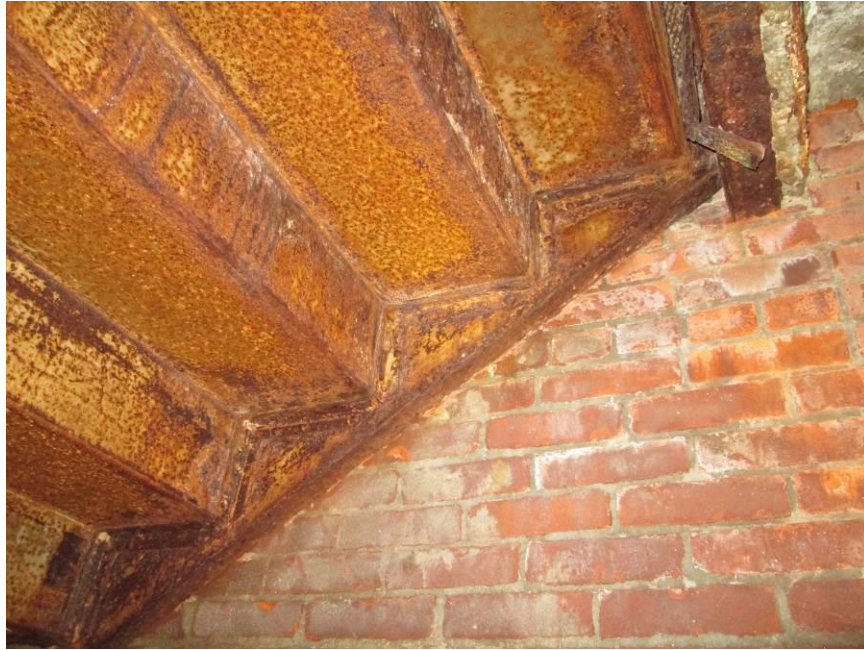
Photograph 20 – Deteriorated Stair Framing – East Wing – First Floor
