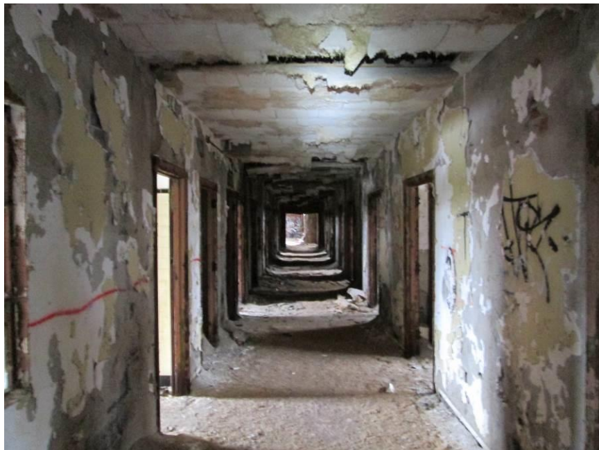
Photograph 3 – Deteriorated Ceiling Construction along Main Hospital Corridor
