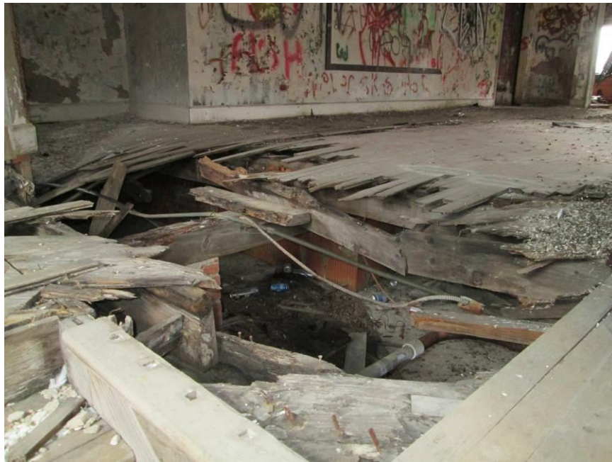
Photograph 17 – Failed Wood Stage Platform Framing
