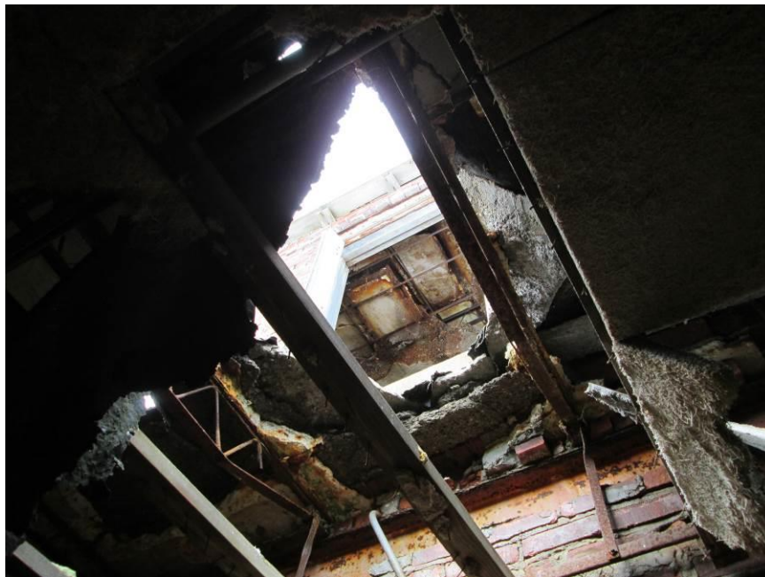
Photograph 21 – Hole in Roof Framing by East Wing Stair
