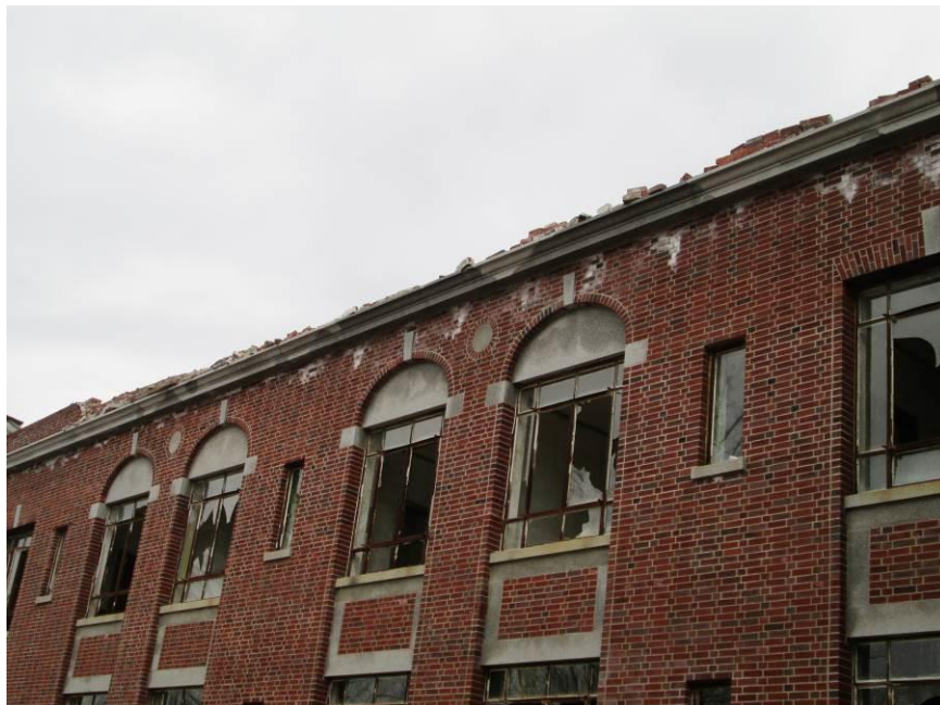
Photograph 40 - Brick Fall Hazard at Main Hospital South Face
