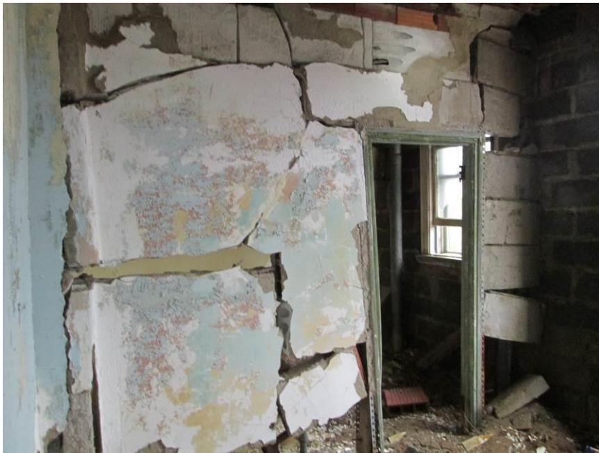
Photograph 6 – Partially Demolished Interior Masonry Partition
