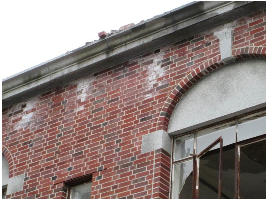
Photograph 38 – Brick Fall Hazard at Main Hospital South Face
