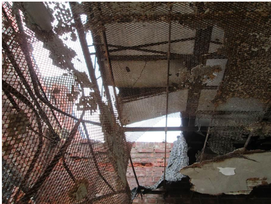
Photograph 25 – Hole in Roof Framing
