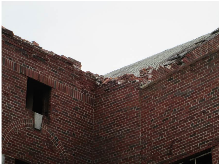
Photograph 34 – Crumbling Brick at Parapet of West Wing Main Hospital
