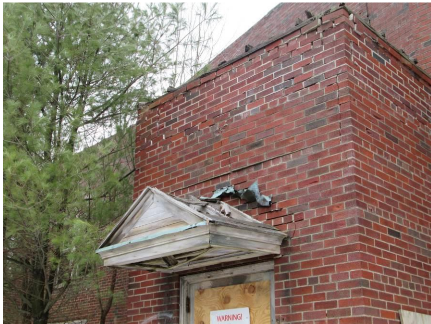
Photograph 36 – Deteriorated Brick and Compromised Awning near Children's Wing Rear Entry
