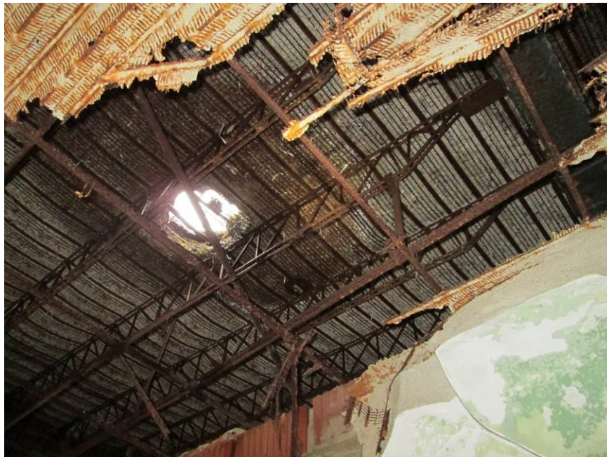
Photograph 28 – Hole in Roof – Children's Wing
