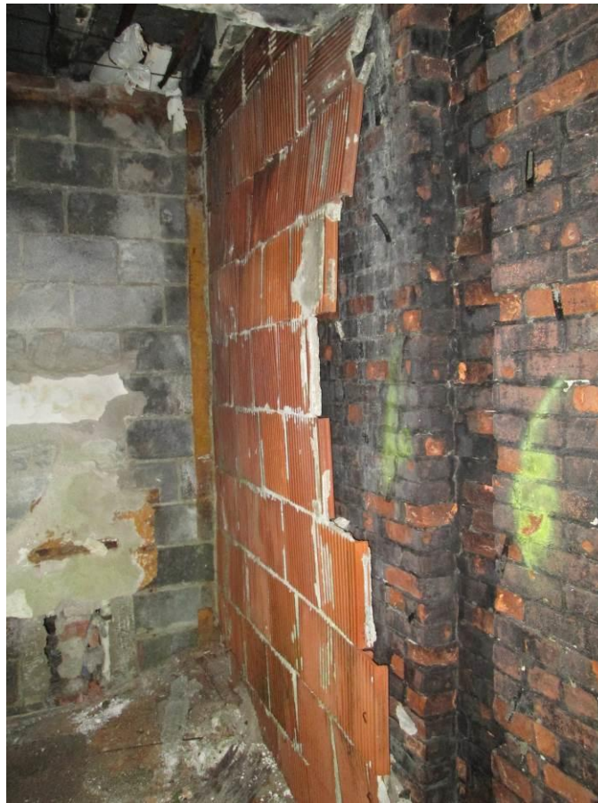
Photograph 9 – Unstable Interior Clay Masonry Finish in Main Hospital Patient Rooms
