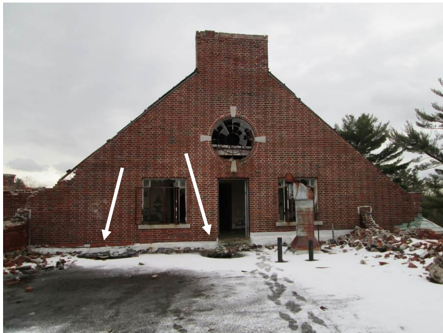
Photograph 11 – Holes in Roof of West Wing Framing Adjacent to Central Roof Top Structure
