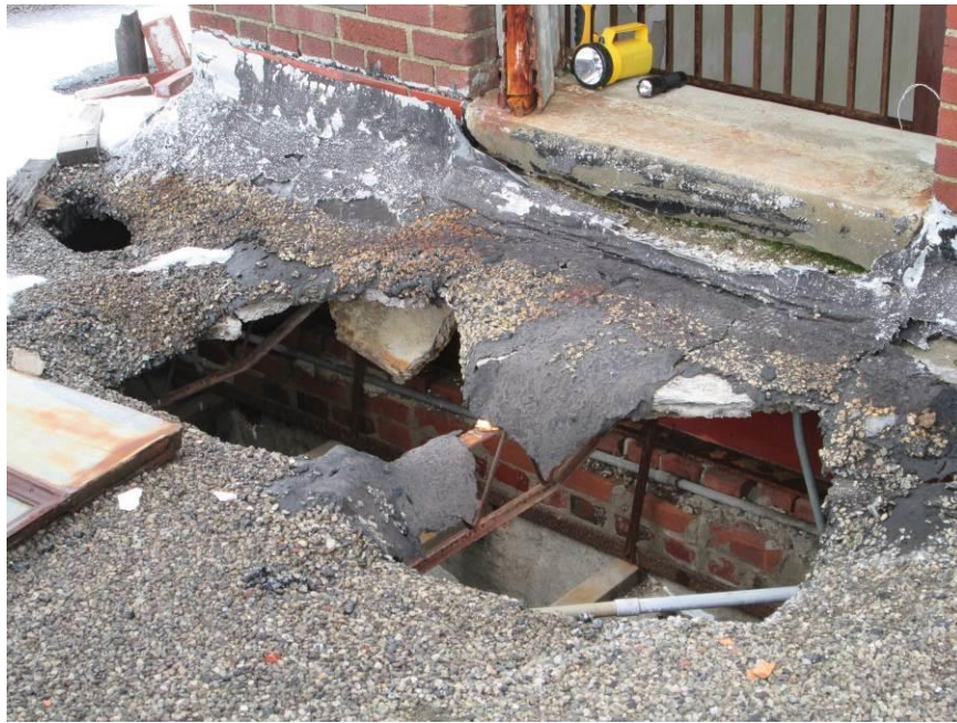
Photograph 10 – Hole in Roof Framing by West Wing Stair
