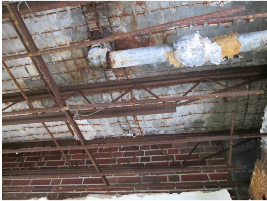
Photograph 30 – Rusting Roof Framing at Roof Drain and Ponding Location
