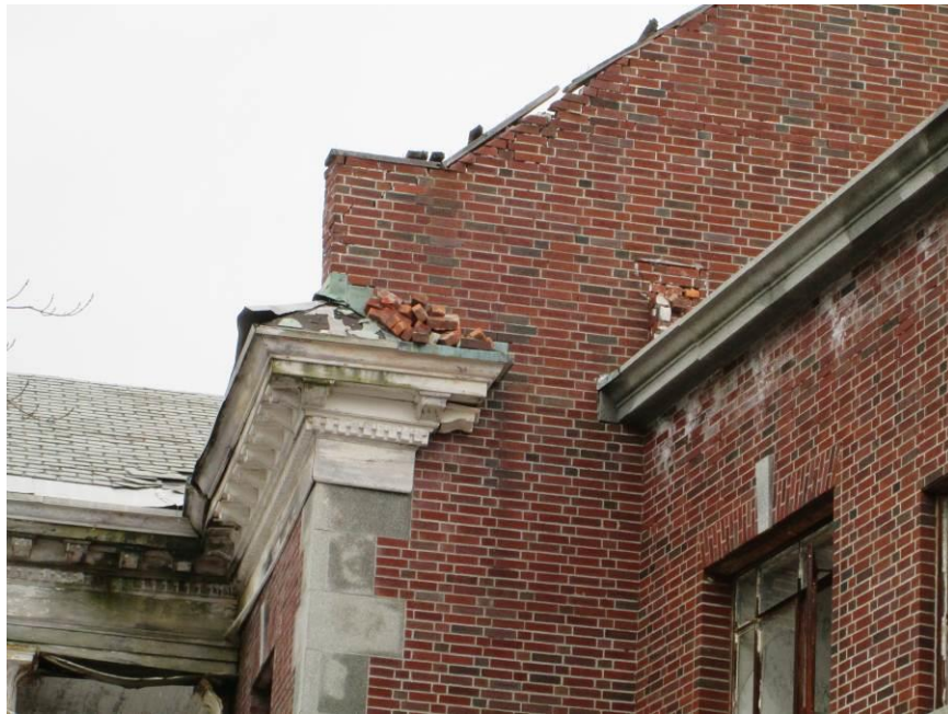
Photograph 39 - Brick Fall Hazard at Main Hospital South Face
