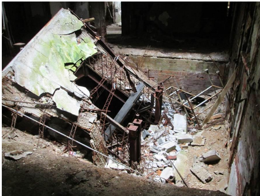
Photograph 14 – Debris on Second Floor of Central Grand Staircase
