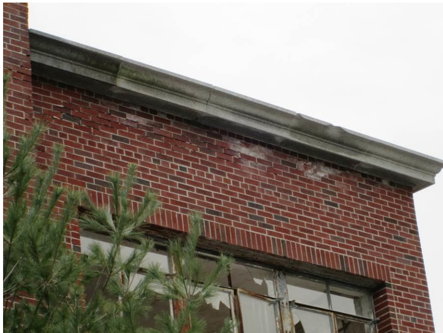
Photograph 32 – Displaced Cornice at West Wing Main Hospital
