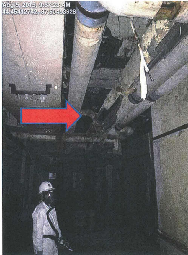
Photo 5: Damaged pipe wrap/friable asbestos
