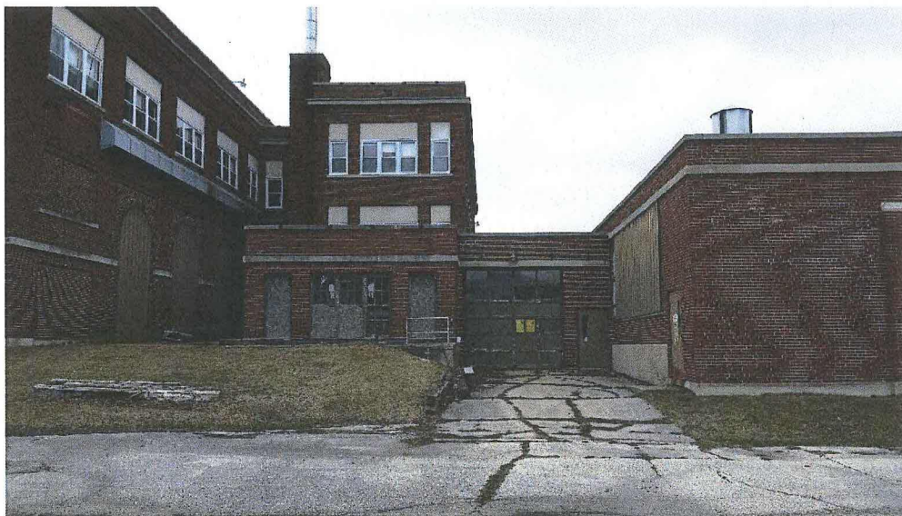
Photo 12: Measures to secure the building (warning signs and boarded up windows)
