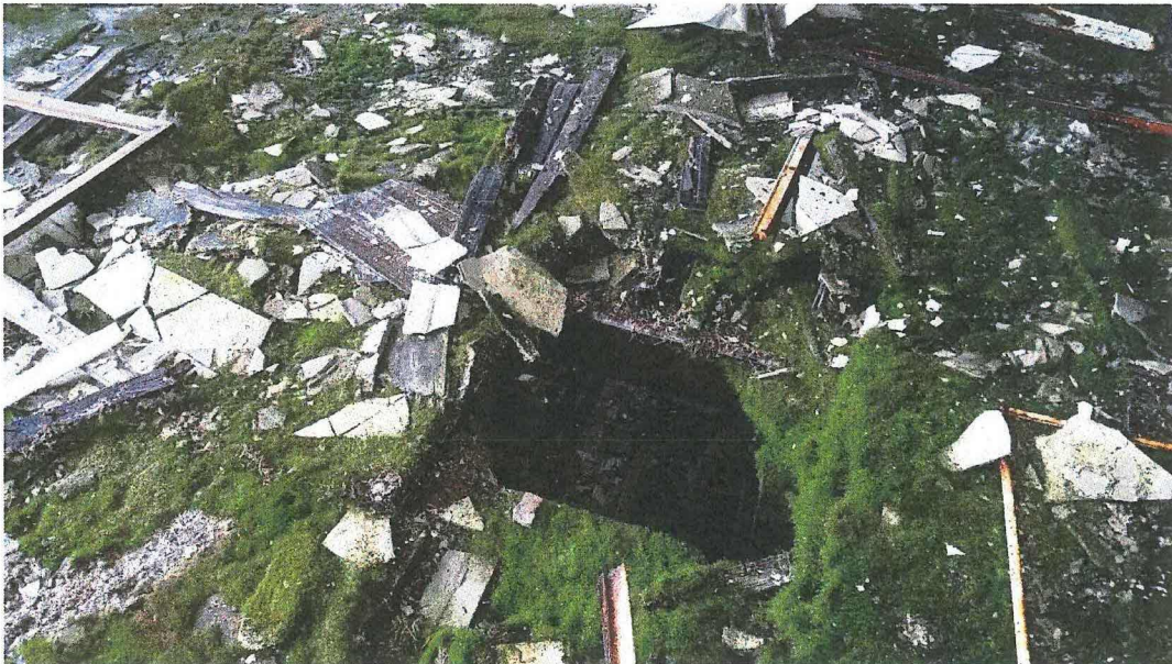
Photo 2: Water damage, including hole in floor and moss
