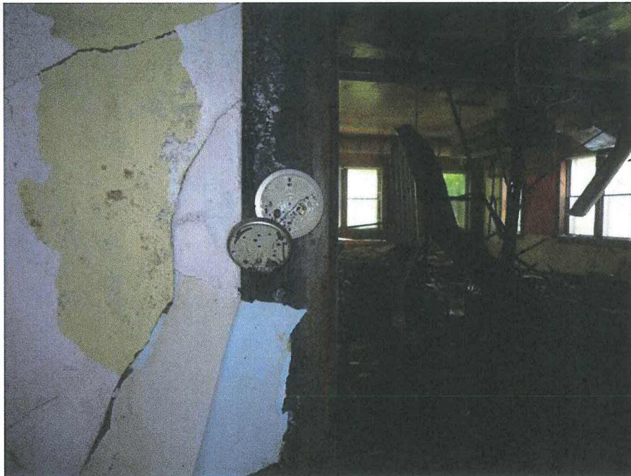
Photo 10: Broken thermostat
