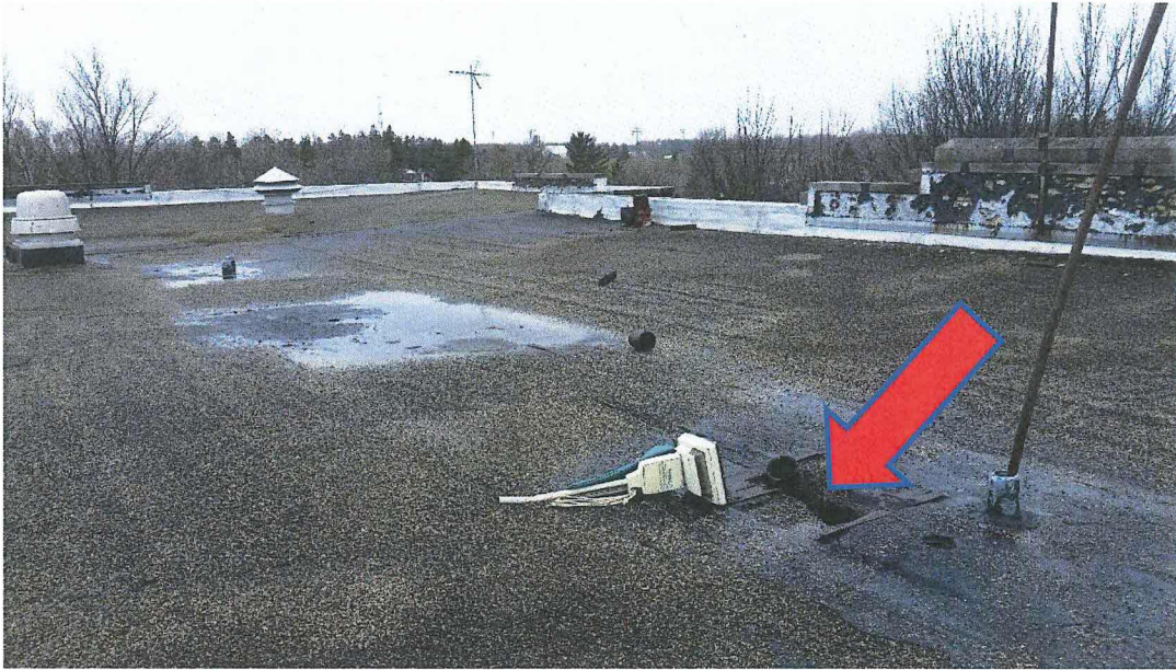
Photo 1: Hole in roof
