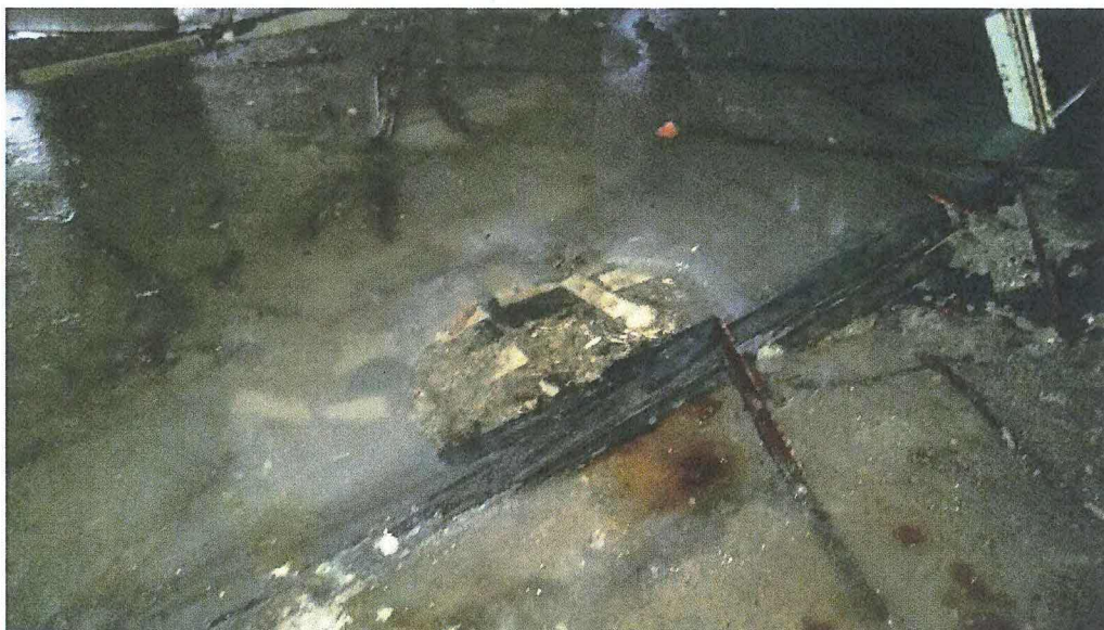
Photo 3: frozen pooled water on buckled floor
