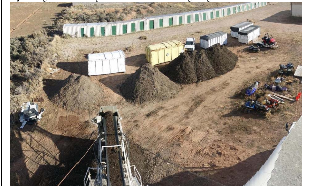
Photo Number: 36-20141212_144539.jpg Date: 12/12/14 Direction: East Photographer: Way Subject: Treated waste stock piled for final disposal
