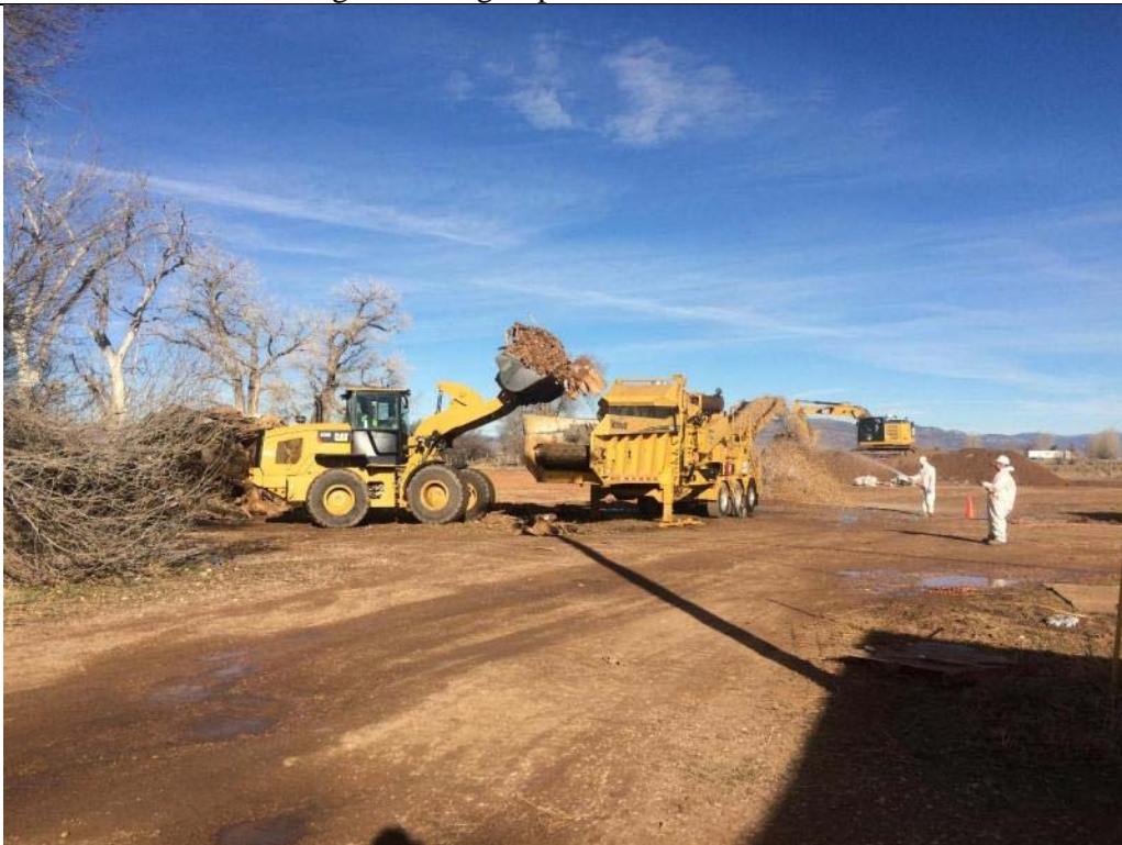
Photo Number: IMG_1483.JPG Date: 12/16/14 Direction: North Photographer: Merritt Subject: Size and volume reduction of non-hazardous debris prior to disposal
