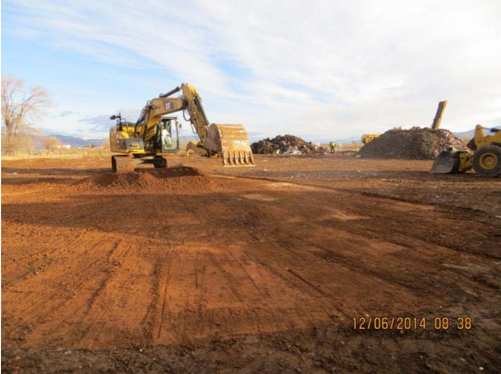
Photo Number: IMG_E02.JPG Date: 12/6/14 Direction: North Photographer: Bryniarski Subject: ERRS contractor removes impacted soil in waste stock pile footprint
