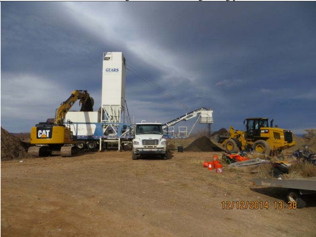
Photo Number: IMG_I05.JPG Date: 12/12/14 Direction: North Photographer: Bryniarski Subject: ERRS contractor loads waste into pug mill for second waste treatment process
