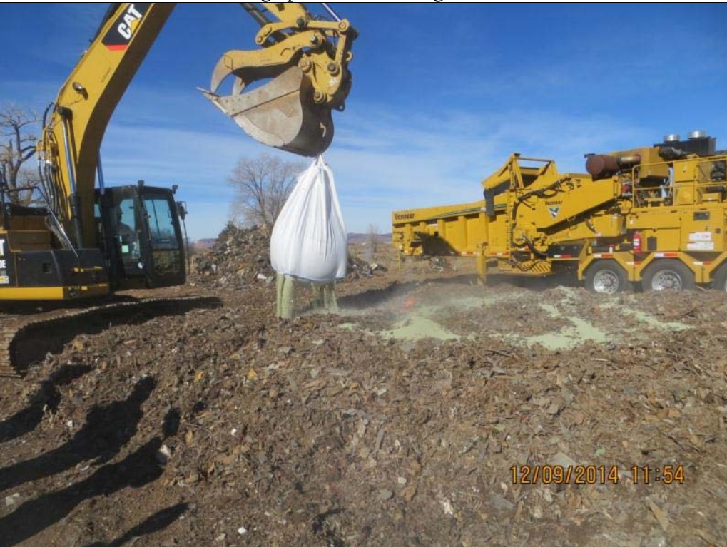
Photo Number: IMG_F04.JPG Date: 12/9/14 Direction: Northwest Photographer: Bryniarski Subject: ERRS contractor treats waste with fertilizer prior to second grinding process
