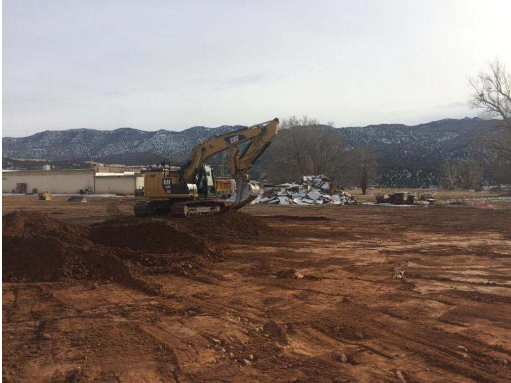
Photo Number: IMG_1463.JPG Date: 12/15/14 Direction: South Photographer: Merritt Subject: ERRS contractor excavating impacted soil in former waste staging footprint
