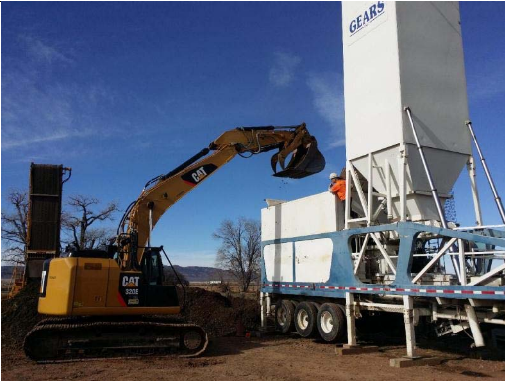
Photo Number: 19-20141210_122103.jpg Date: 12/10/14 Direction: West Photographer: Way Subject: ERRS contractor loading pug mill with ground waste
