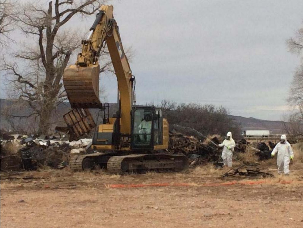
Photo Number: IMG_1335.JPG Date: 12/2/14 Direction: North Photographer: Merritt Subject: ERRS contractor sorts electronic waste and sprays water to suppress airborne dust
