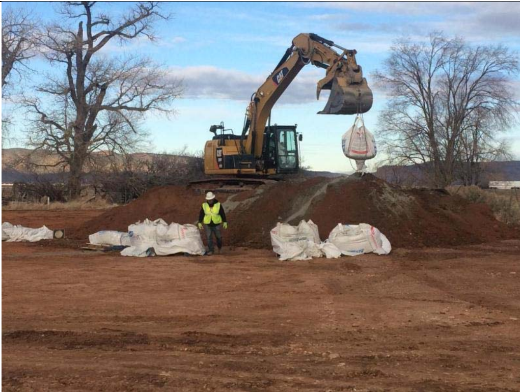
Photo Number: IMG_1475.JPG Date: 12/16/14 Direction: Northwest Photographer: Merritt Subject: ERRS contractor treating remaining impacted soil with Portland cement
