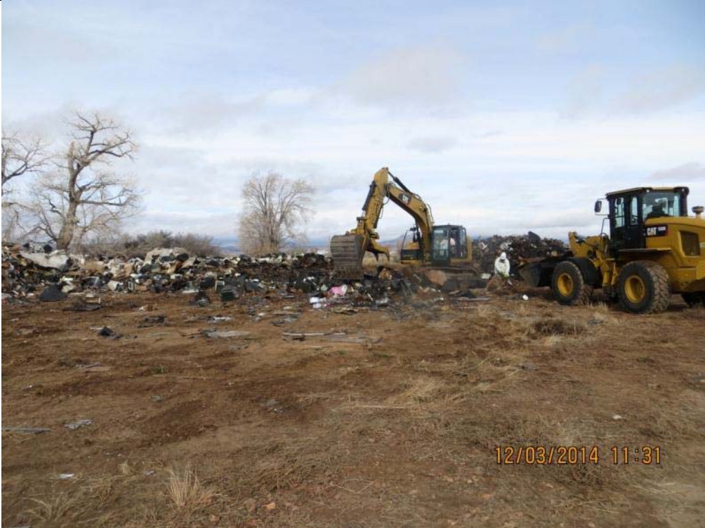
Photo Number: IMG_B13.JPG Date: 12/3/14 Direction: North Photographer: Bryniarski Subject: ERRS contractor sorts electronic waste prior to grinding and treatment
