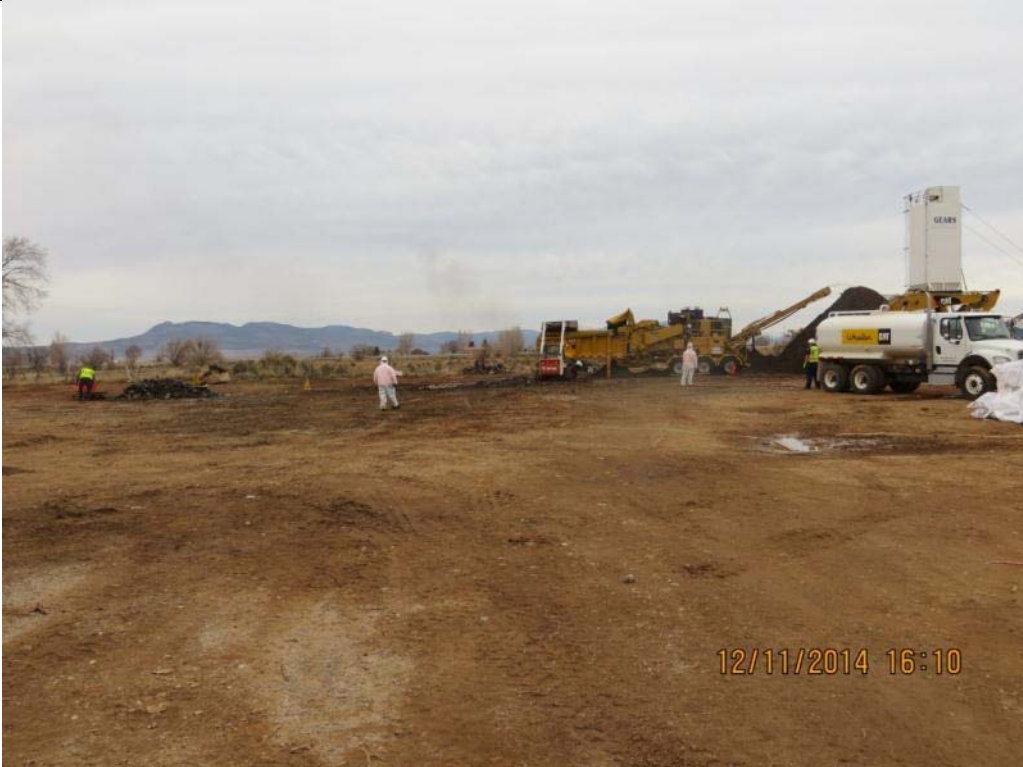
Photo Number: IMG_H04.JPG Date: 12/11/14 Direction: North Photographer: Bryniarski Subject: ERRS contractor loads remaining waste for second grinding process
