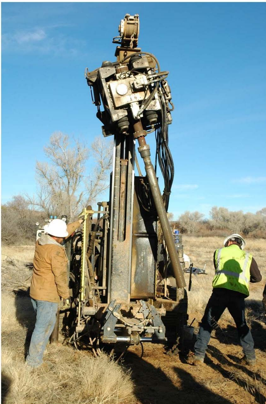
Photo DSC_0643: Photos during investigation: depicting percussion drill rig used to obtain cores from the ground in the Iron King Mine Blow Out Path
