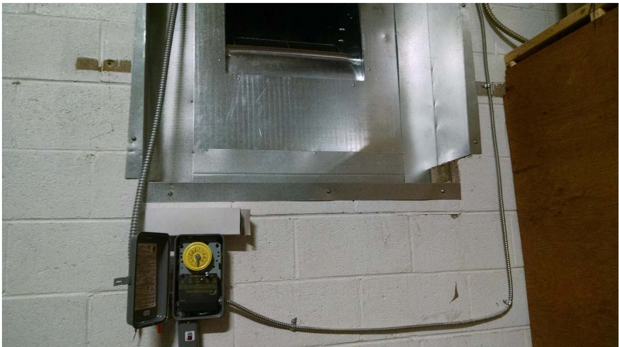
Photo #2: Thermostat control (lower left) for the positive pressure ventilation fan.
