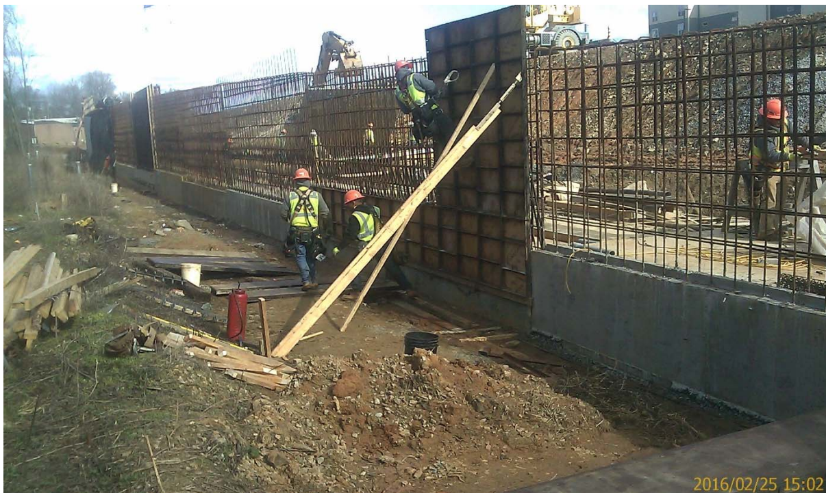
Photo #8: Retaining wall construction to south of Leather Trimmings building. Note the lack of exposed groundwater at this work location.
