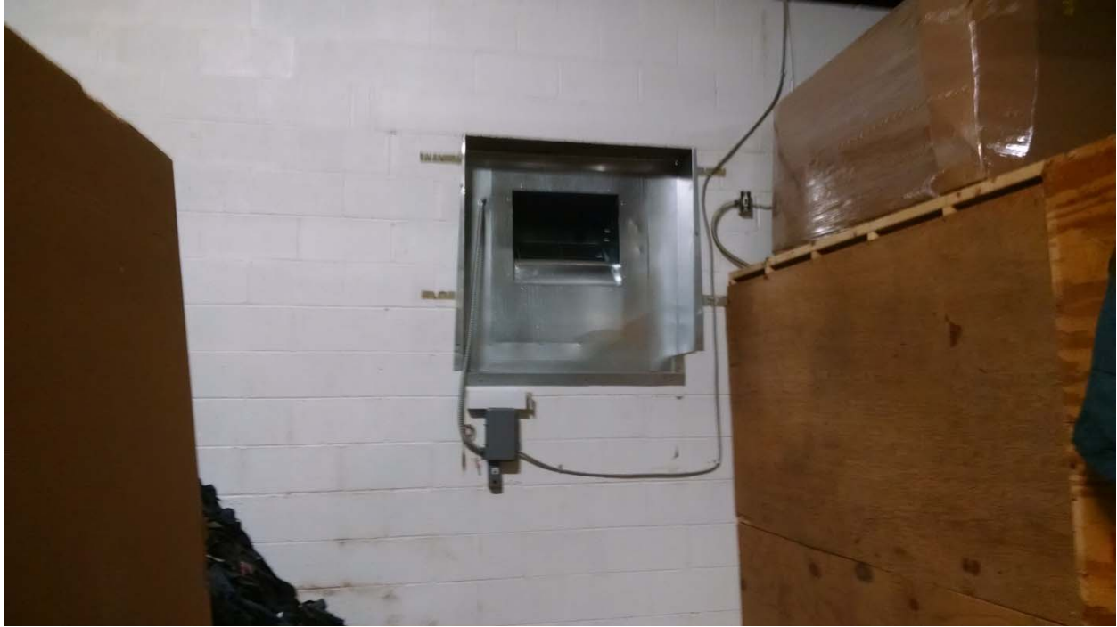
Photo #1: Positive pressure ventilation fan installed within the south wall of the Leather Trimmings facility.
