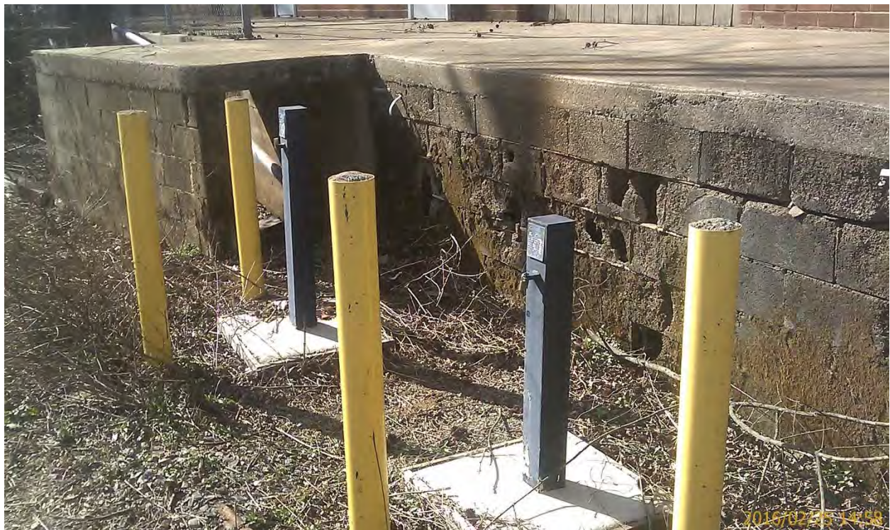
Photo #8: Closer view of PMW-20A & 20B and deteriorated cinder blocks that comprise the loading dock behind the Nexus Church.
