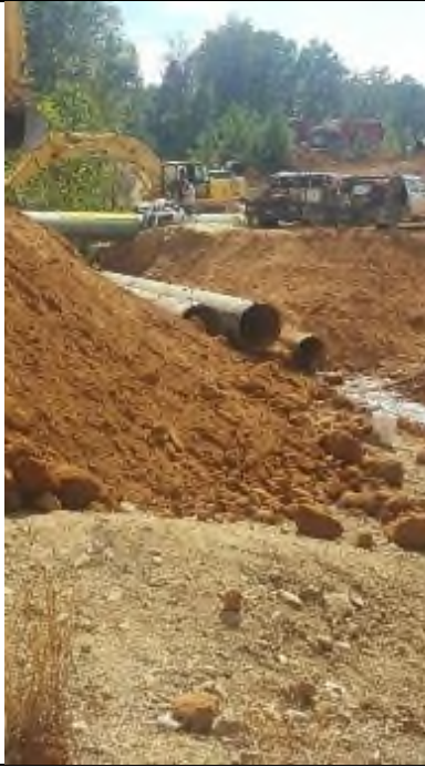
Installation of the two 40-inch culverts near Pond 1.
