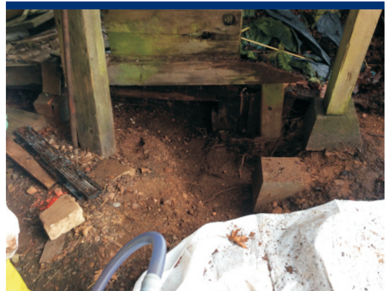
Photo 7 Excavated area in the carport, ranging from 3 to 21 inches in depth.
