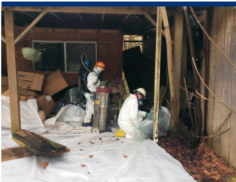
Photo 3 Excavating mercury-contaminated soil by hand in the carport.
