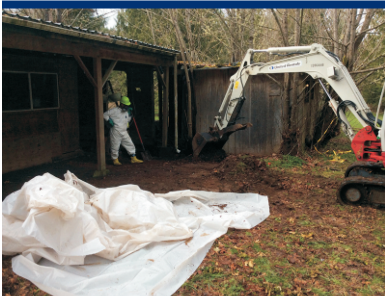
Photo 8 Excavating shallow soil and leaf litter outside the carport to a depth of 2 inches.
