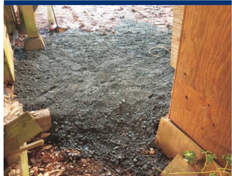
Photo 12 Backfilled excavated area near the carport with 3/4" minus gravel.
