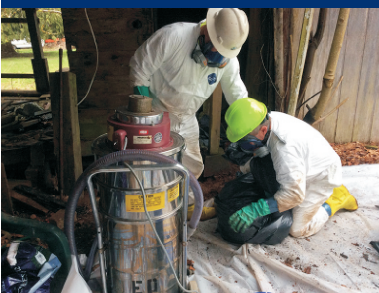
Photo 4 Excavating mercury-contaminated soil by hand in the carport.
