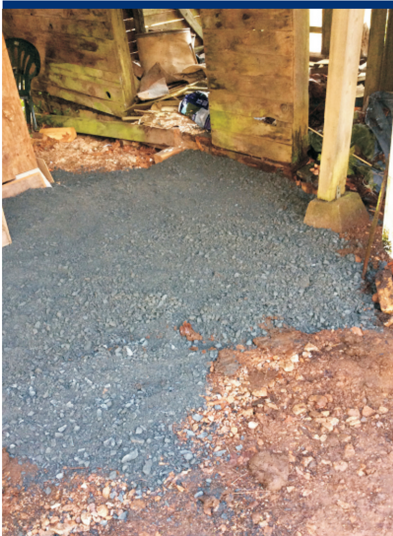
Photo 11 Backfilled excavated area in the carport with 3/4" minus gravel.
