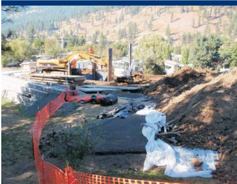
Photo 17 Excavation of drywell in background, with stockpile of asbestos-contaminated soil in foreground.
