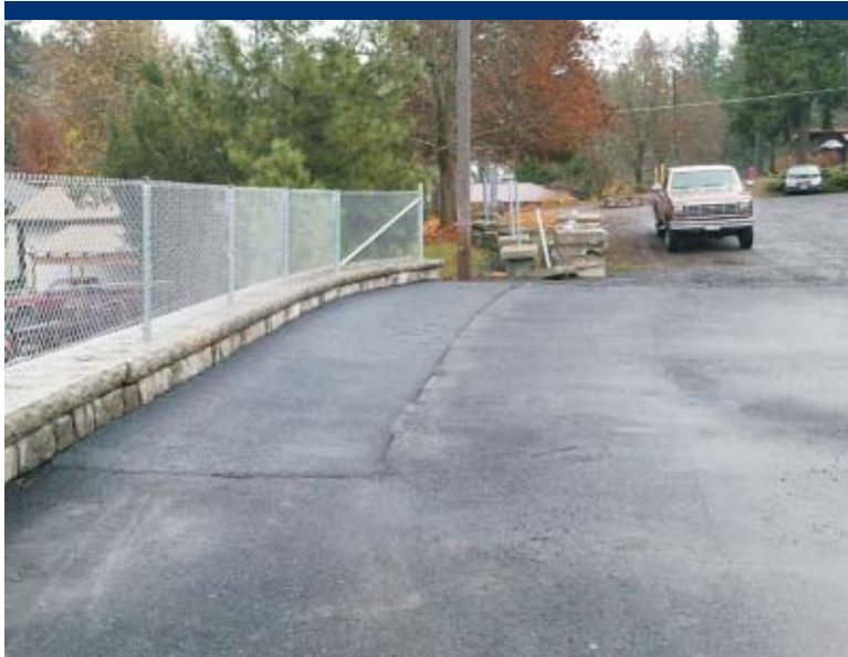
Photo 33 Completed retaining wall and chain-link fence with asphalt for parking area.
