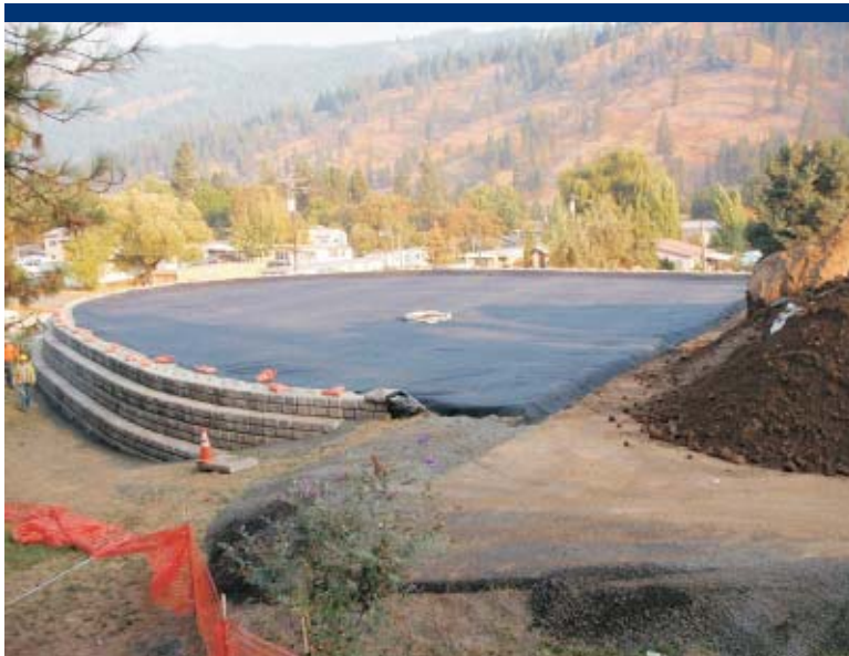
Photo 31 Final view of liner over asbestos-contaminated material before installation of asphalt and top soil.
