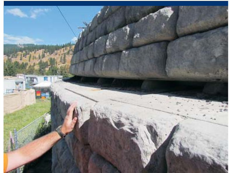
Photo 4 Close-up of retaining wall with shifted blocks before 2012 removal action.
