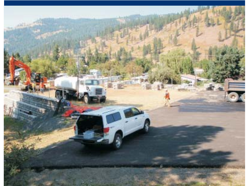
Photo 2 Heavy equipment is used to disassemble the wall by removing individual precast blocks.
