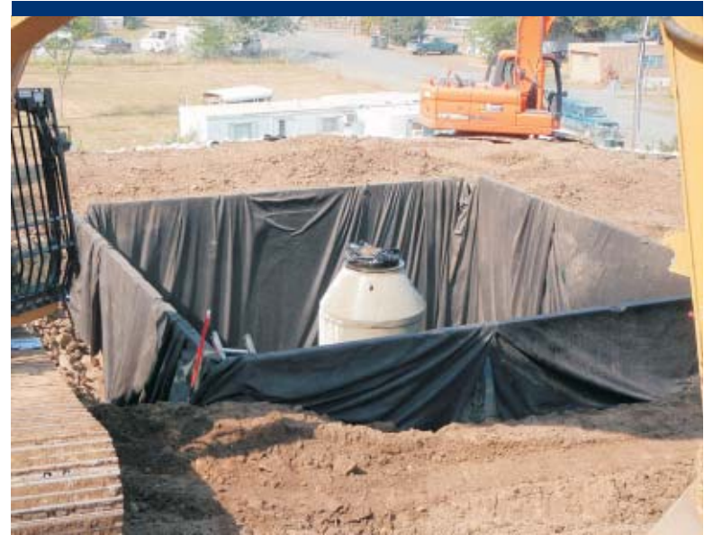
Photo 22 Installation of fabric liner around drain rock and dry well.
