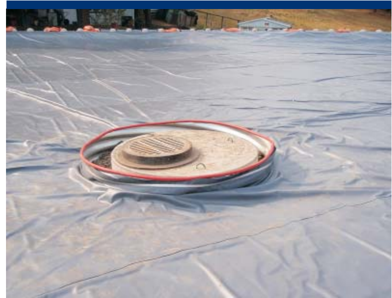
Photo 30 Liner material around surface of dry well.
