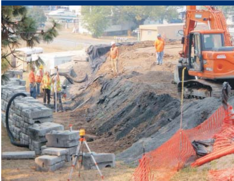
Photo 9 Measuring the base height for the southwest section of the wall.
