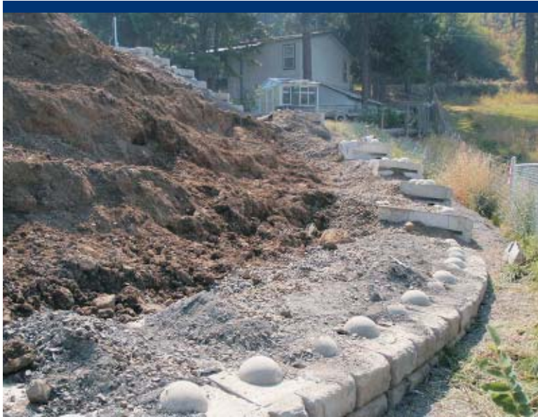
Photo 5 Dis-assembling of the west wall shifted blocks.
