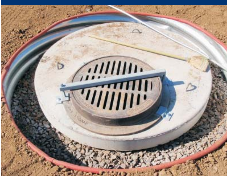
Photo 25 Dry well completed to the surface level.
