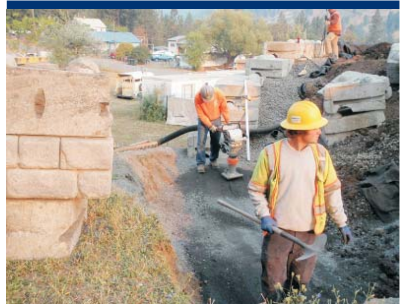
Photo 10 Compaction of base in preparation for the rebuilding of the southwest section of wall.
