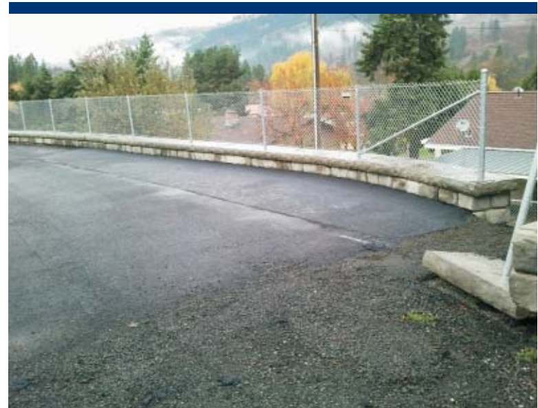
Photo 32 Completed retaining wall and chain-link fence with asphalt for parking area.
