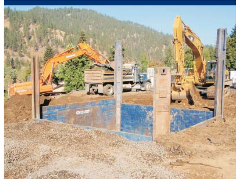
Photo 18 Close-up of dry will excavation and shoring.
