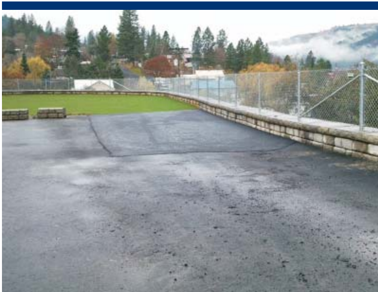
Photo 35 Completed asphalt parking area and grass dry retention basin.
