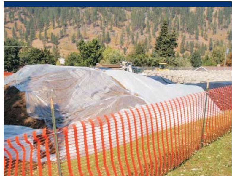
Photo 16 Asbestos-contaminated soil excavated from behind wall stockpile on-site with cover.
