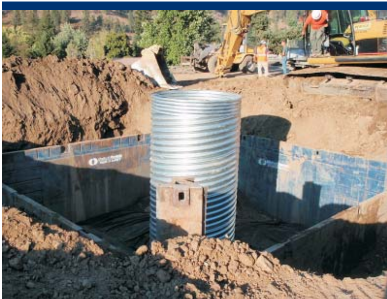
Photo 23 Installation of galvanized culvert around dry well for drain rock.
