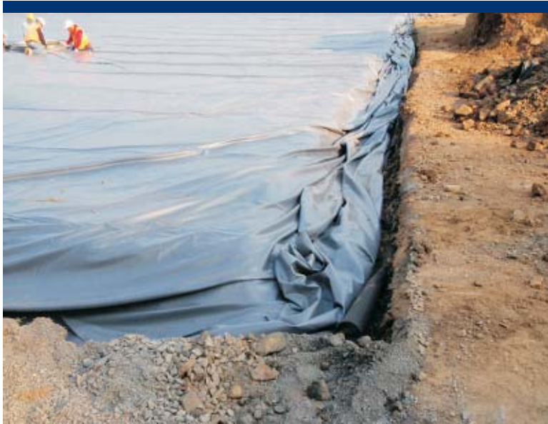
Photo 29 Installation of liner material at edge of soil retention basin and at the edge of the asphalt parking lot.
