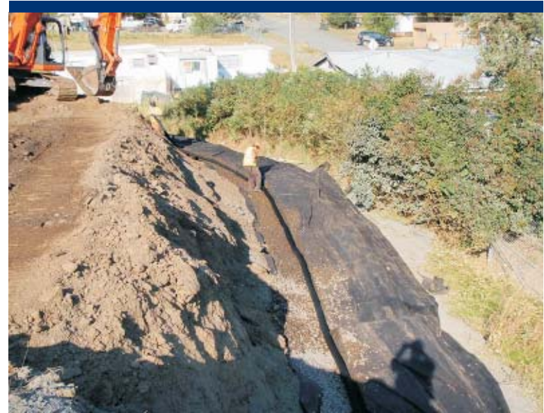
Photo 6 Base Blocks replaced with fabric liner.
