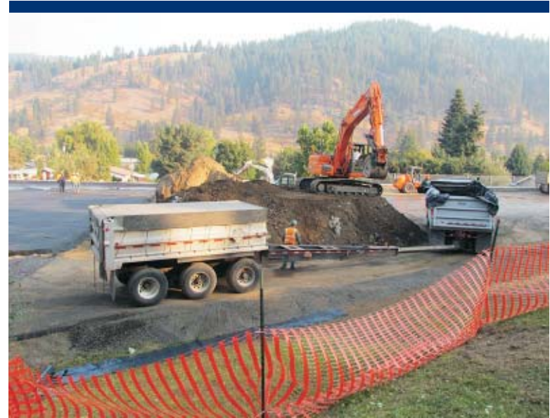
Photo 34 Loading of asbestos-contaminated soil into trucks for off-site disposal.
