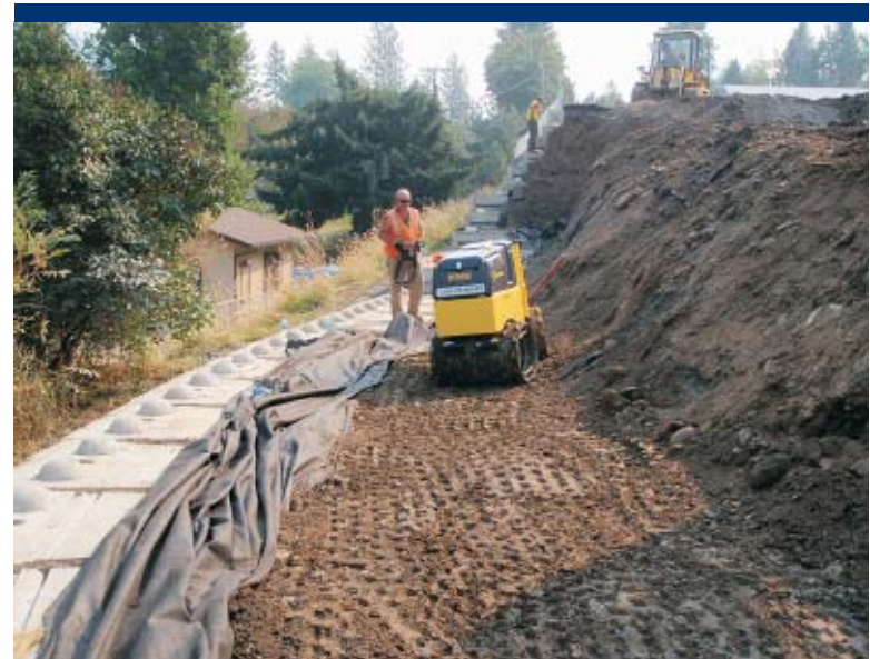
Photo 8 Compaction of asbestos-contaminated soil behind the wall.
