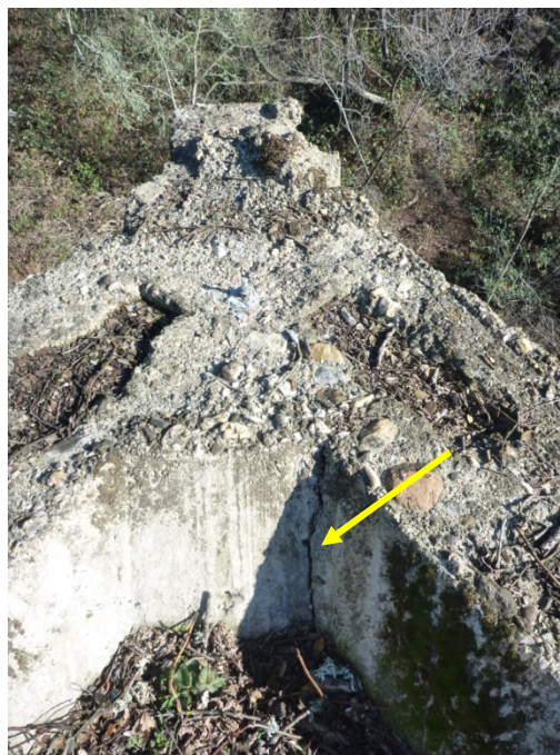
Figure 11 Crack between Arch and Buttress Shared by Arches 5 and 6
