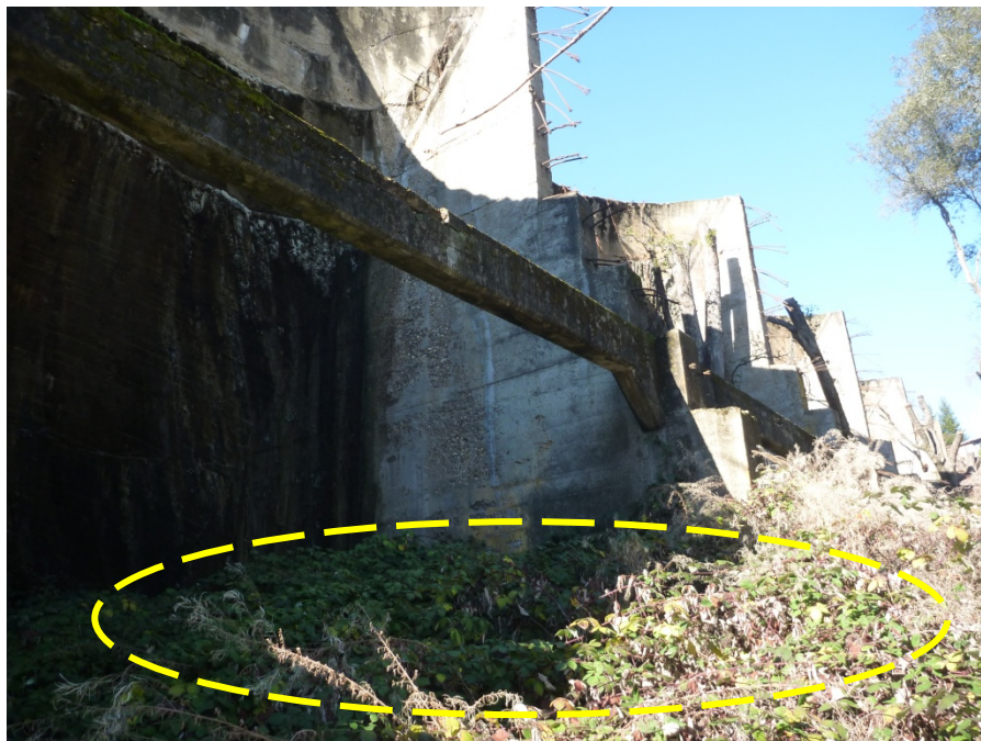
Figure 29 Vegetation overgrowth at Arch #7
