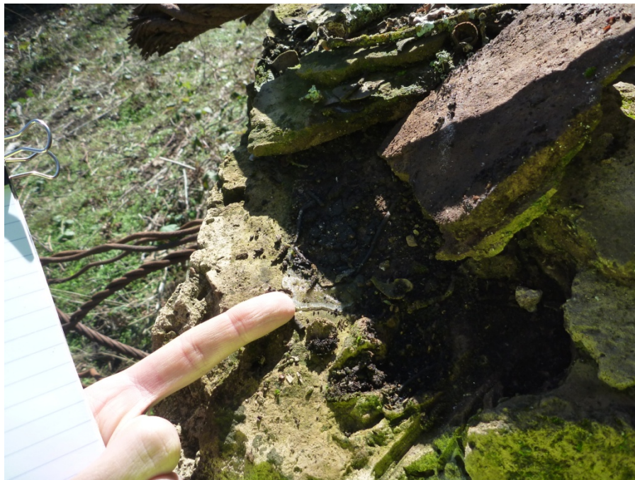
Figure 9 Right Buttress Wall of Arch #5 showing signs of Freeze Thaw Damage
