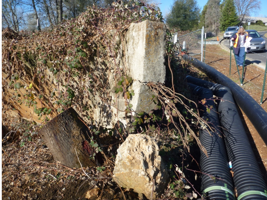
Figure 2 Condition of Right Buttress Wall of Arch #1
