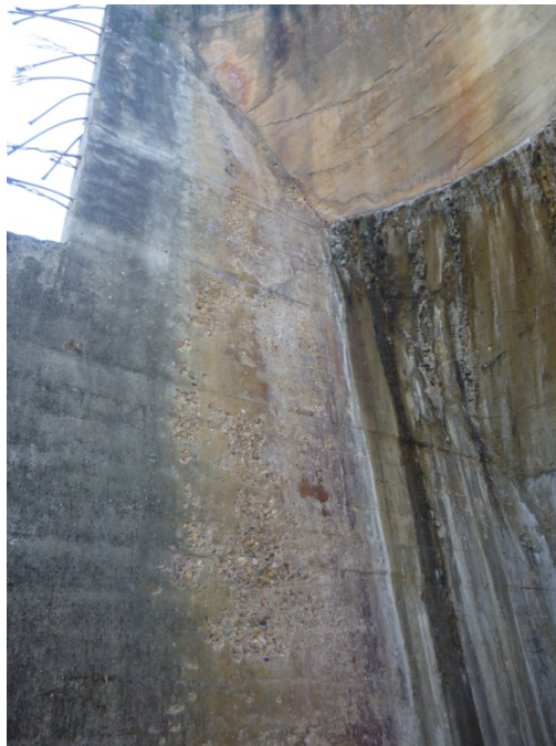
Figure 13 Possible Freeze Thaw Damage on Buttress Wall
