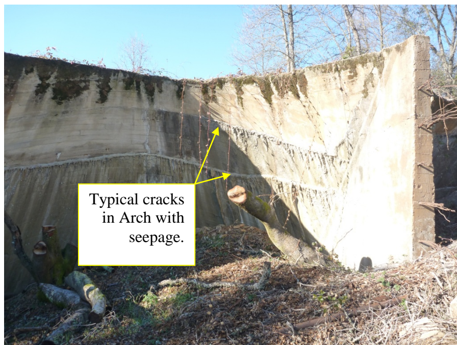
Figure 4 Condition of Arch #3
