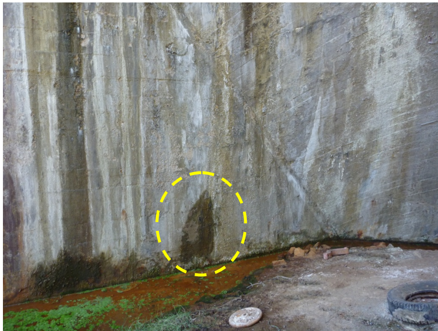
Figure 15 Seepage Coming through possible Diagonal Crack on Right Buttress Wall of Arch #6
