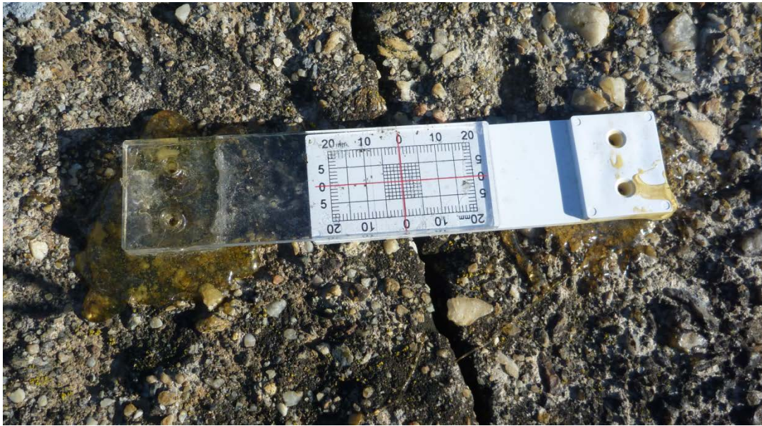
Figure 19 Crack between Arch and Buttress Shared by Arches 8 and 9
