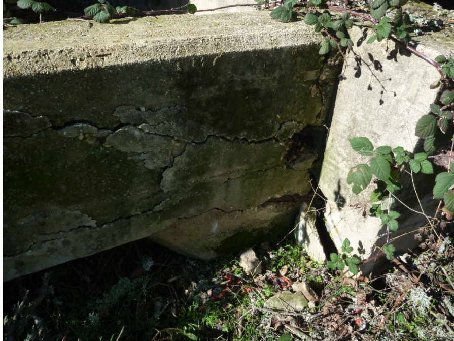
Figure 10 Failed Tie Beam extending between Buttresses of Arch #5
