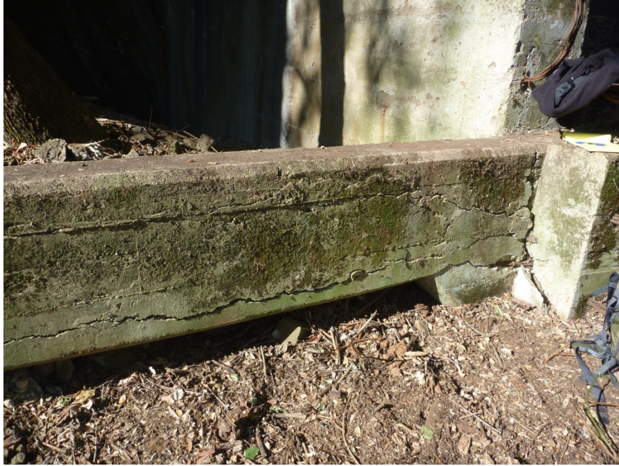
Figure 4 Existing Condition of Tie Beams (Exampple 2)
